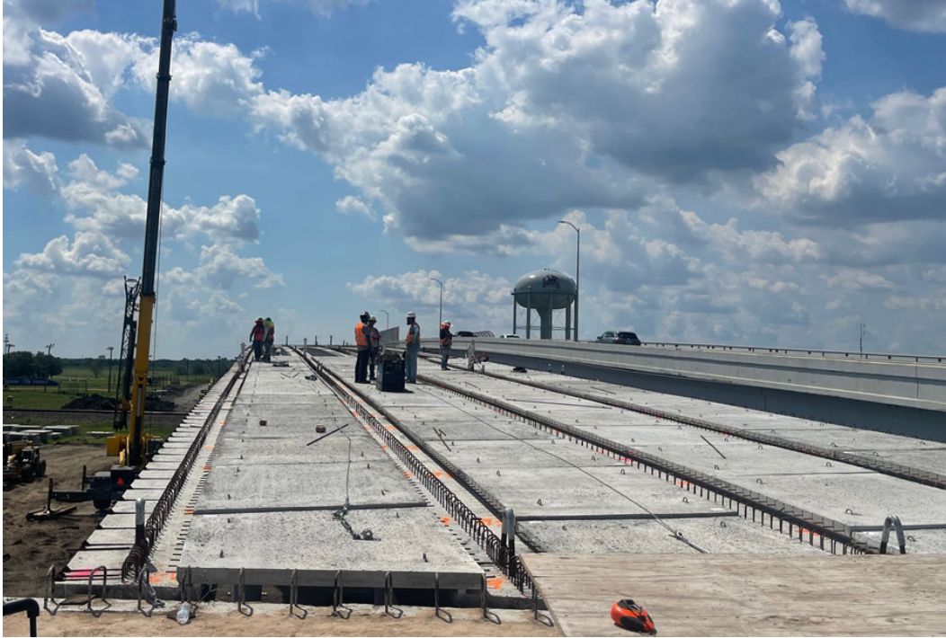
Precast Concrete Panel Installation
