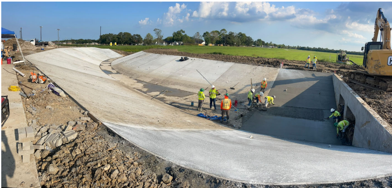
BDD4 Channel lining and Headwall
