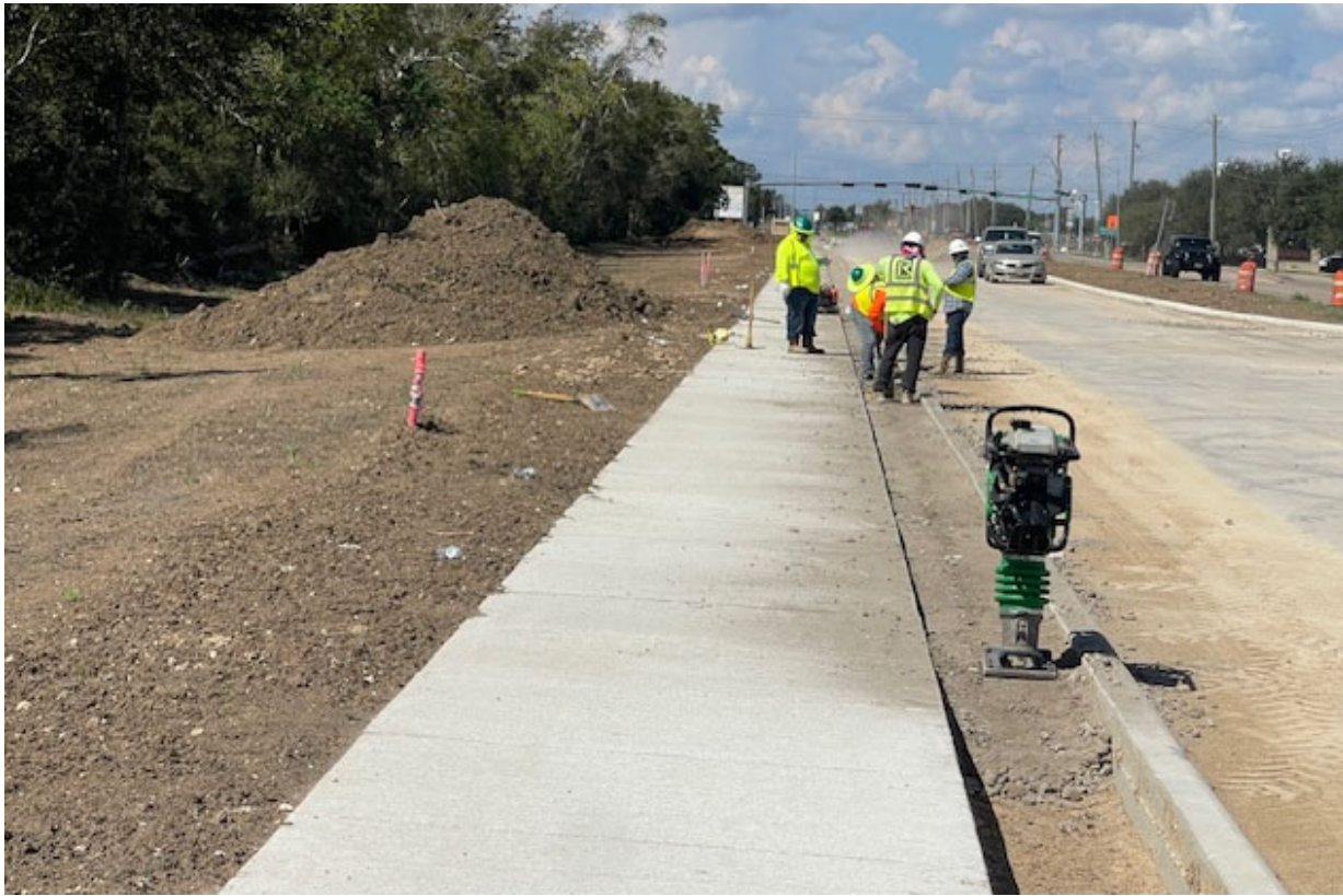
Installation of Cement Stabilized Base for Brick Pavers
