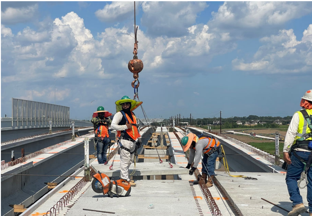
Precast Concrete Panel Installation
