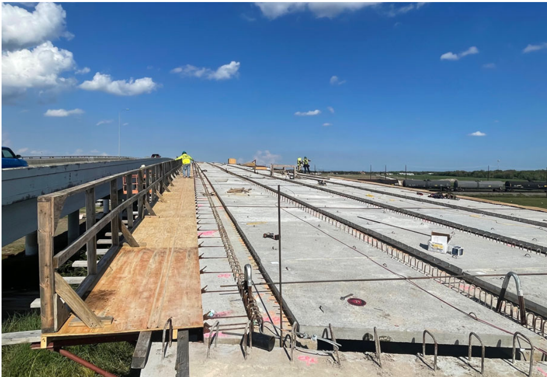
Overhang Installation
