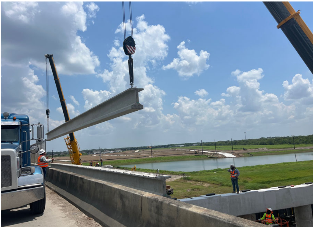
Beam Installation
