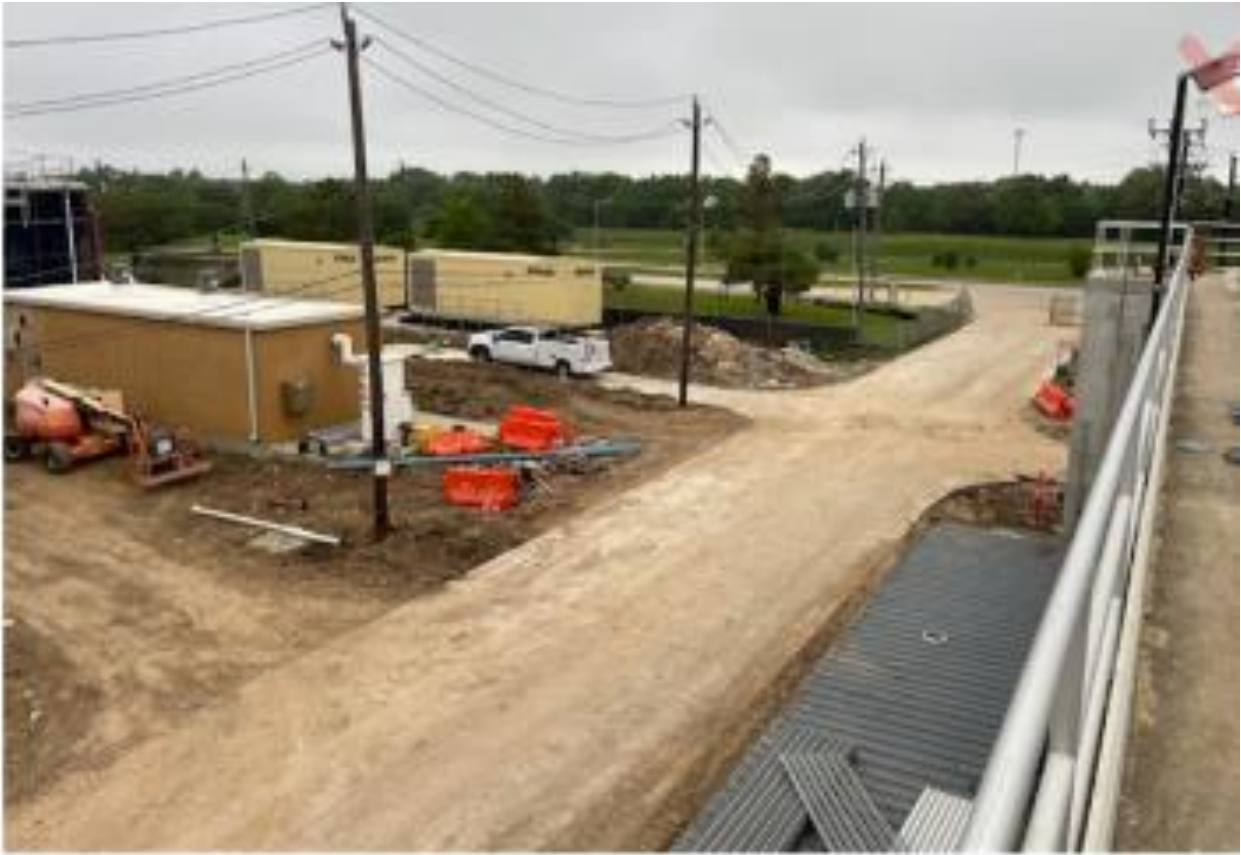
Site Works (paving)
