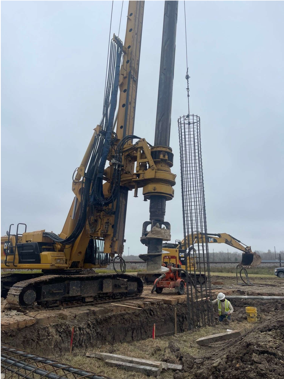
Roadway bridge drill shaft construction
