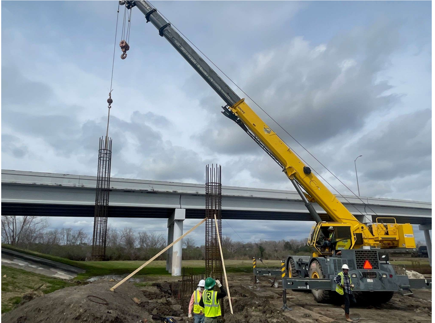
Roadway bridge drill shaft construction.
