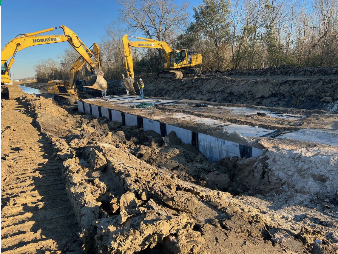
Installing new 8'x5' Reinforced Concrete Boxes for stormwater system
