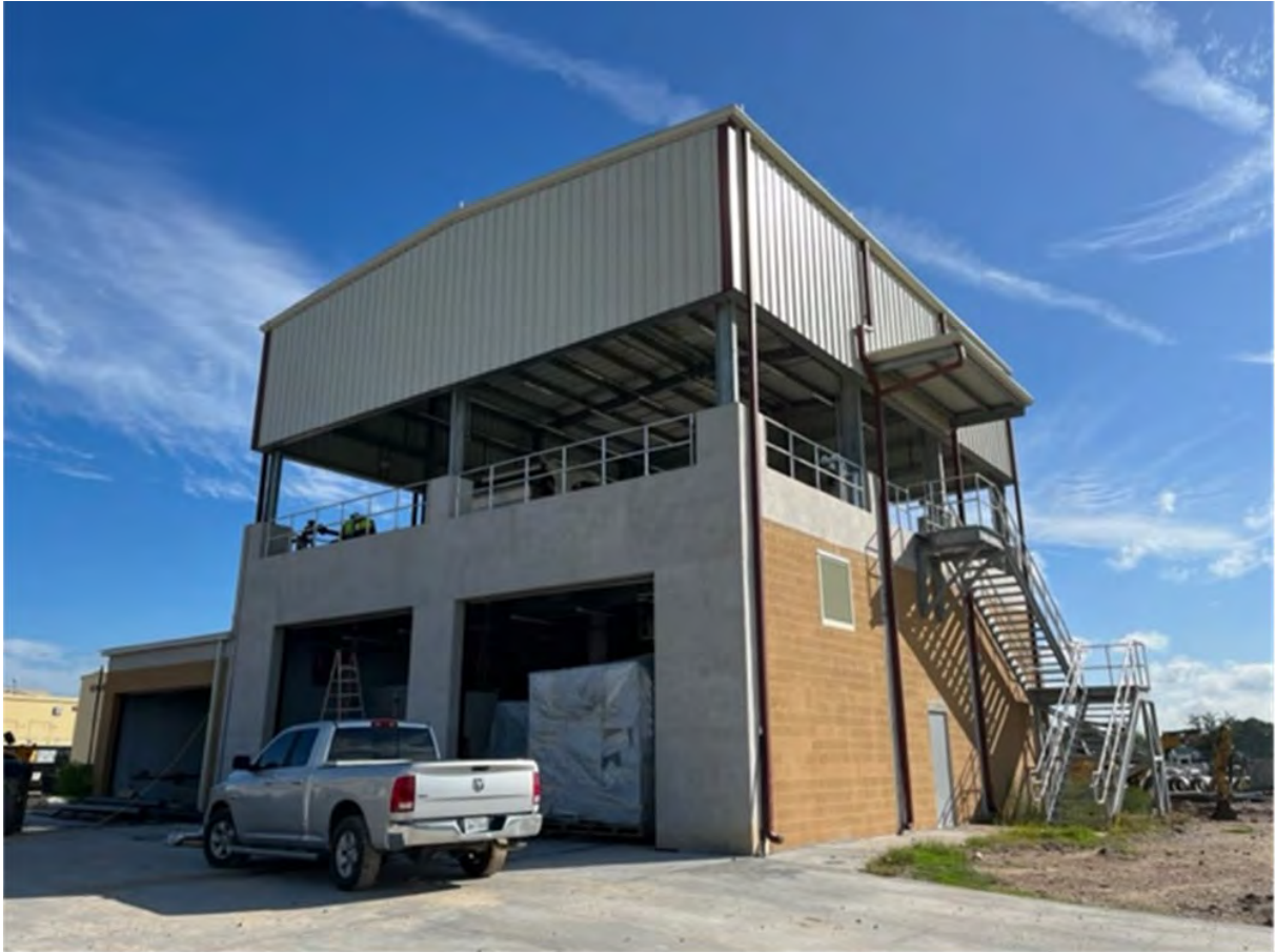
Substantially complete Sludge Building
