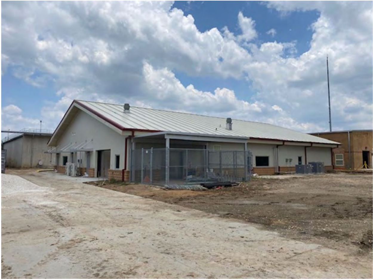
The Operations Building-exterior ready for site finishes
