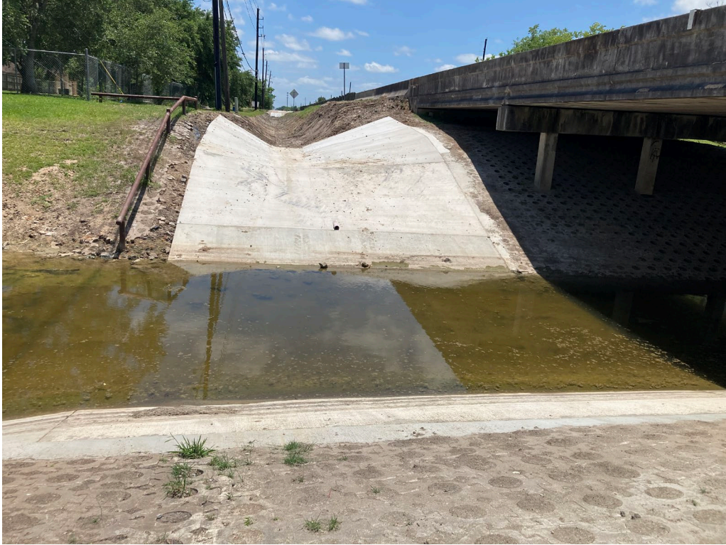
Slope Paving at Mary's Creek
