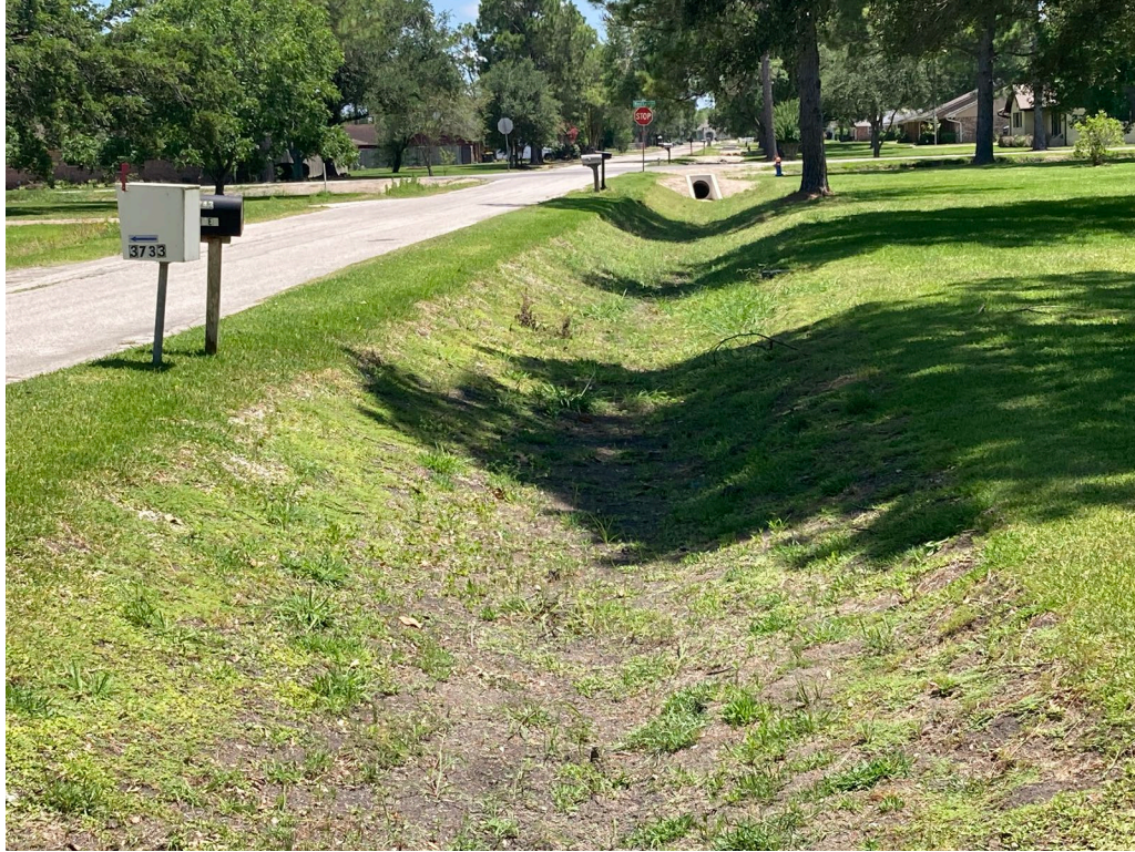
Graded Ditches along Wingtail Way at West Lea Lane
