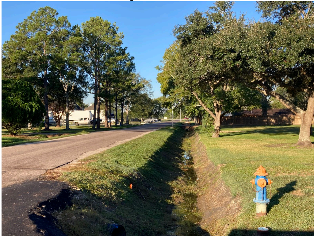
Ditches along Heron Lane
