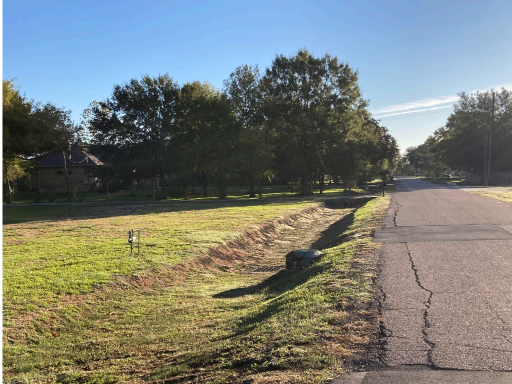
Ditches Along the North Side of Meadow Lane
