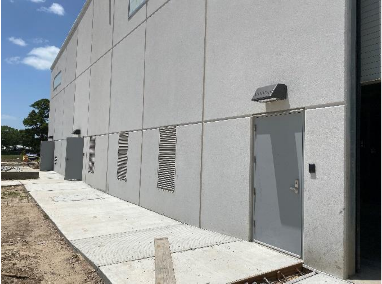
Sidewalk completed around Membrane Building
