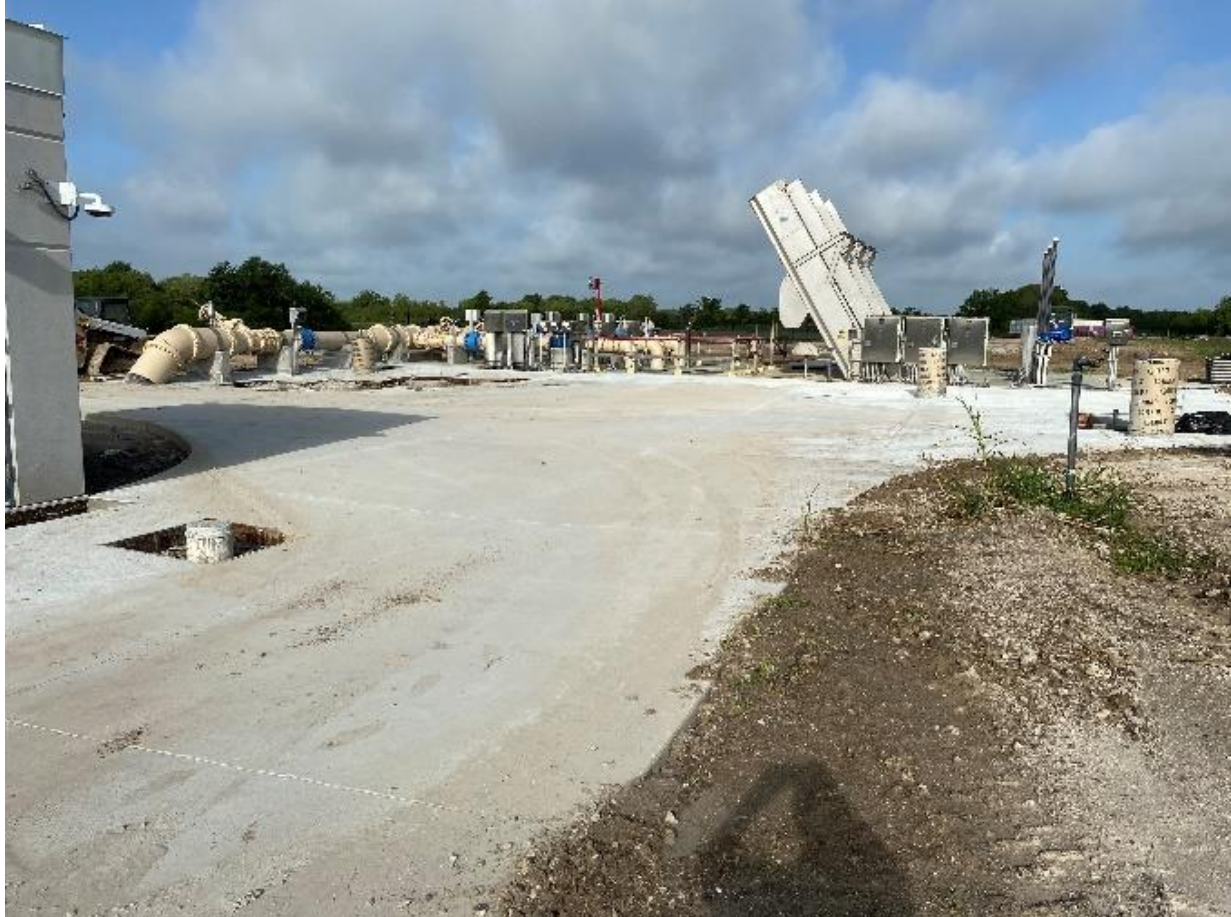
Raw Water Lift Station paving
