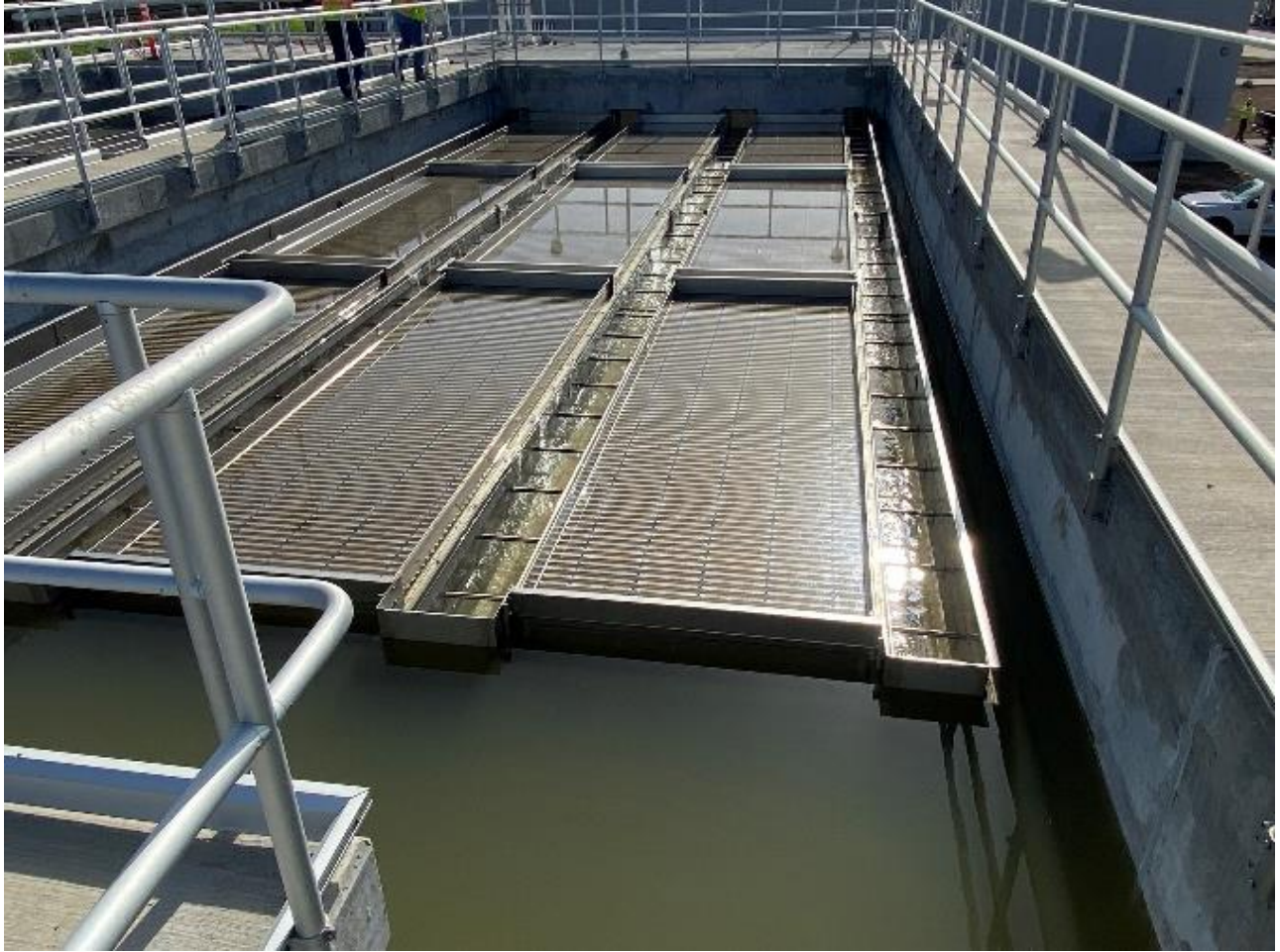
View of plate settlers in action, creating settled water for flushing (Loop 4)
