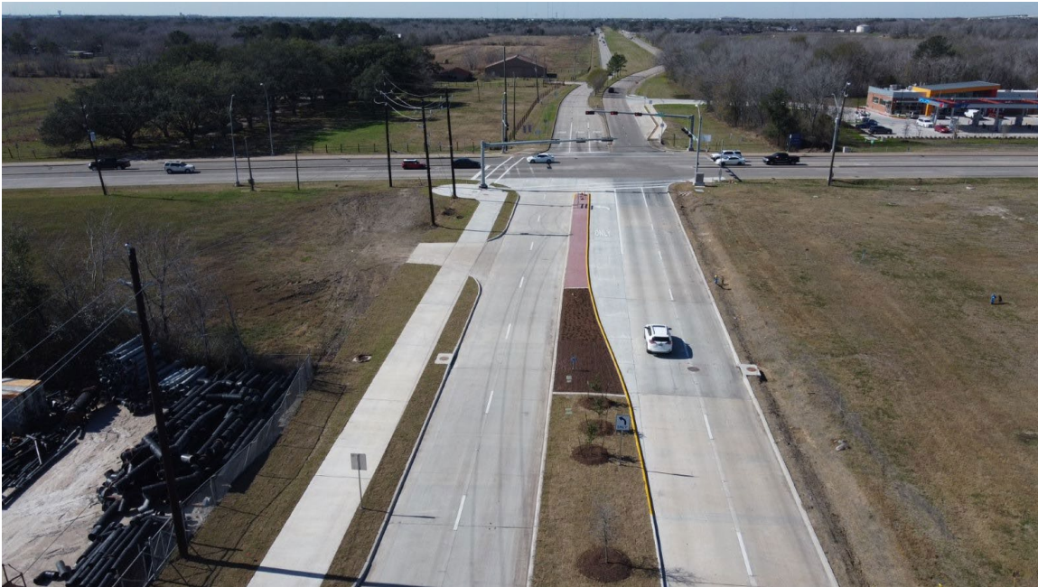
Cullen at McHard Rd. intersection, looking west.
