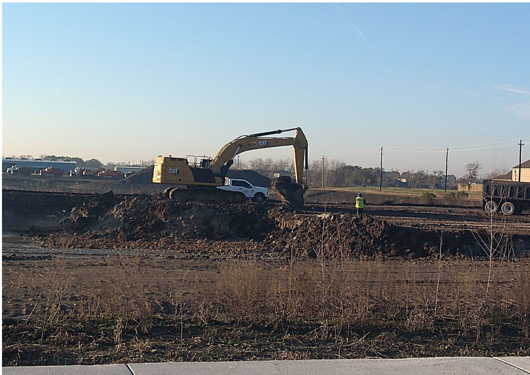
Excavating Hickory Slough Pond 2.
