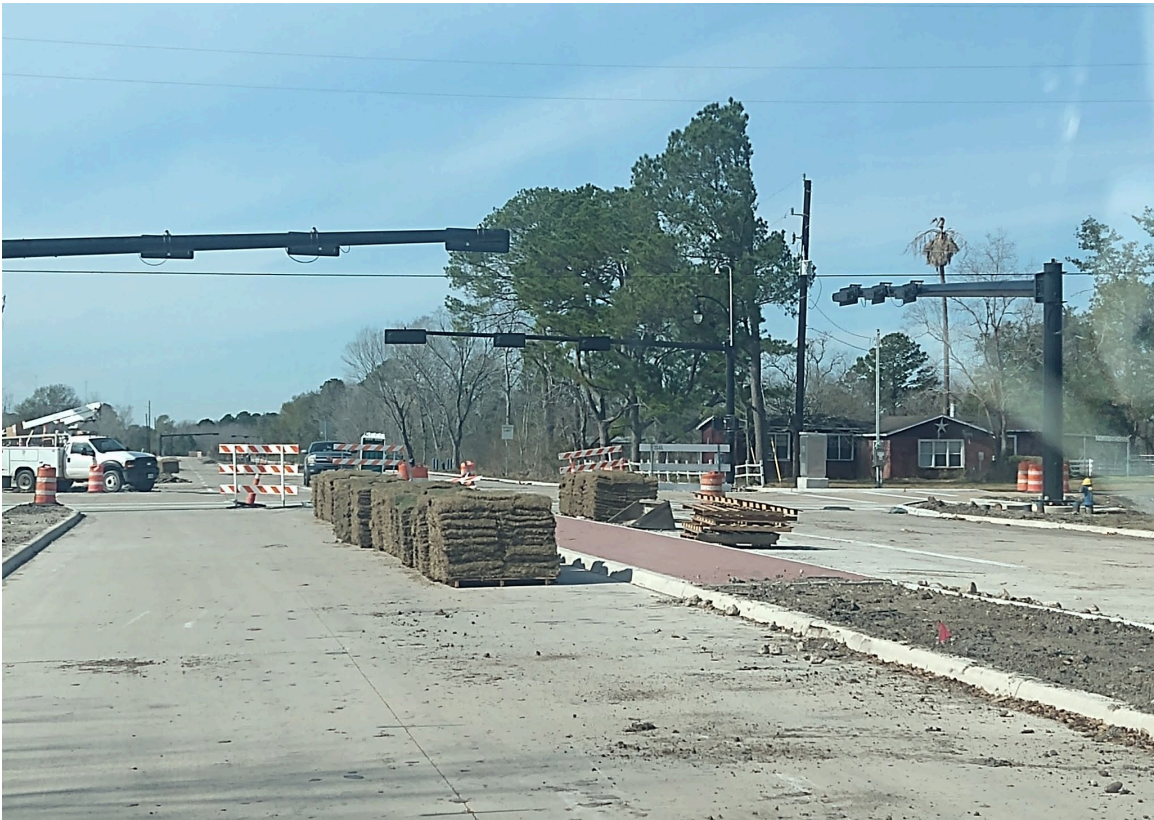
Laying sod in the median at Roy Rd.
