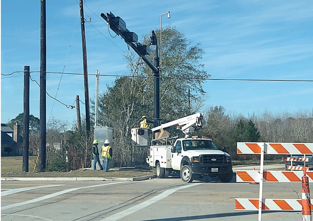
Energizing the traffic signal at O'Day Rd.
