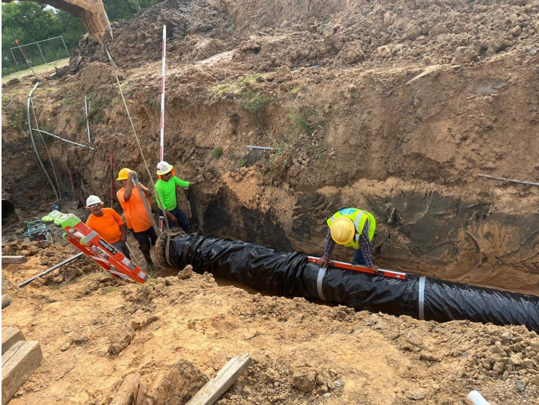
Installation of gravity line to backwash pond
