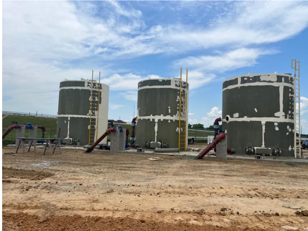
Exterior painting on all 5 aerators underway
