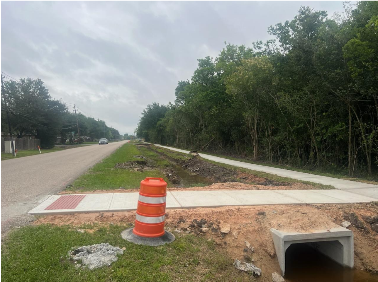
Sidewalk and pedestrian crossings along Knapp Road.
