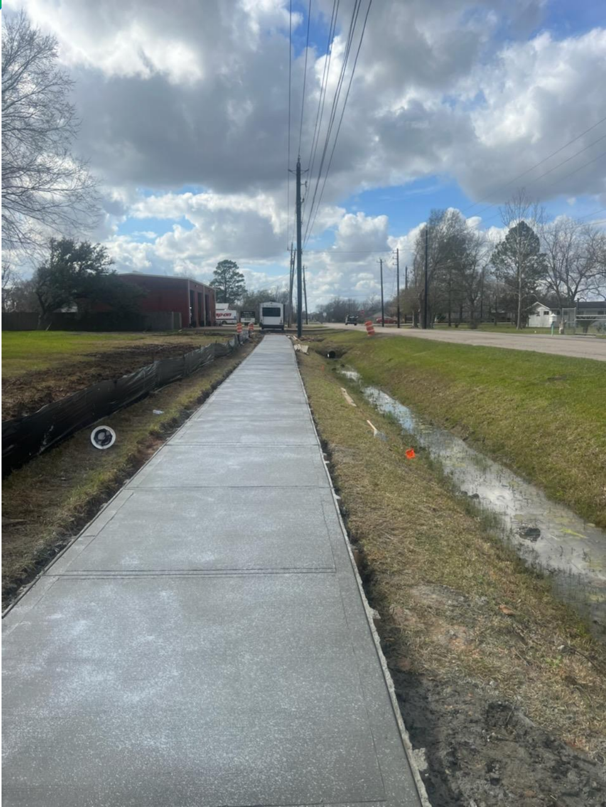
Freshly placed concrete sidewalk on Fite Road, south side.
