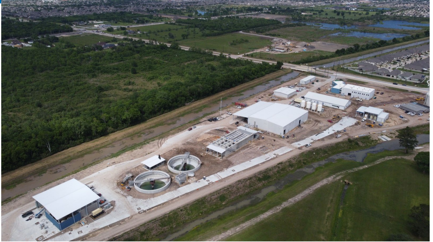
High altitude shot of overall site showing roadway pavement progression
