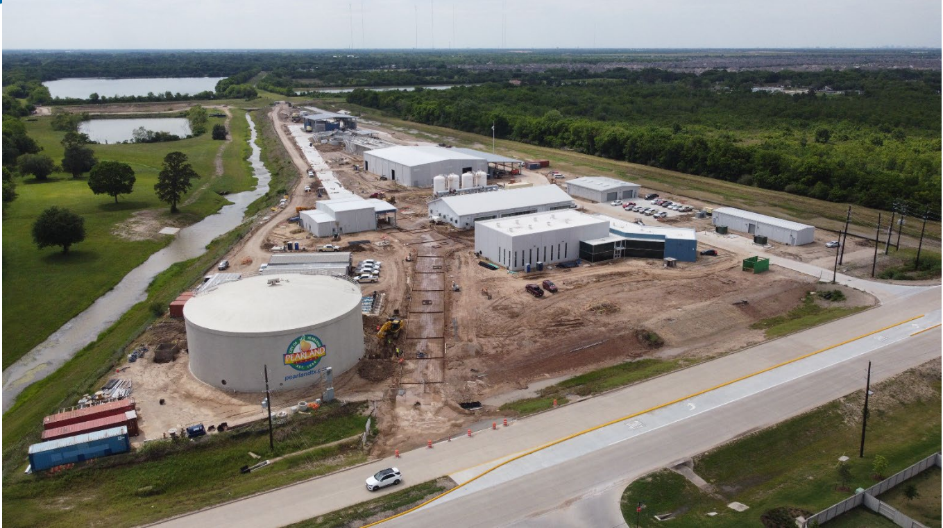
Above, Paving forms for south driveway, plant exit
