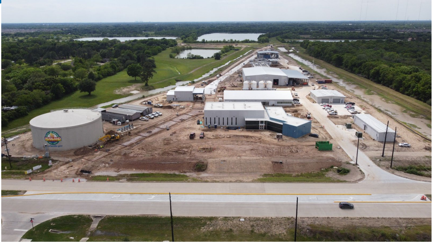
Westerly view from County Road 48 showing roadway progression
