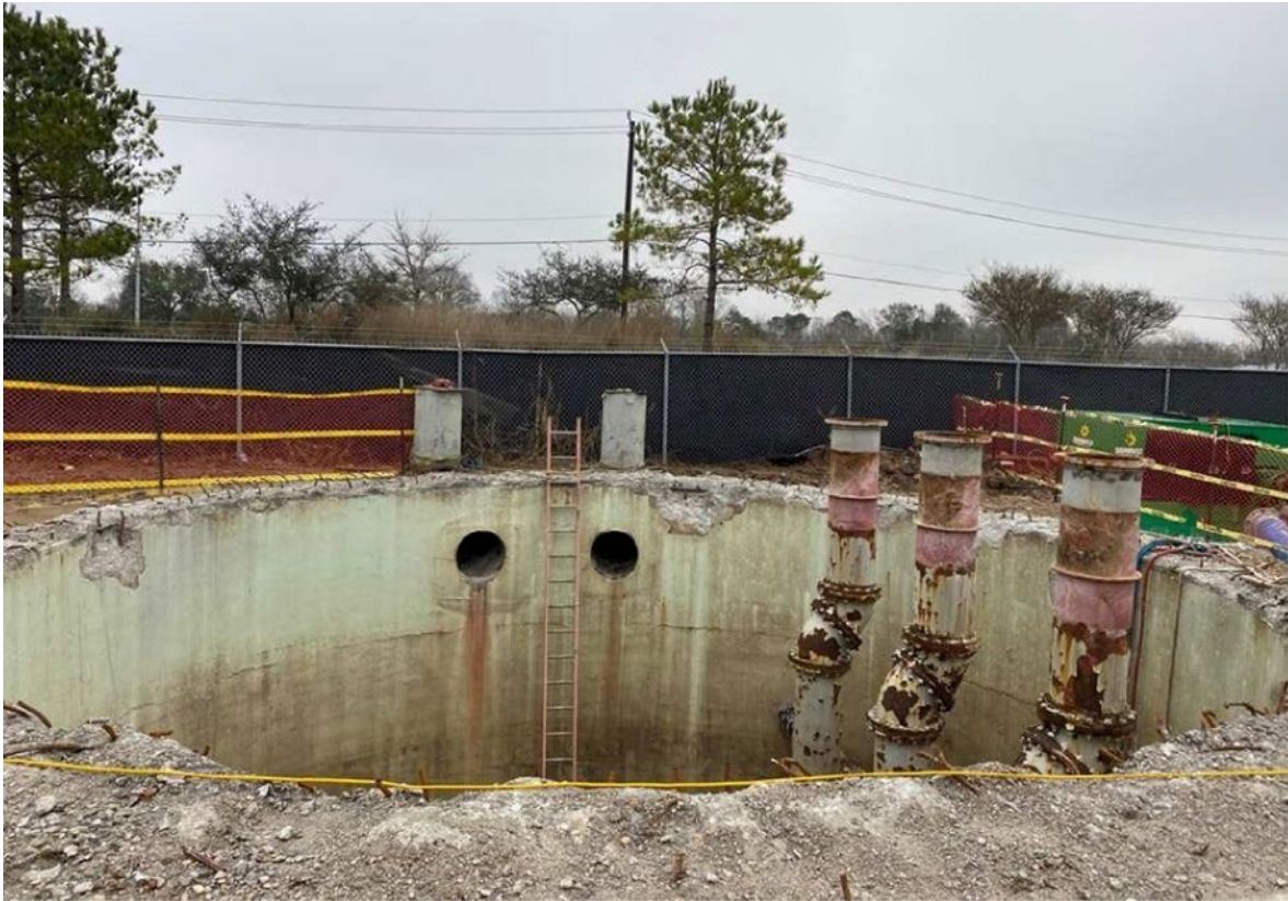
Demolition of Lift Station #2
