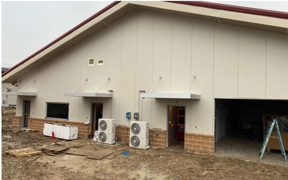
The Operations Building
