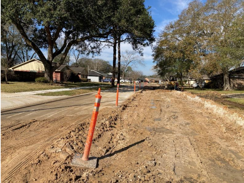
Concrete Paving, Sidewalks, and Driveways on the South Side Plum Street
