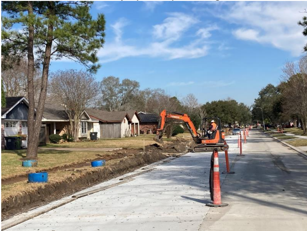
Concrete Paving on the West Side of Willow Blvd
