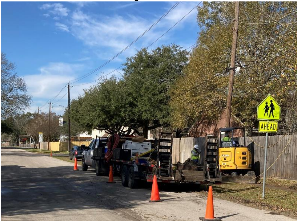
CenterPoint Energy Contractor Relocating the Gas Line on Cherry Street
