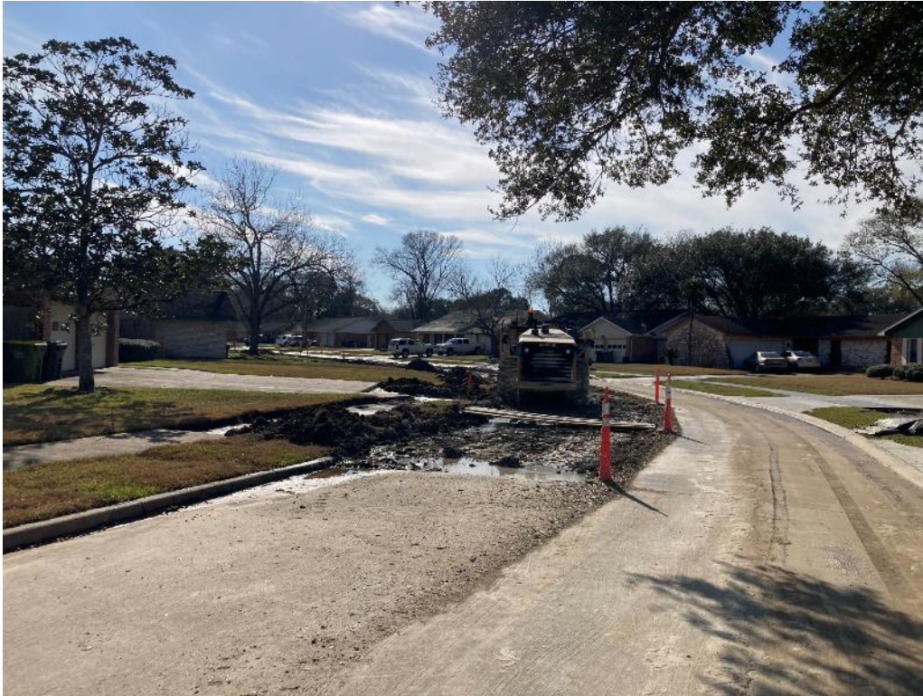
Second Mixing Lime on West Plum Street
