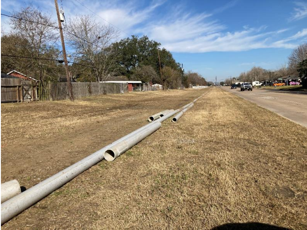
Sanitary Pipe for Pipe Bursting
