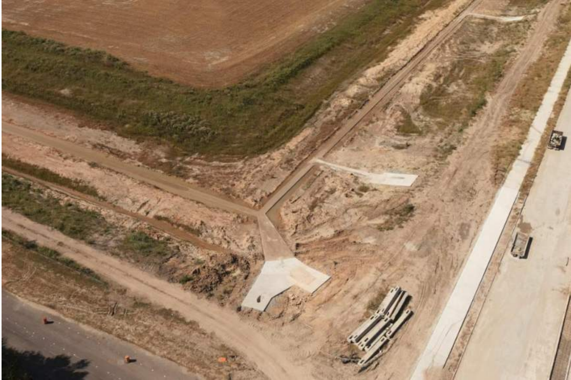
Hickory Slough Detention Pond 1 channel.
