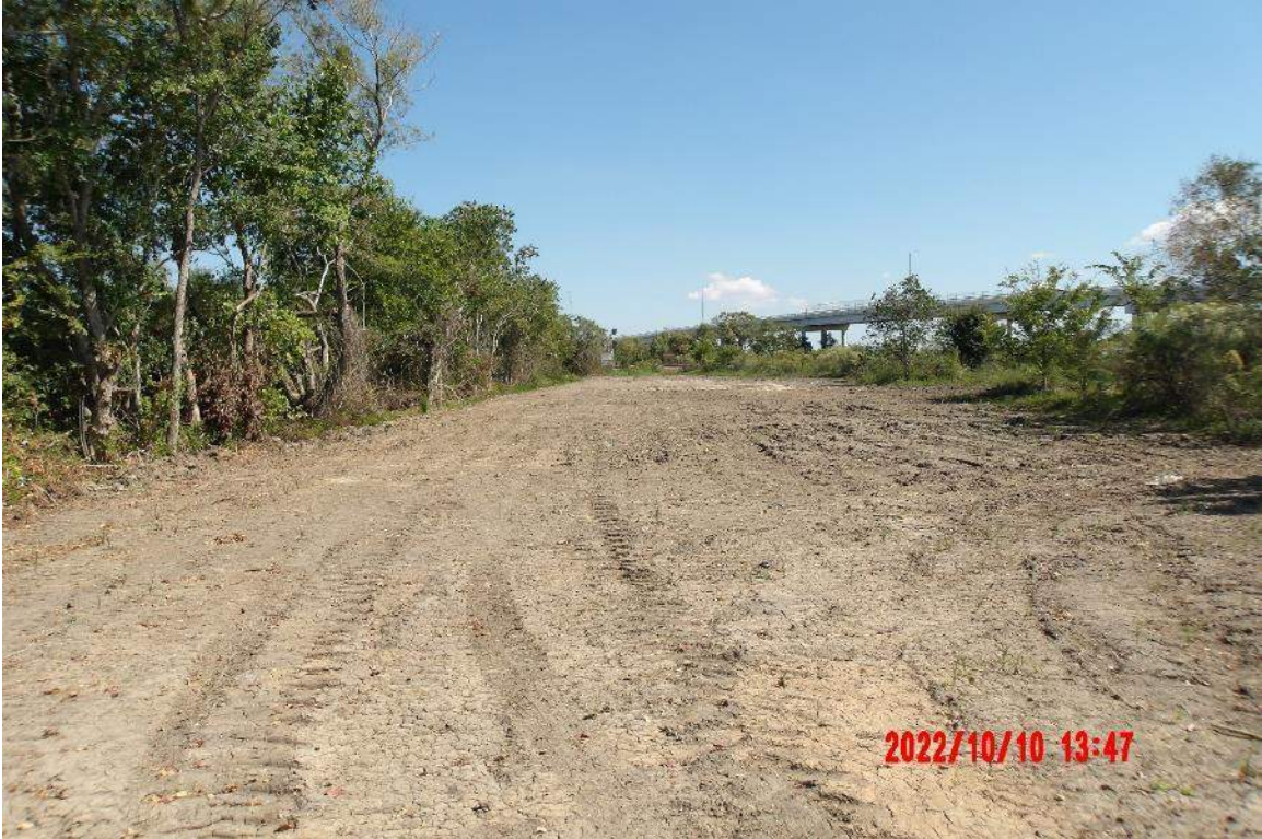
Magnolia Transmission Line Covered and Route Regraded
