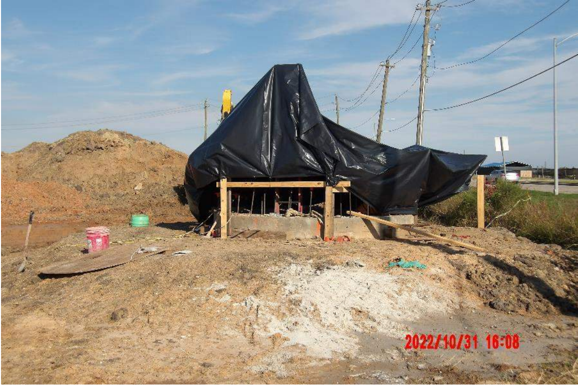
Station Walls Sunk to Final Elevation
