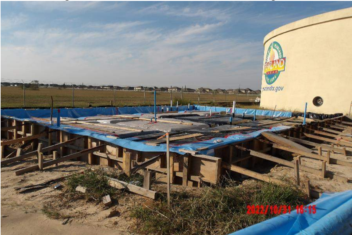
Control Building Foundation Formwork is Ready for Rebar
