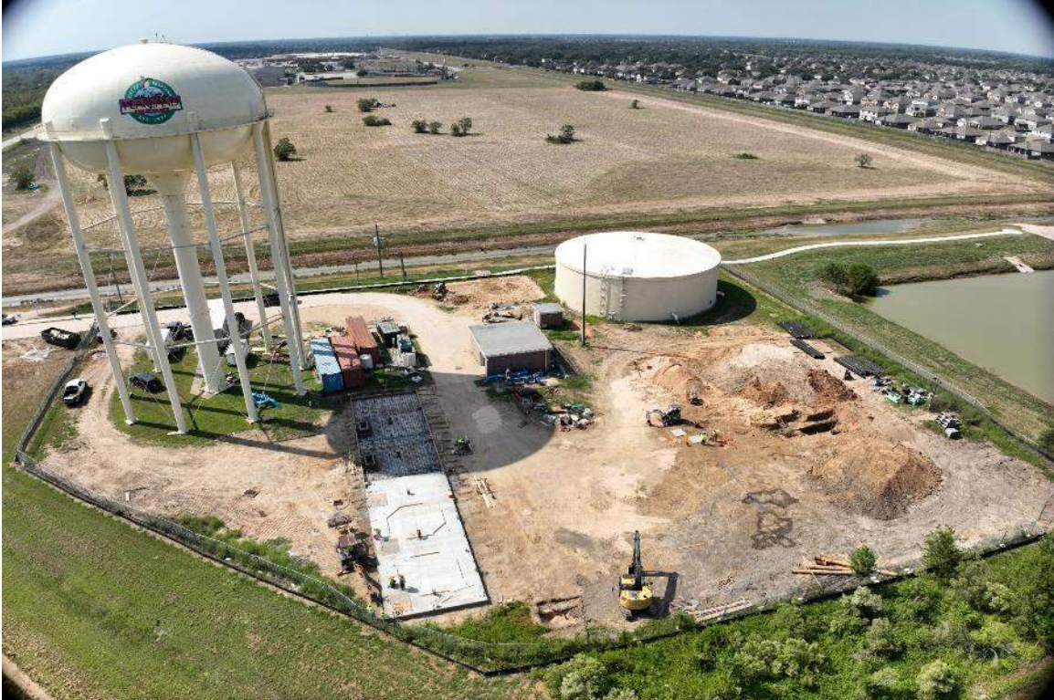
East Facing Aerial Image of Bailey Water Treatment Plant
