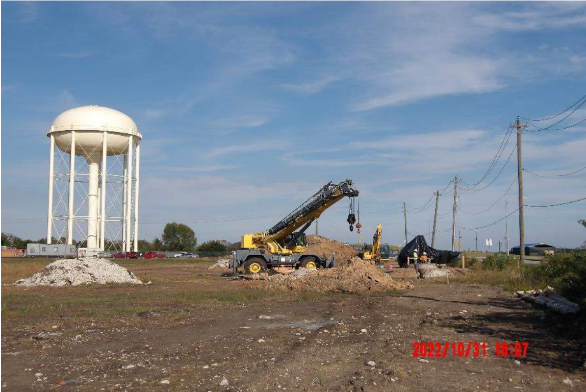
Lift Station Site with Station Walls Sunk to Final Grade
