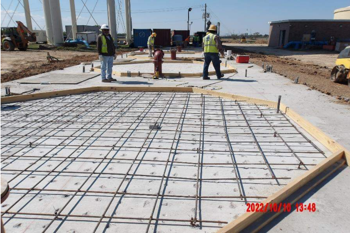
Aeration Equipment Pads Being Formed and Rebar Being Tied
