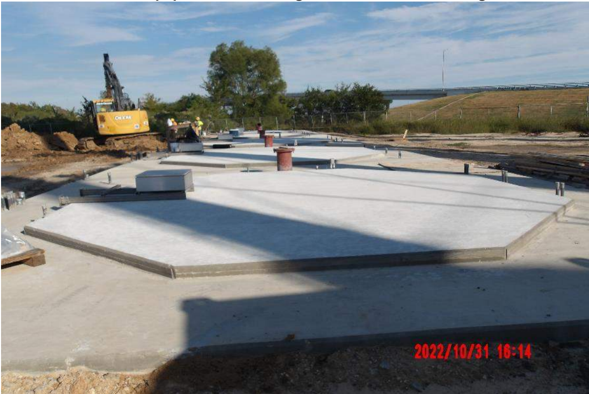
Aeration Equipment Pads Poured
