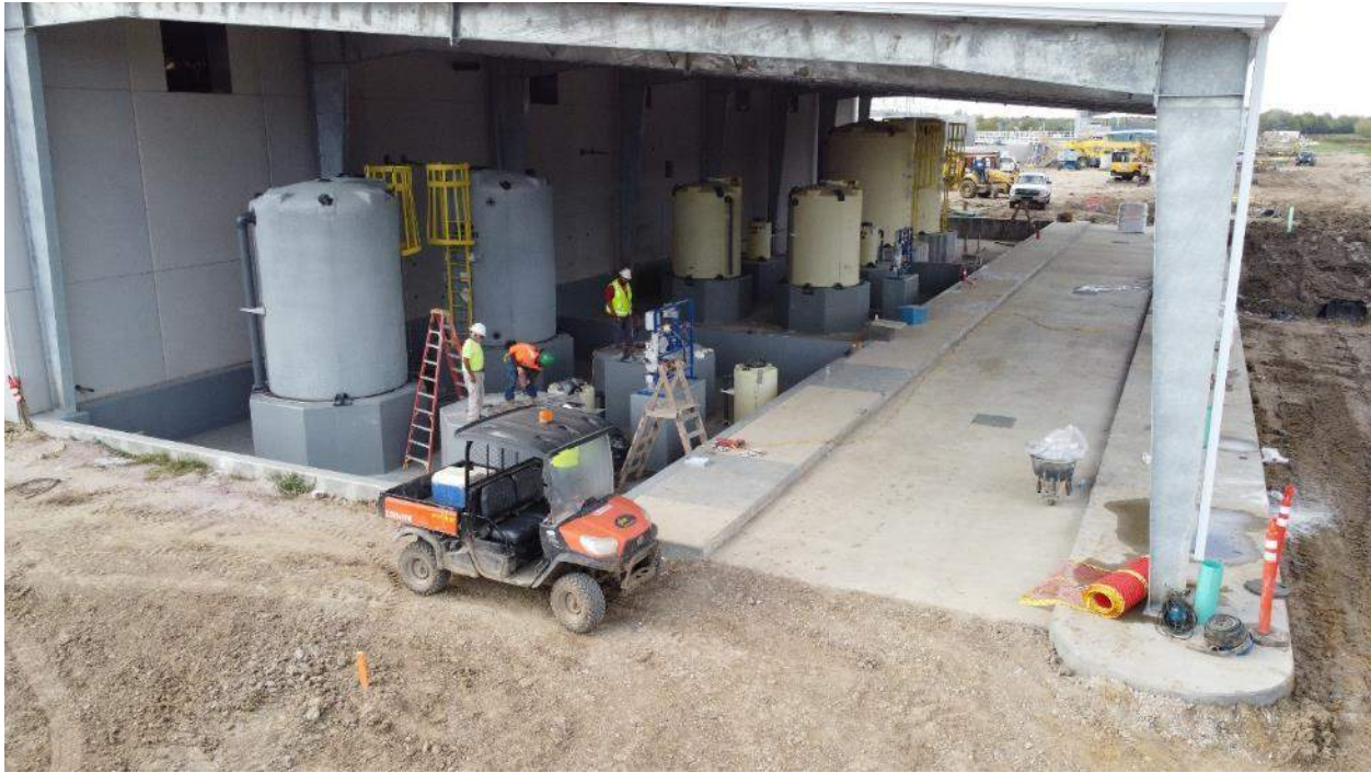
Bulk Chemical Storage and Truck Unloading Area
