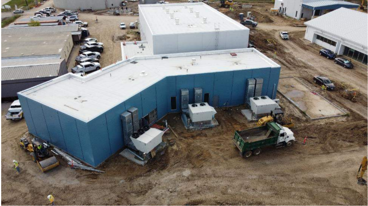
Back side of Administration & High Service Pump Bldg
