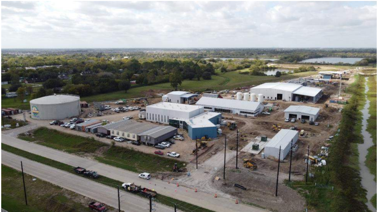
Overall Site from East looking West
