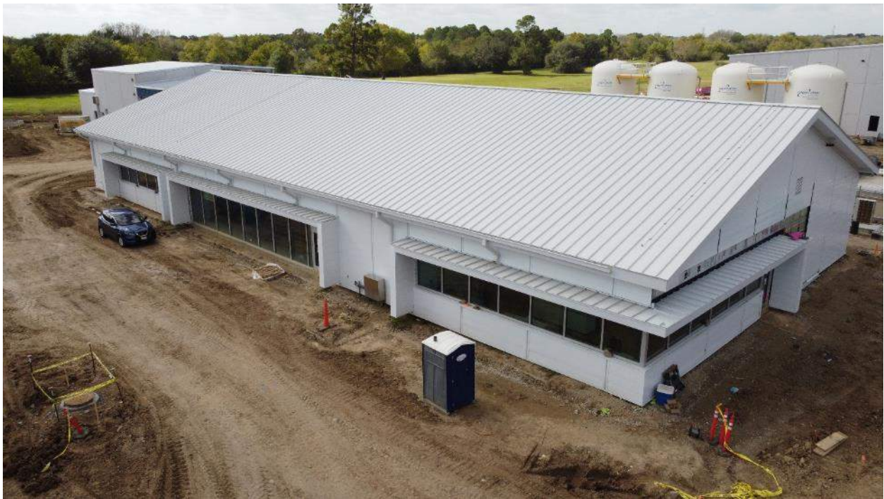
Operations Building with Control Room Windows in front right corner
