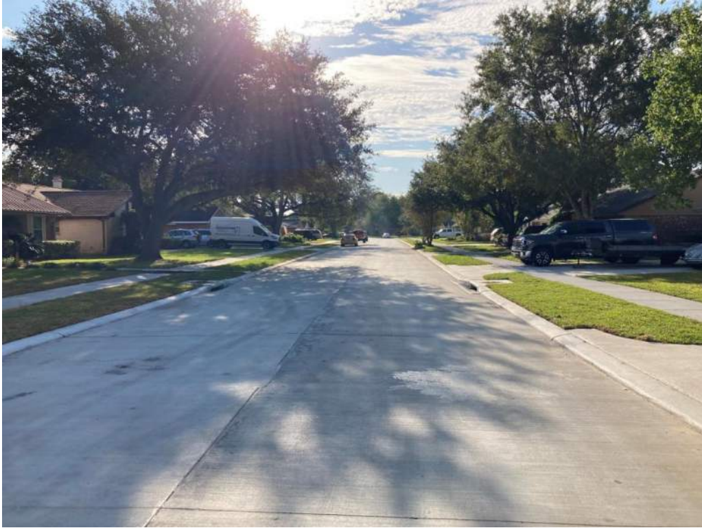
West End of Elm Street Completed
