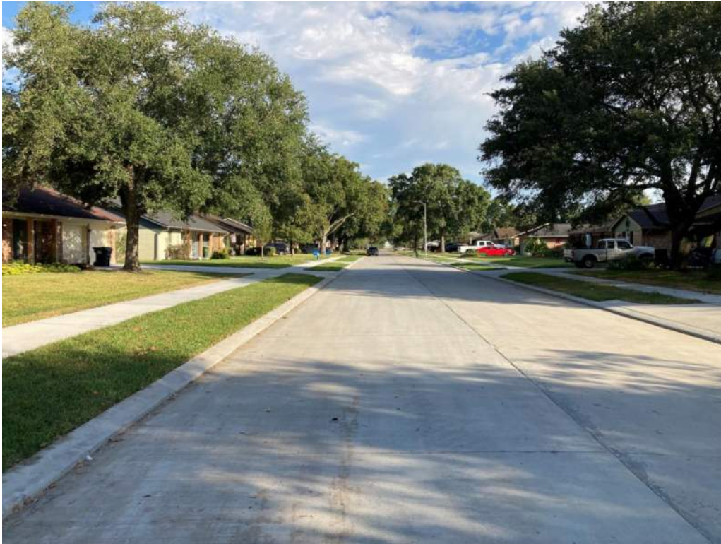
South End of Cedar Street Completed
