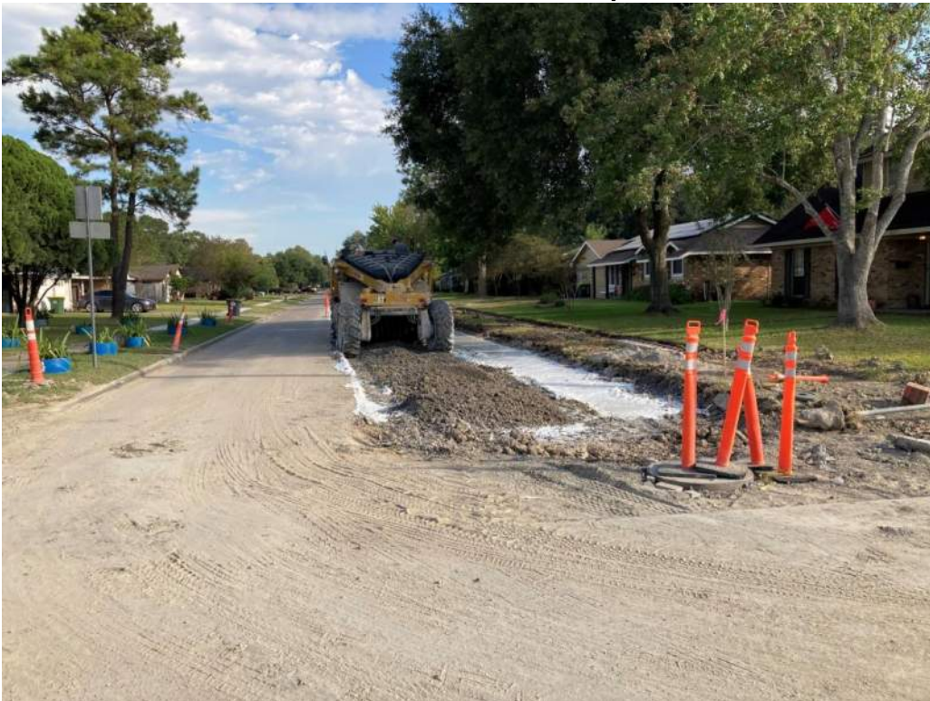
Installing Lime on South End of Willow Blvd
