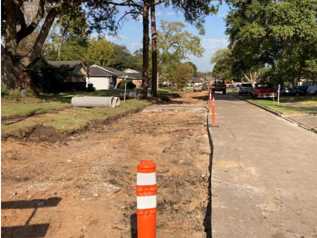
Removed Existing Street on the West End of Plum Street
