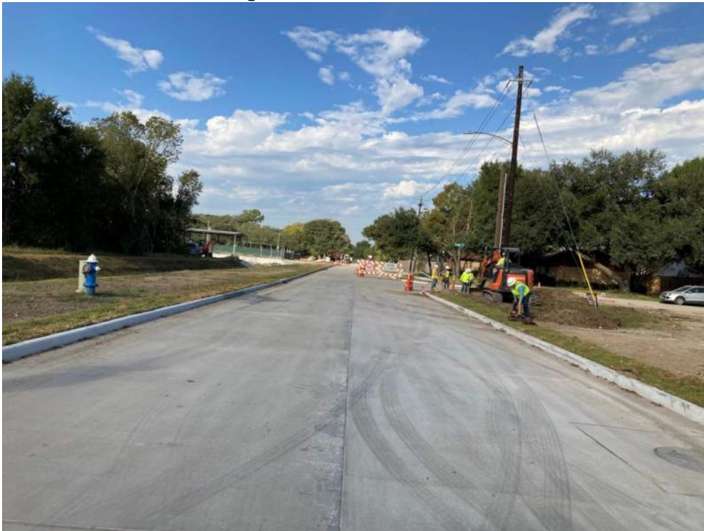
East End of Cherry Street Completed to Willow Blvd
