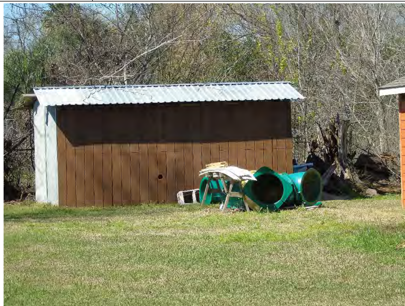
Camera facing west.
