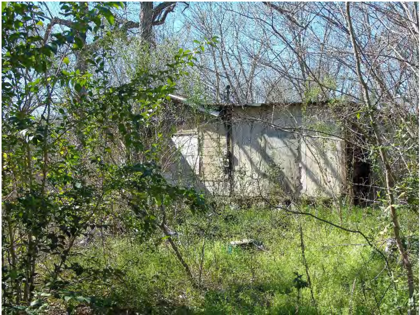
Camera facing west.
