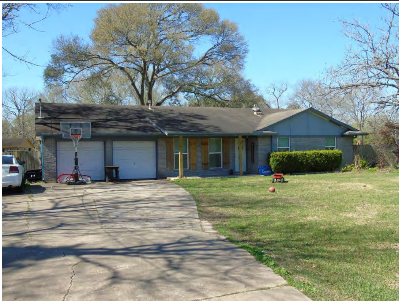
Camera facing west.
