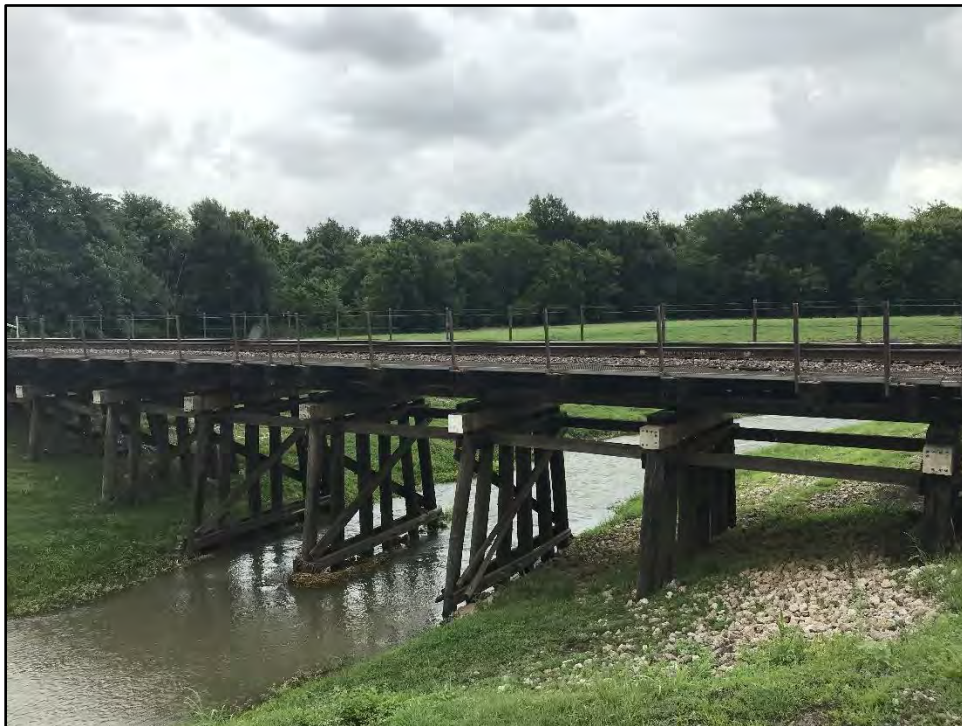
View of railroad bridge over Hickory Slough, facing northeast.
