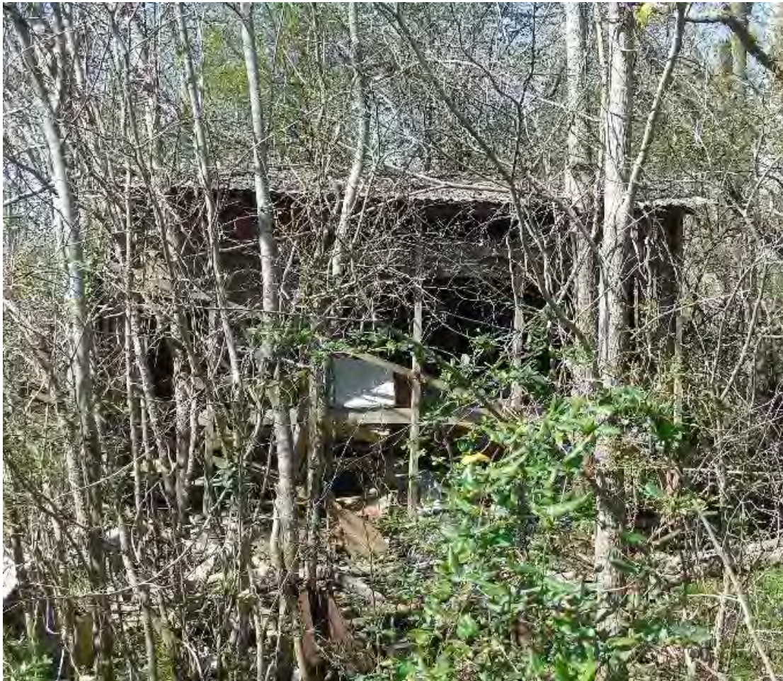
Camera facing west.
