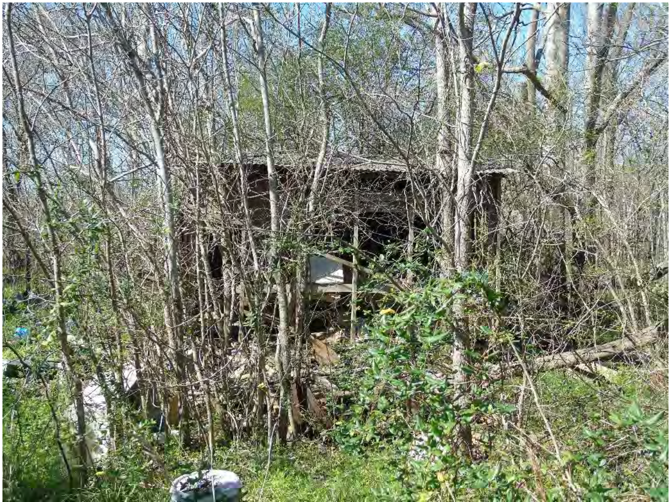
Camera facing west.
