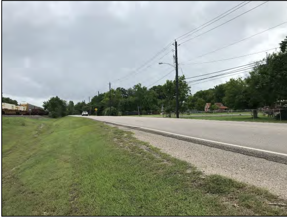
View of Mykawa Rd. at Isla Rd., facing south. Railroad track shown left in photo
