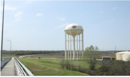
Bailey Water Plant Improvements $14.4M - Construction in Process at 20%
