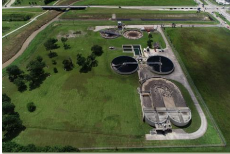
Barry Rose Water Reclamation Facility Replacement & Expansion $228.4M- Met 75% capacity and required to be in design
