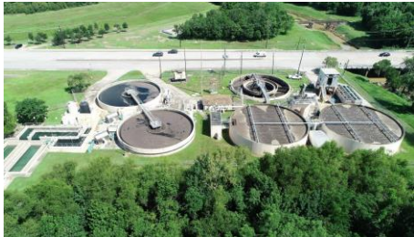
Longwood Water Reclamation Facility Decommissioning $36.2M- Met 90% capacity, required to construct expansion, exemption provided as service area is built-out
