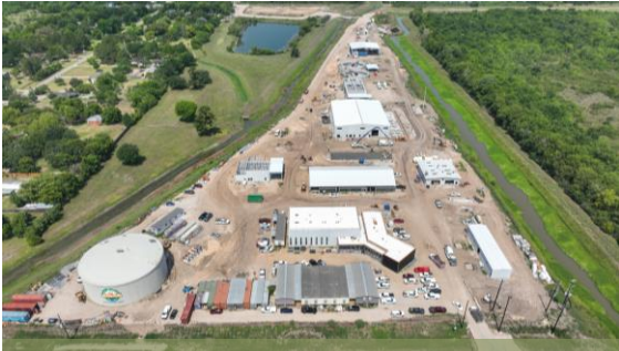
Surface Water Treatment Plant Operational in FY23 $175.5M - Construction in Process at 75%
