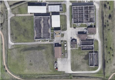
JHEC Water Reclamation Facility Expansion $80.6M - Construction in Process at 65%
