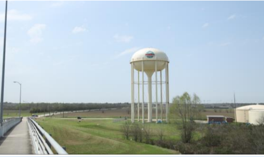
Bailey Water Plant Improvements $14.4M - Construction in Process at 20%
