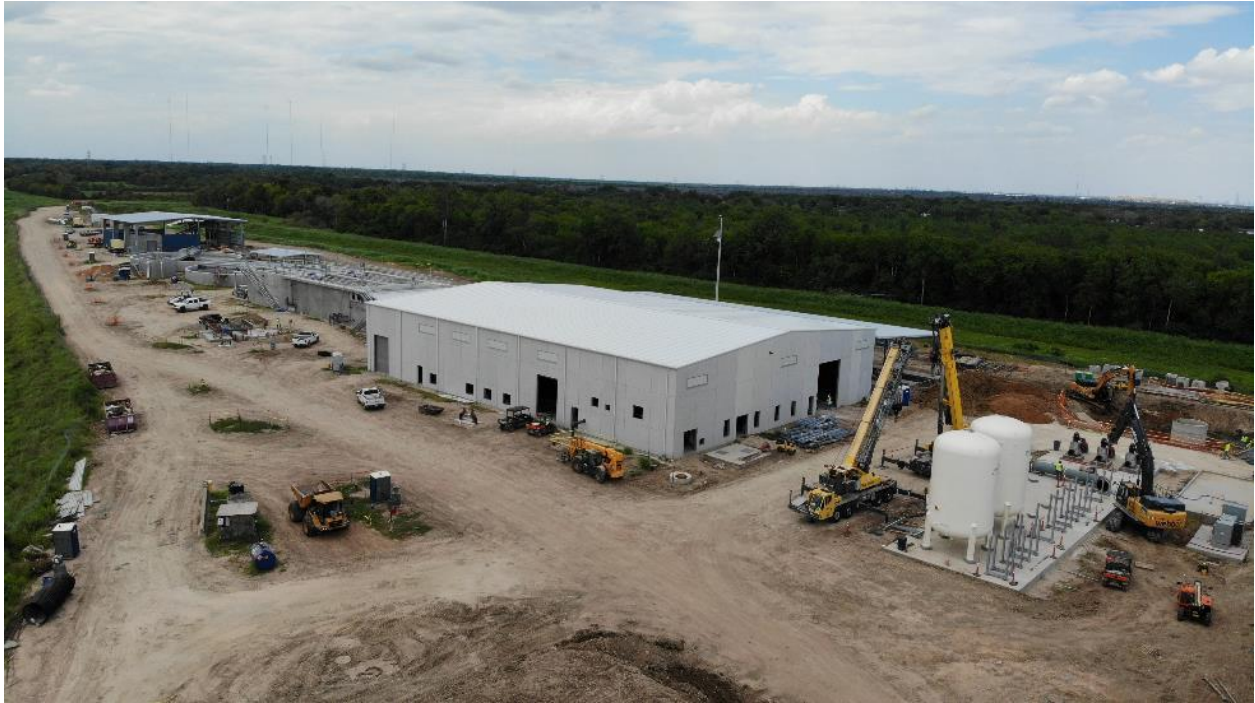
View looking north at the Membrane Building.
