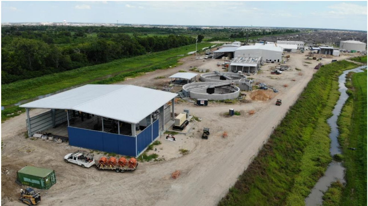
View looking east of the sludge press building and sludge thickeners
