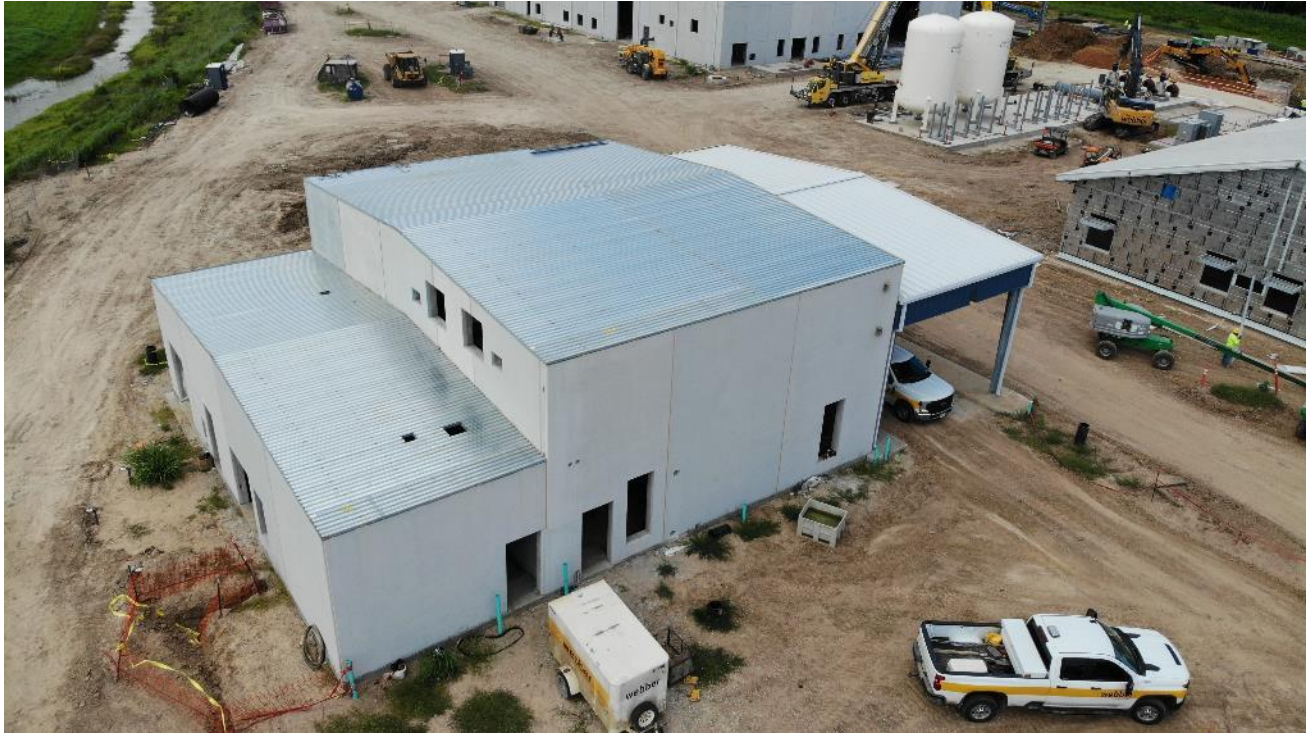
View of the Chlorine Treatment and Storage Building
