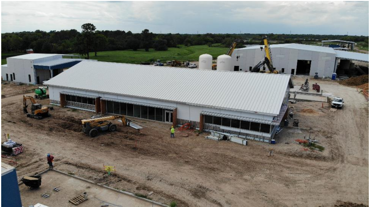
View looking at the Operations Building.
