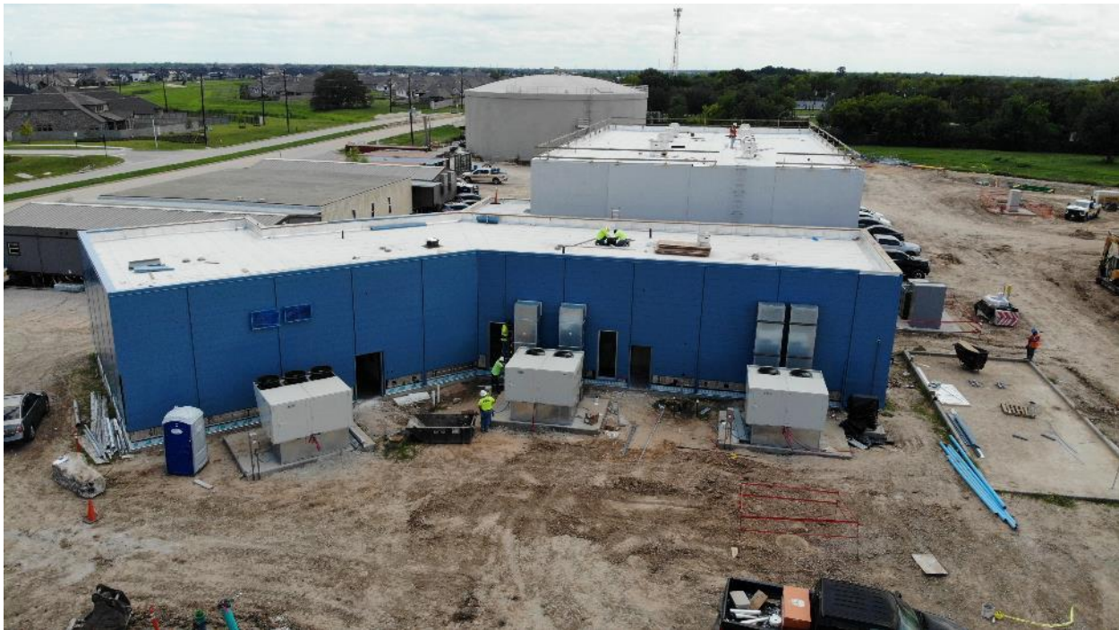
Aerial View of the back side of the Administration Building
