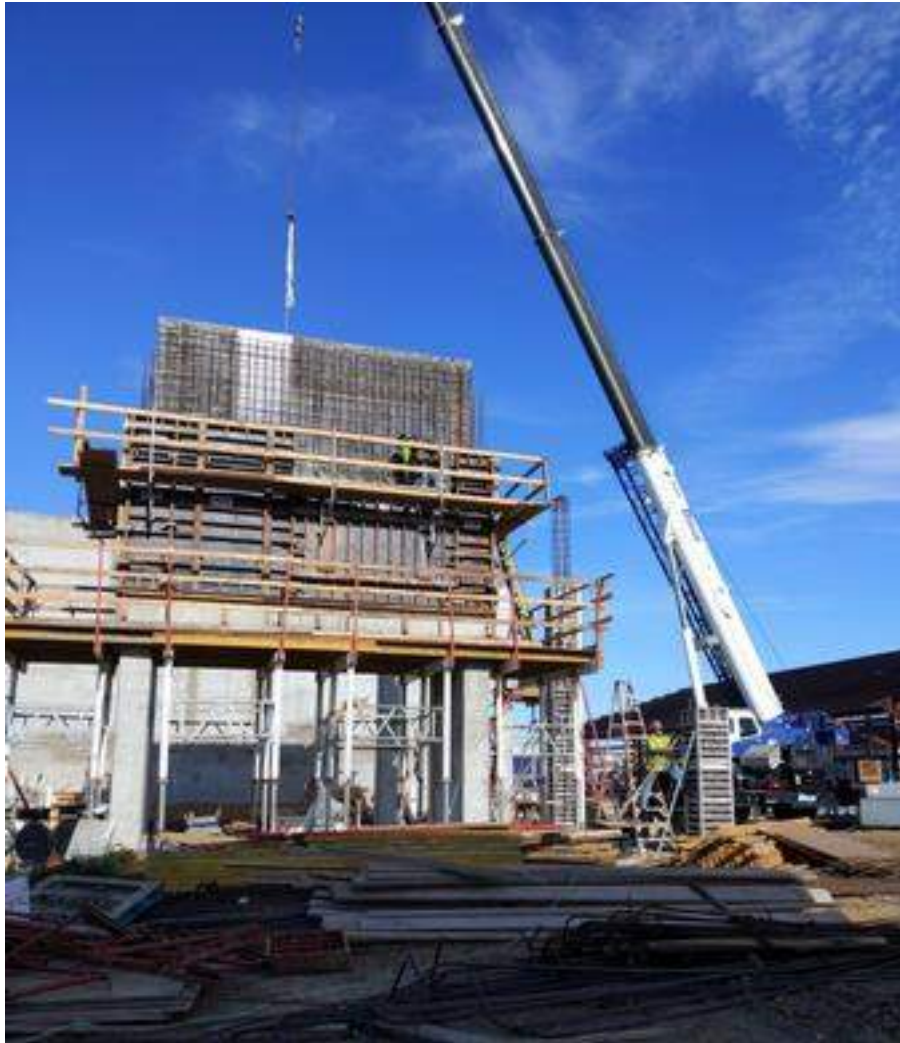
Setting forms and re-bar at the Headworks building
