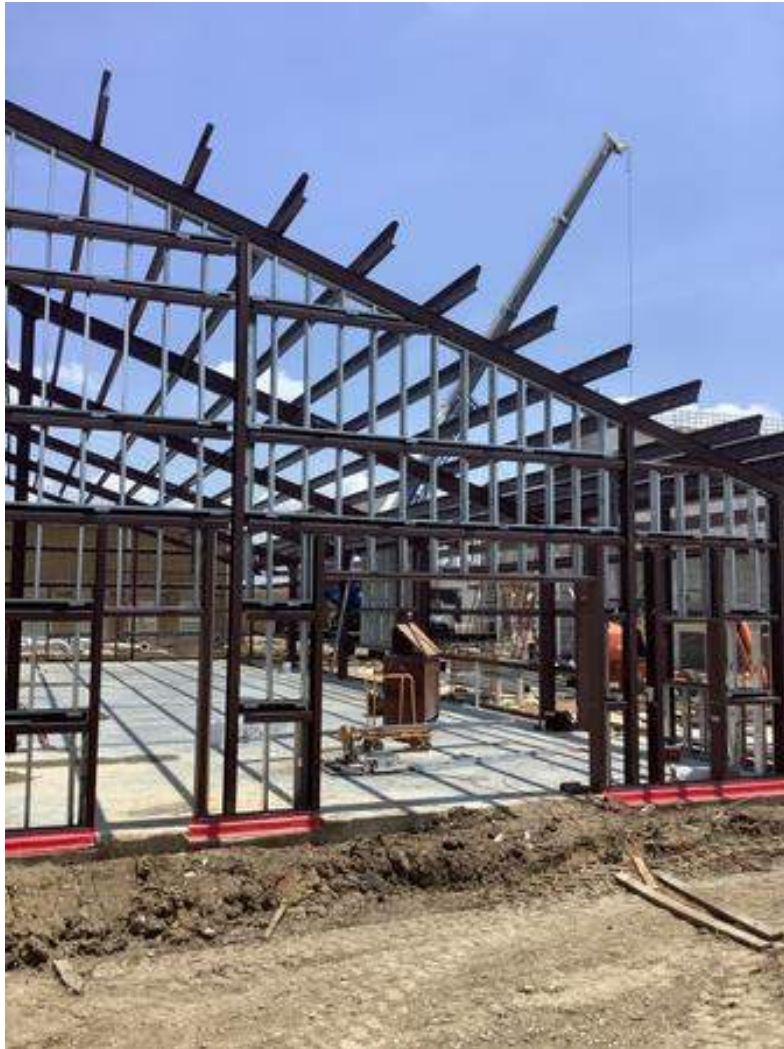
Operations Building Steel Structure
