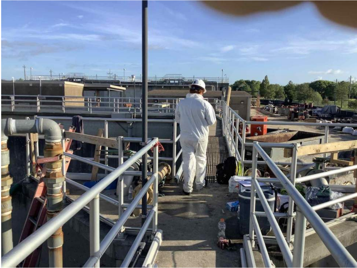
New walkway between SBR 4 and 5
