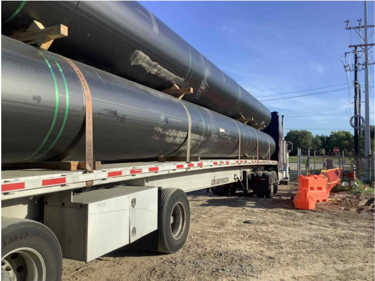
Large diameter HDPE pipe arriving on site
