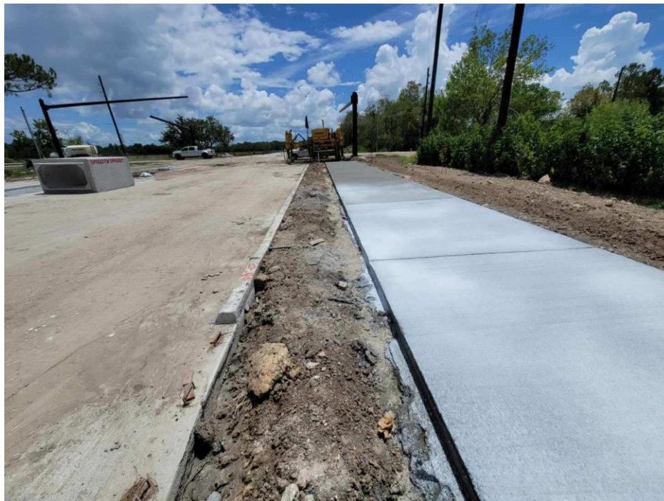
Sidewalk installation near Max Rd.
