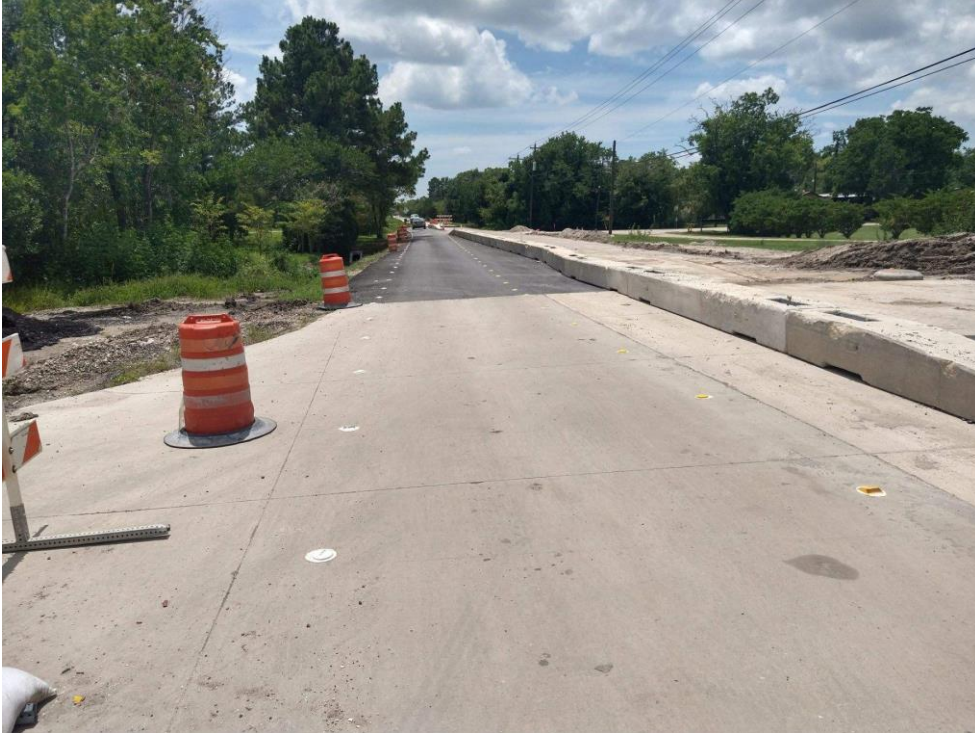
Asphalt paving on Stone Rd.
