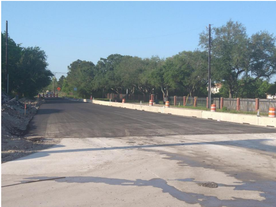
Asphalt paving at O'Day Rd., looking south.
