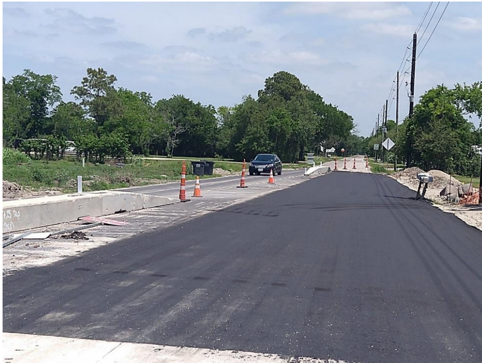
Asphalt Paving at Garden Rd.-southbound Lane.
