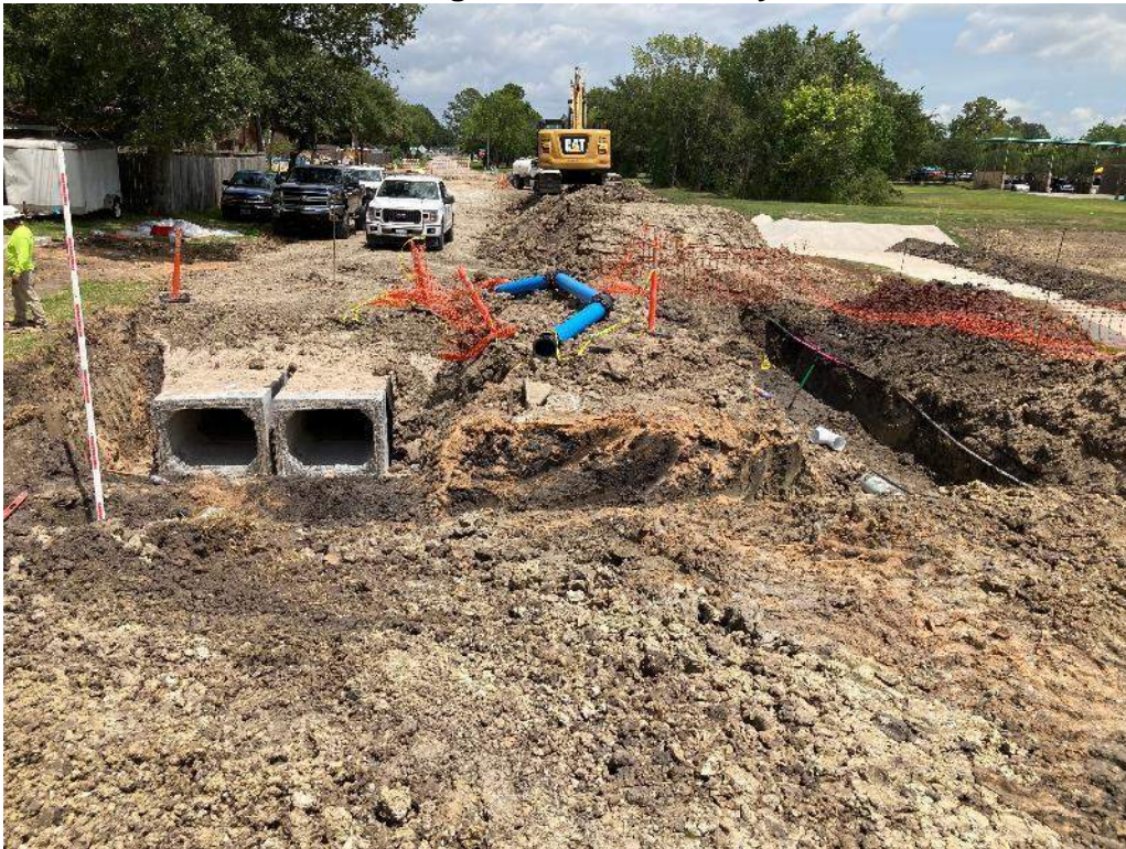
Installed Storm Boxes and Waterline Offset on Cherry Street
