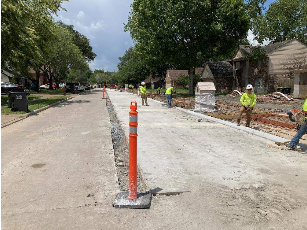
Installed Paving on the East Side Lynn Street
