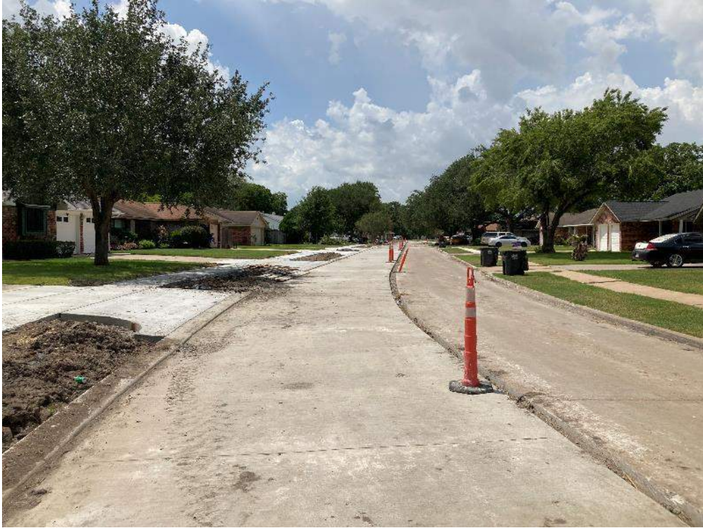
Installed Paving on South Side of Lynn Street
