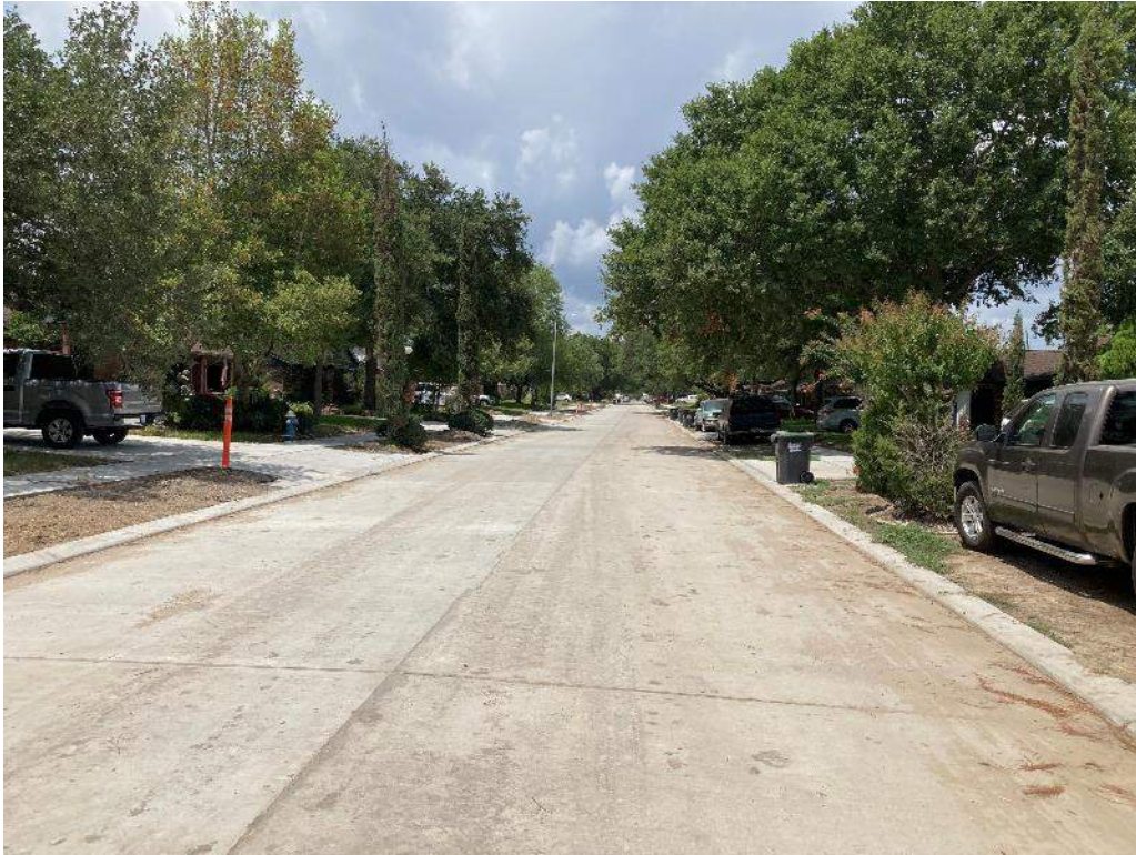
South End of Cedar Street
