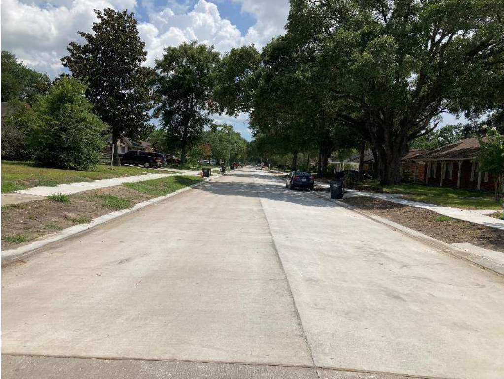
North End of Cedar Street
