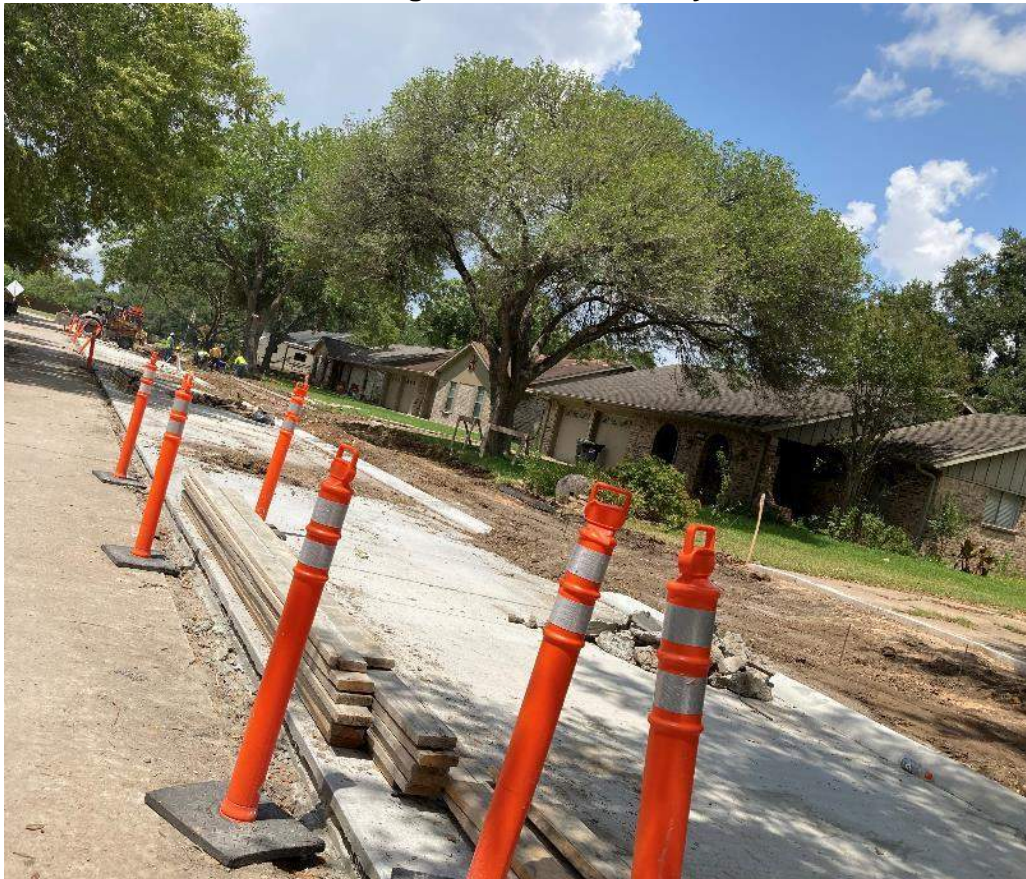
Installed Paving on the East Side of Rose Street
