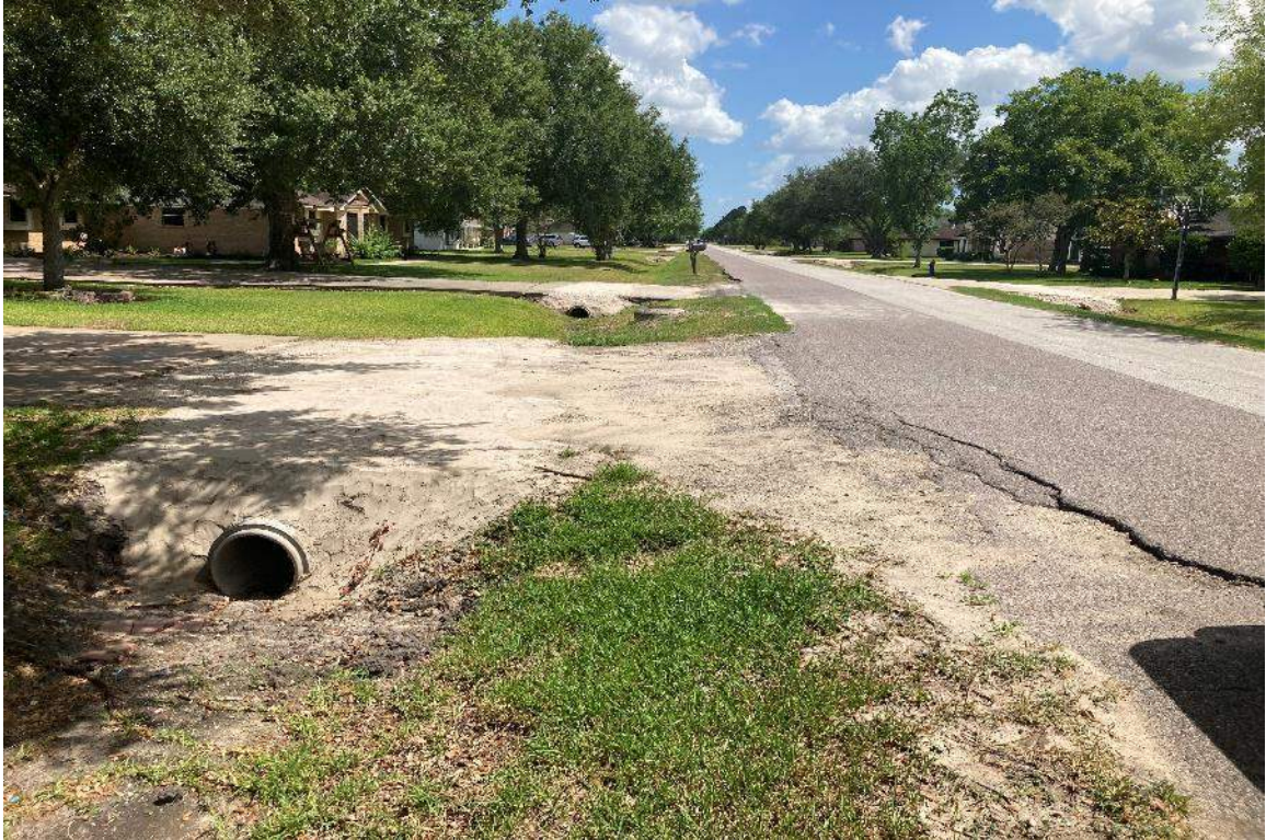
Driveway Culverts Wingtail Way Facing West Lea Lane
