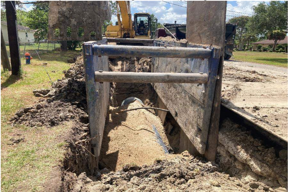
Installing 42" Storm Pipe Meadow Lane 20+00 Left
