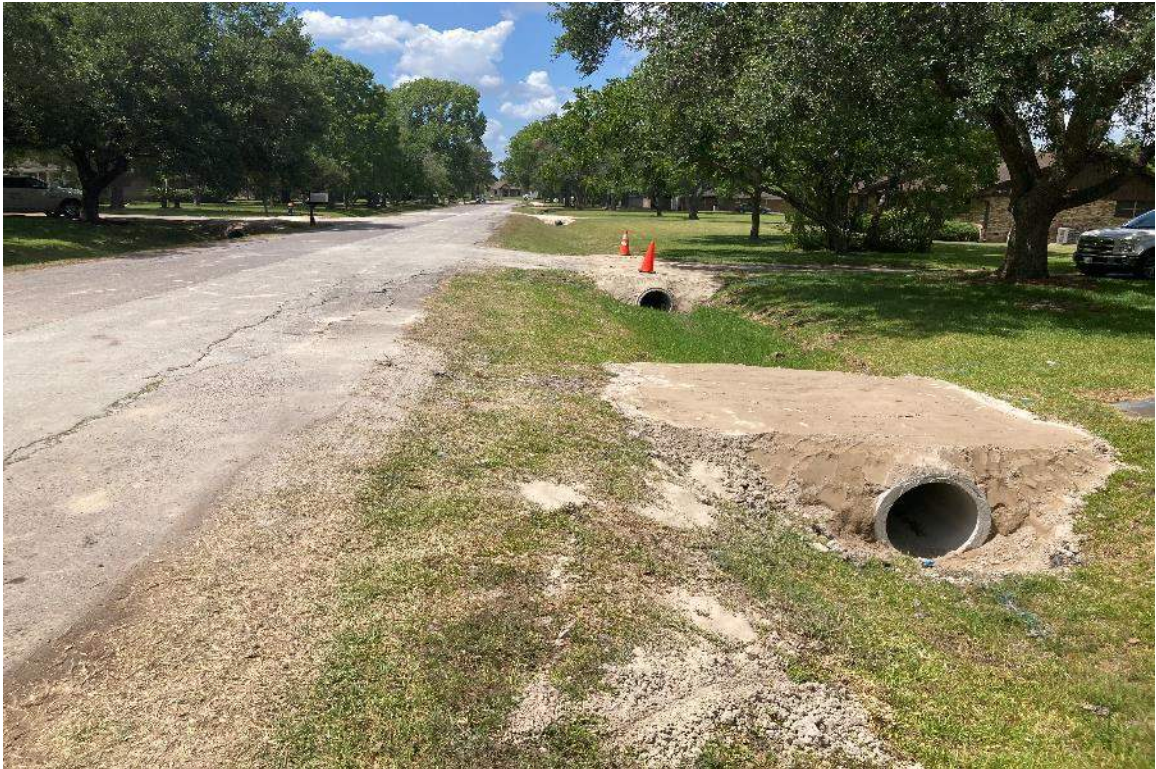
Driveway Culverts Skylark Way Facing Meadow Lane
