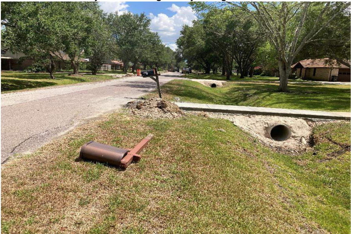
Driveway Culverts Meadowlark Way with New Concrete Paving
