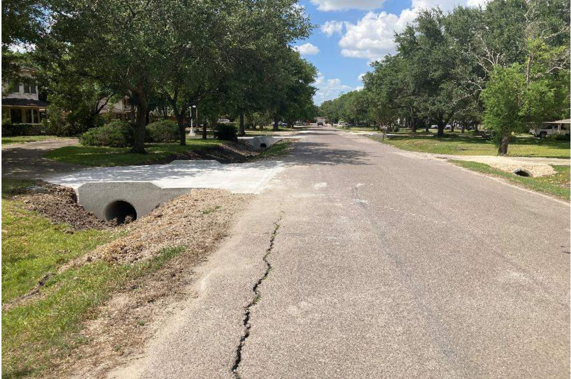
Driveway Culverts and Paving Bluebird Way facing Meadow Lane
