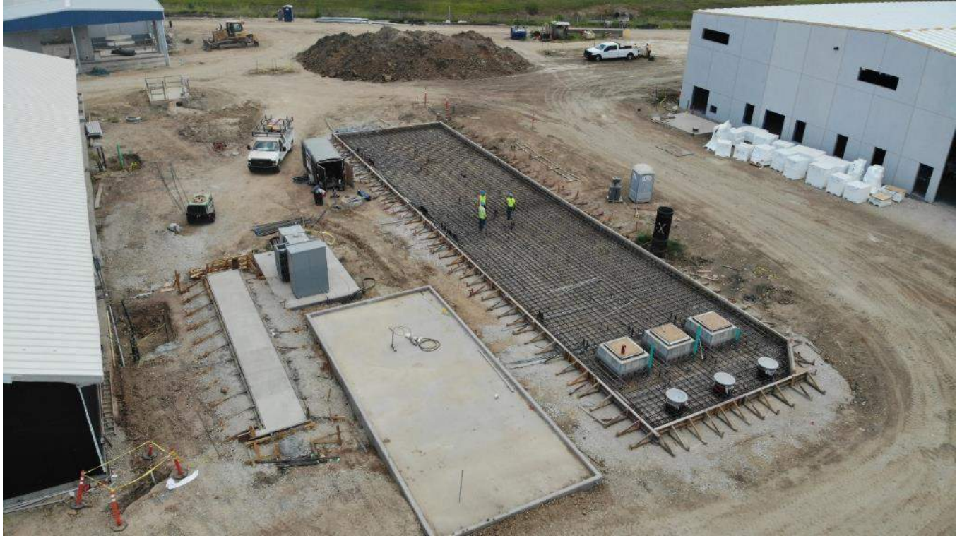
Granular Activated Carbon (GAC) filter foundation located between the membrane building and the back side of Operations.
