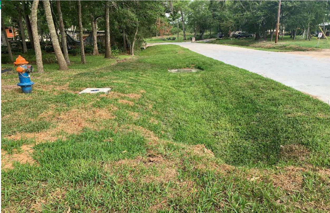
Sleepy Hollow Drainage Ditch Graded and Sodded
