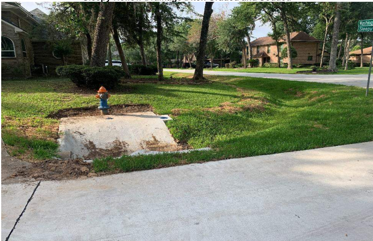
New Fire Hydrant and Slope Paving to Clear Creek Outfall
