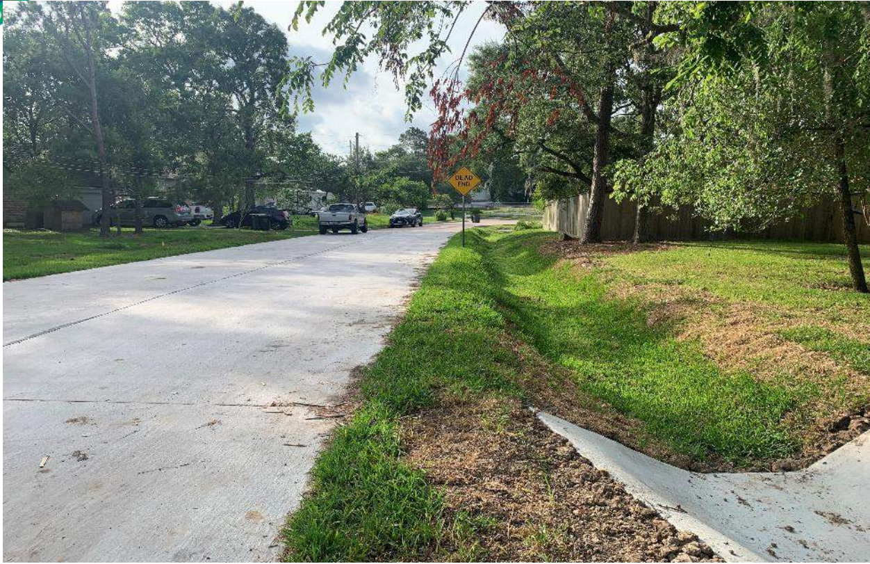
Sleepy Hollow Cul-De-Sac Drainage Ditch
