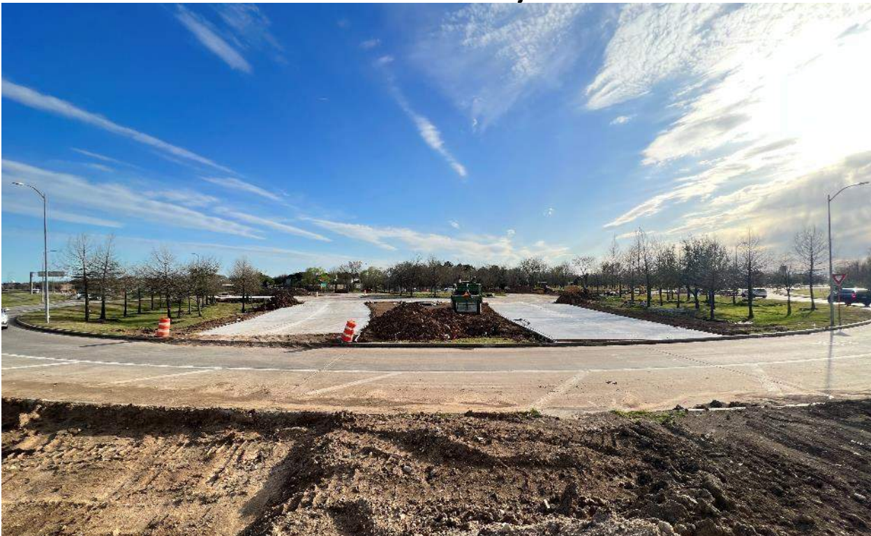
All Concrete Inside Existing Circle has been Poured
