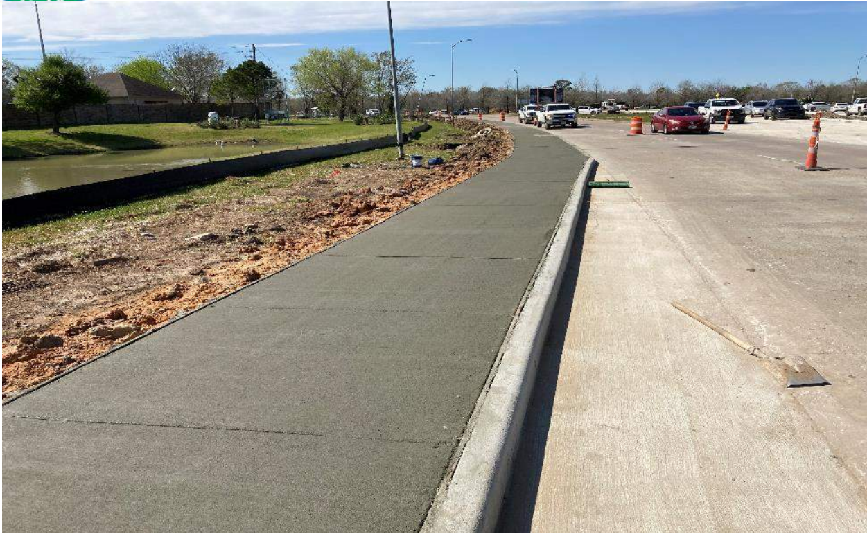
Sidewalk on Eastern Side of Pearland Parkway has been Poured
