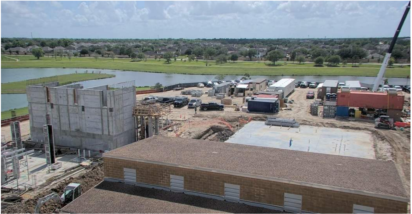
New slab for Operations Building
