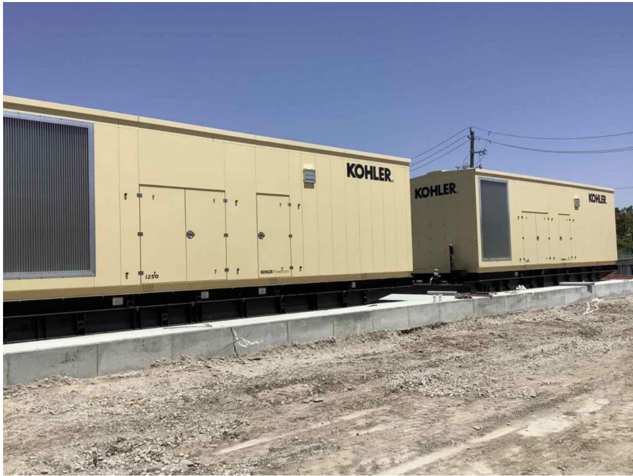
Preparing to set the Generators
