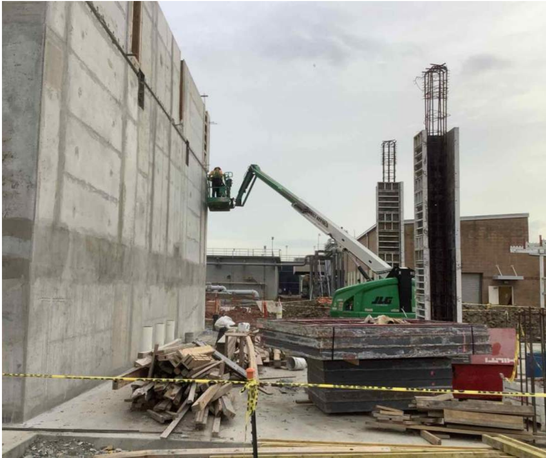
Headworks wall construction
