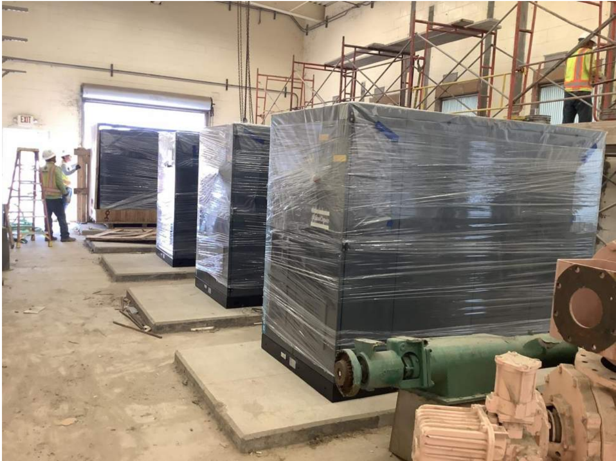
Blowers being installed in Blower Building #2
