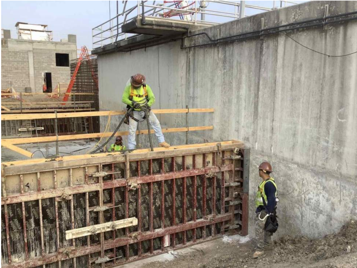
Construction of Splitter Box
