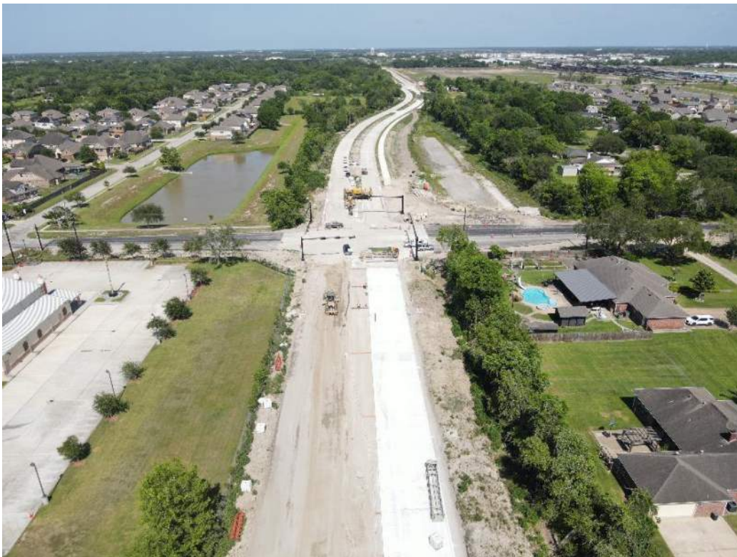
The intersection of O'Day Rd, looking east.
