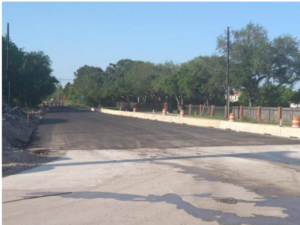
Asphalt paving at O'Day Rd., looking south.
