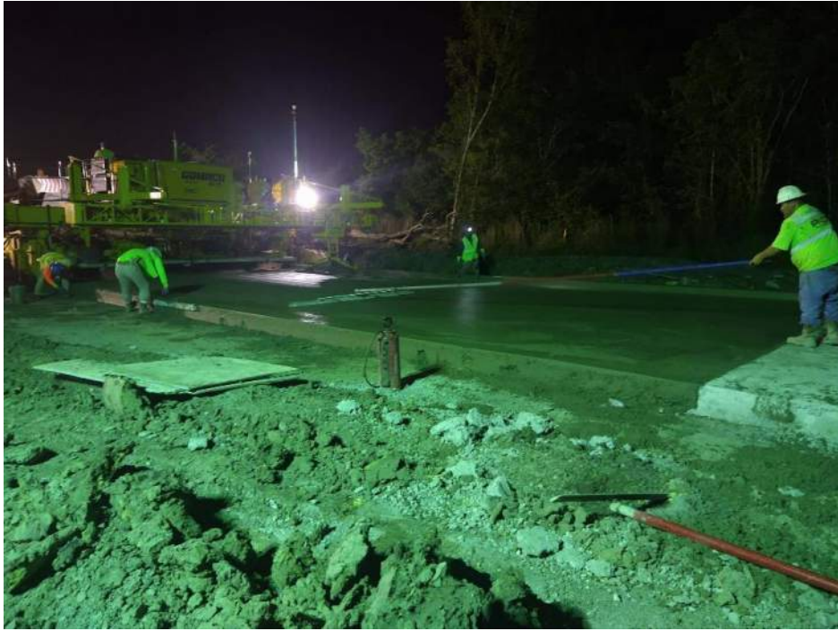
McHard Rd. night pour between O'Day Rd. and Garden Rd.
