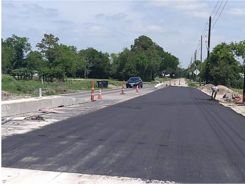
Asphalt paving on Stone Rd.
