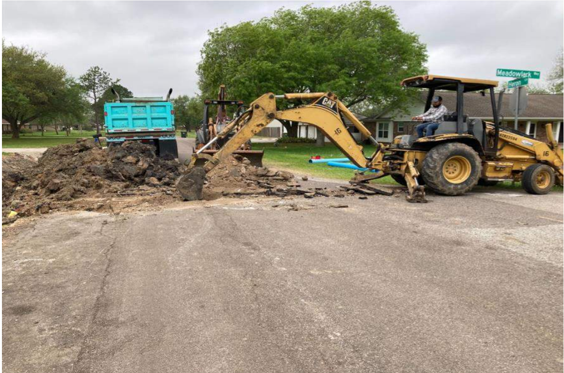
Waterline crossing at Meadowlark and Heron Way
