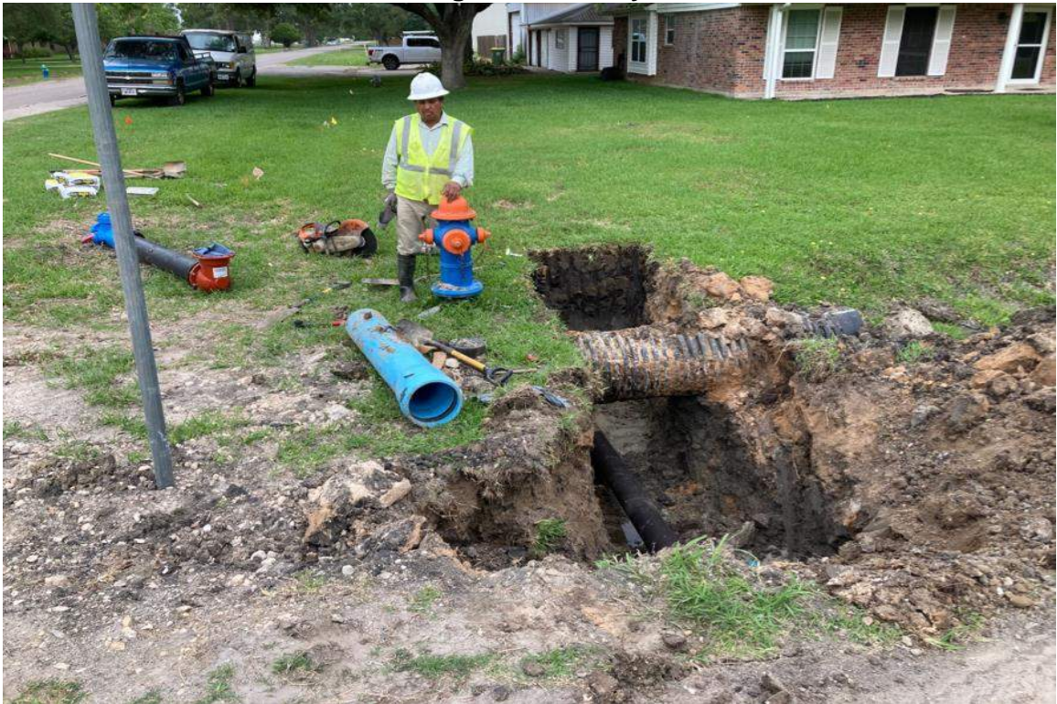
Installing Fire Hydrant on Heron Lane
