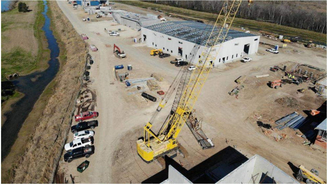
Membrane Bldg from southeast looking north west
