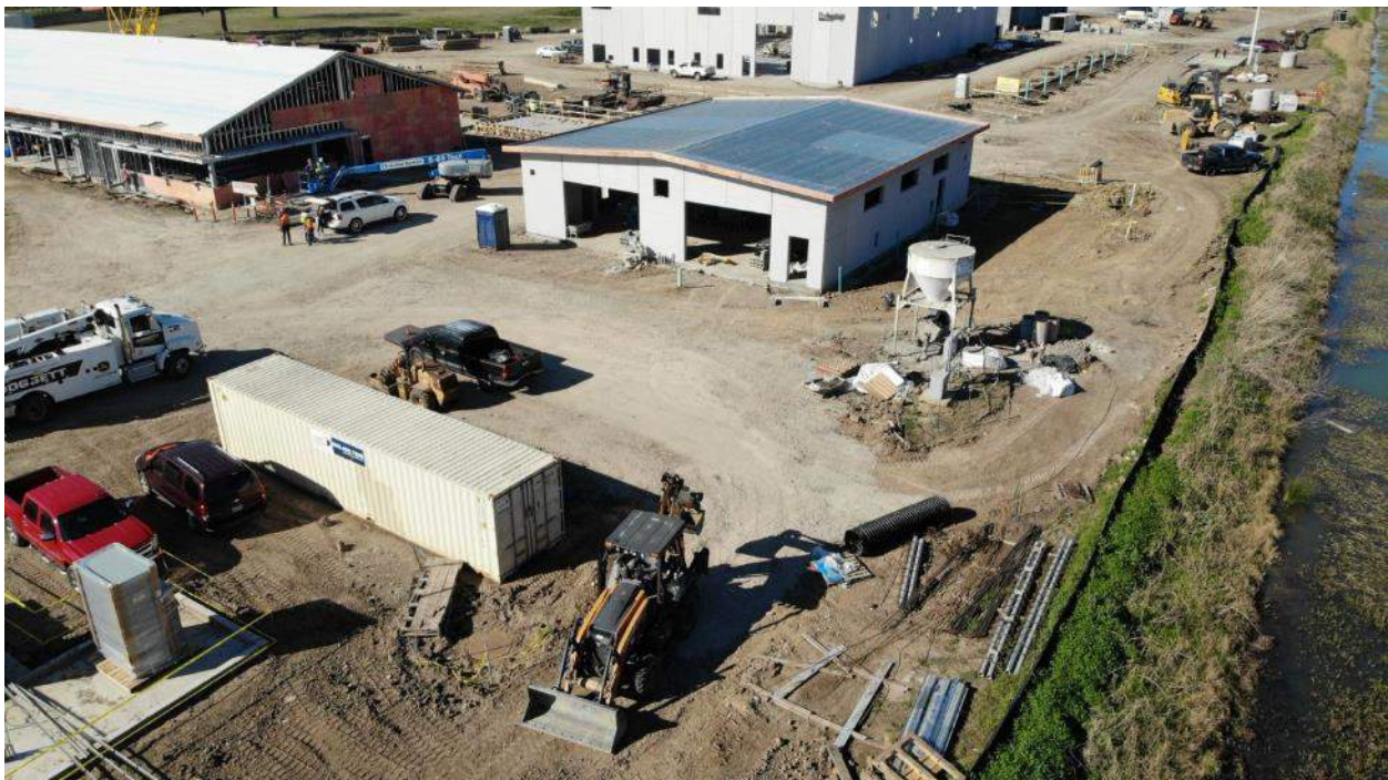
Maintenance Building East looking west with Operations Building to the left and Membrane in the background
