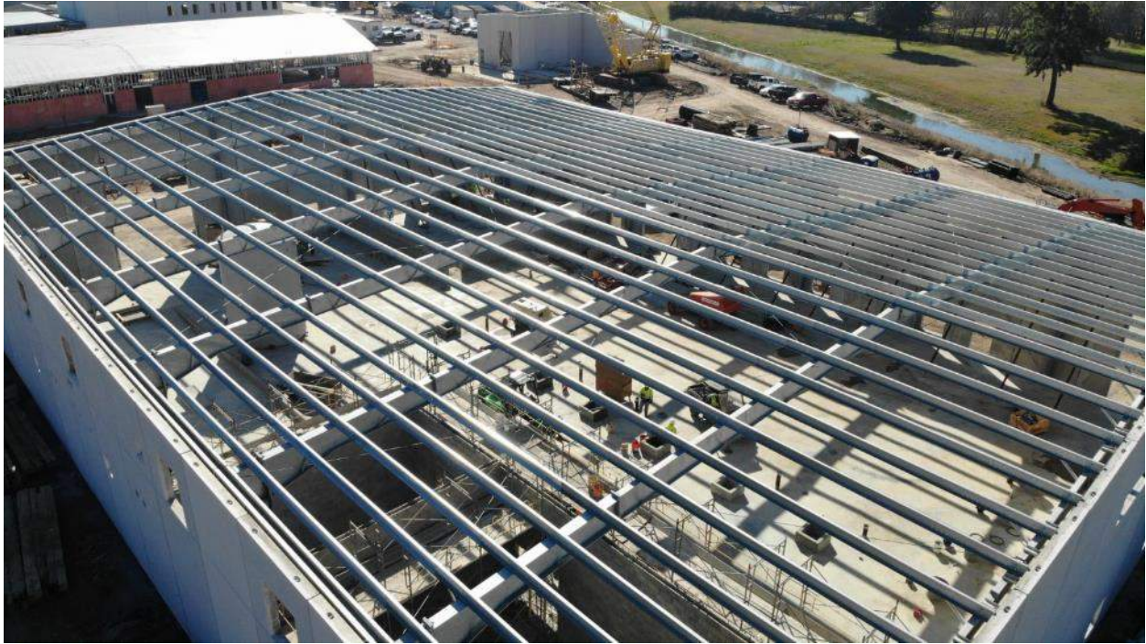
Top down view into the interior of the Membrane Bldg showing the early installation of process equipment and status of work on Electrical Room buildout.
