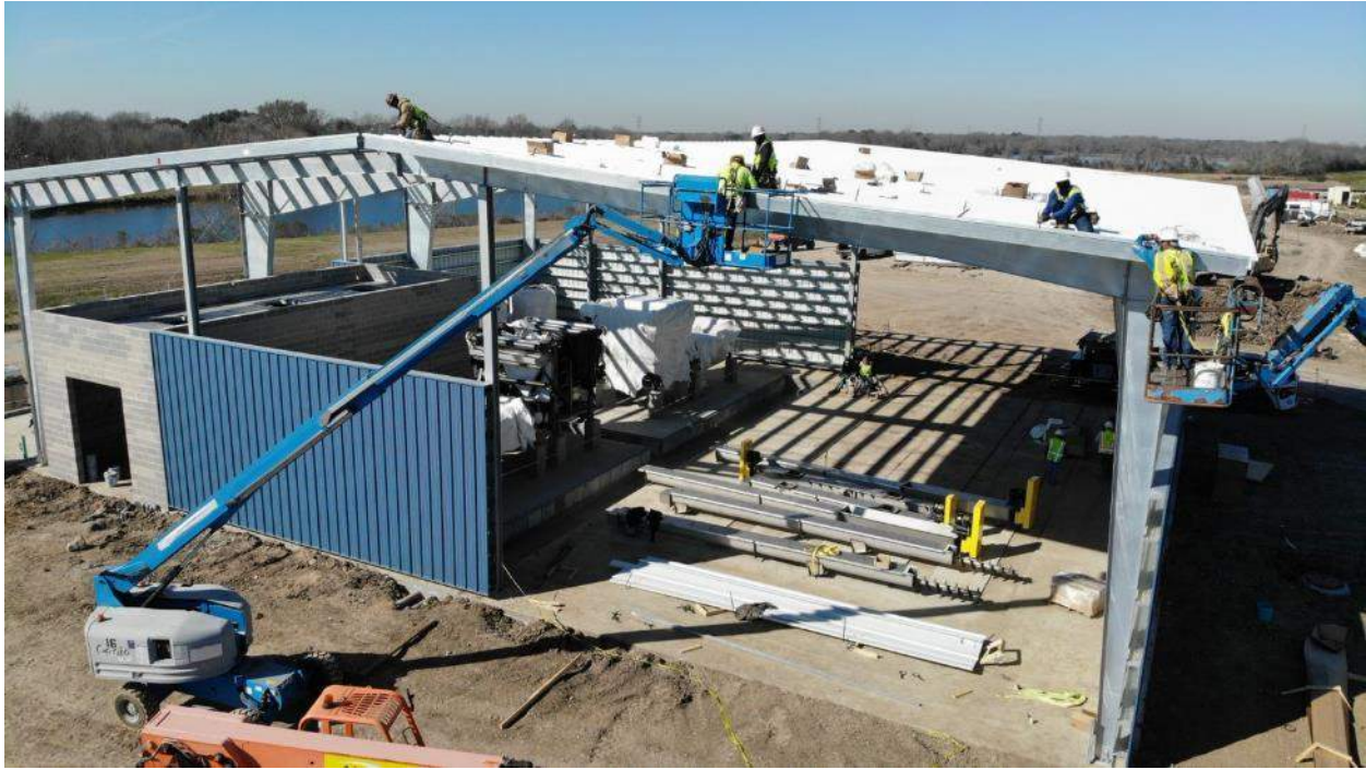
Solids Handling building showing installation of Belt Presses.
