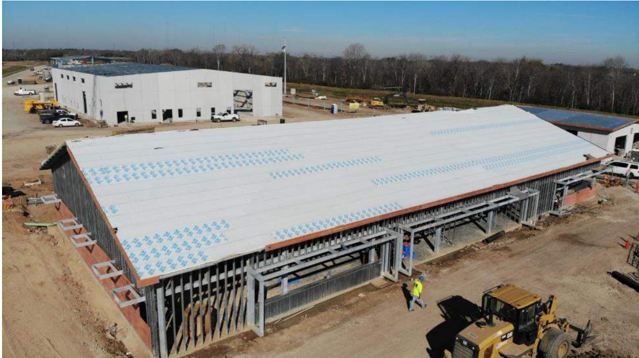
Front of Operations Building with Membrane Bldg in background
