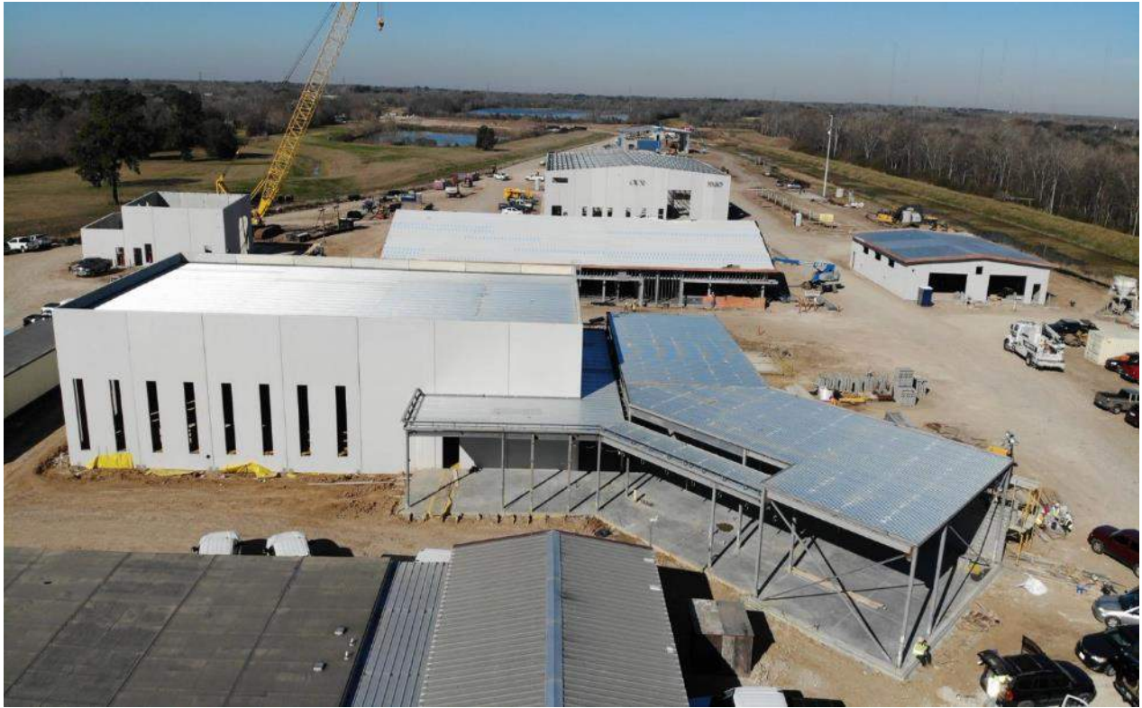
Front side of Administration (right) and High Service Pump building (left)
