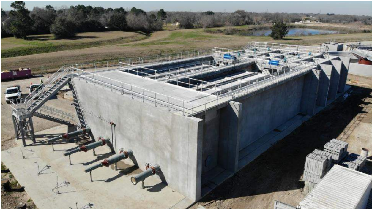
Aerial view of the east end of Pre-Treatment basin showing settled water suction piping and pump foundation pads.
