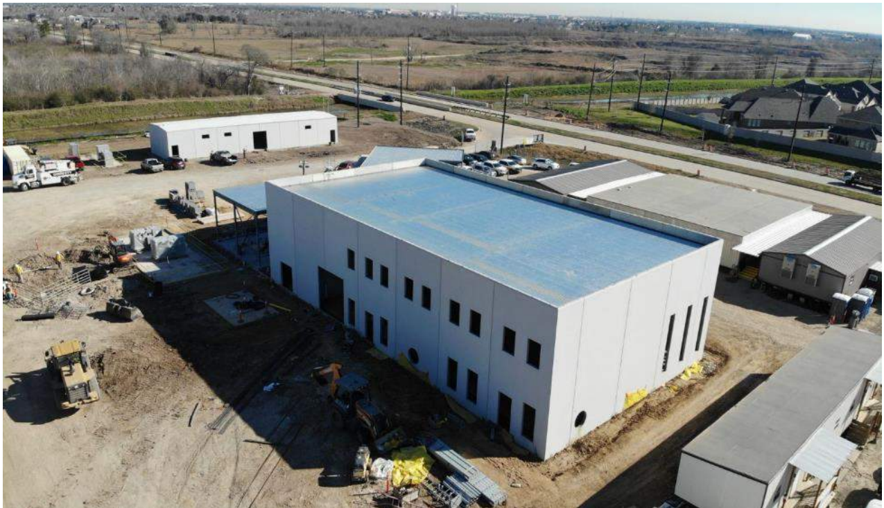
Back side of High Service Pump Building looking North East
