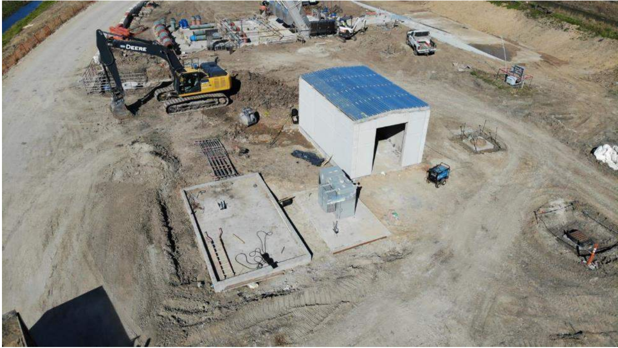
Raw Water Electrical Building and Generator foundation.
