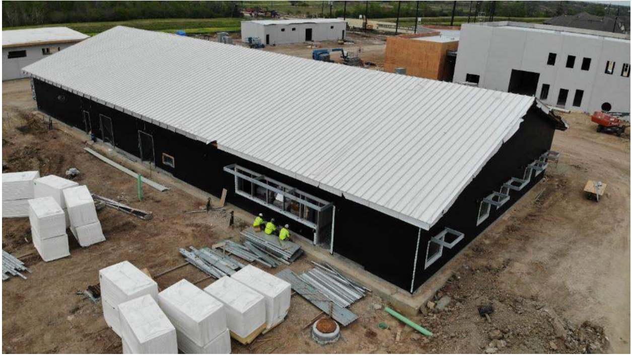
Overhead of Operations Bldg.
