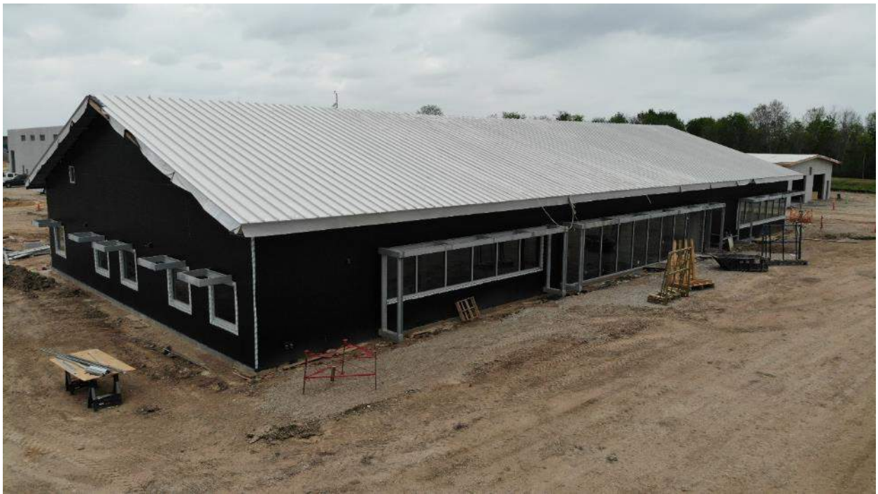
Back side, (west) of Operations Bldg.
