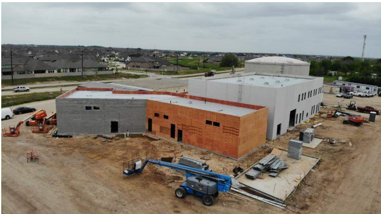
North side of Administration Bldg. with High Service in background
