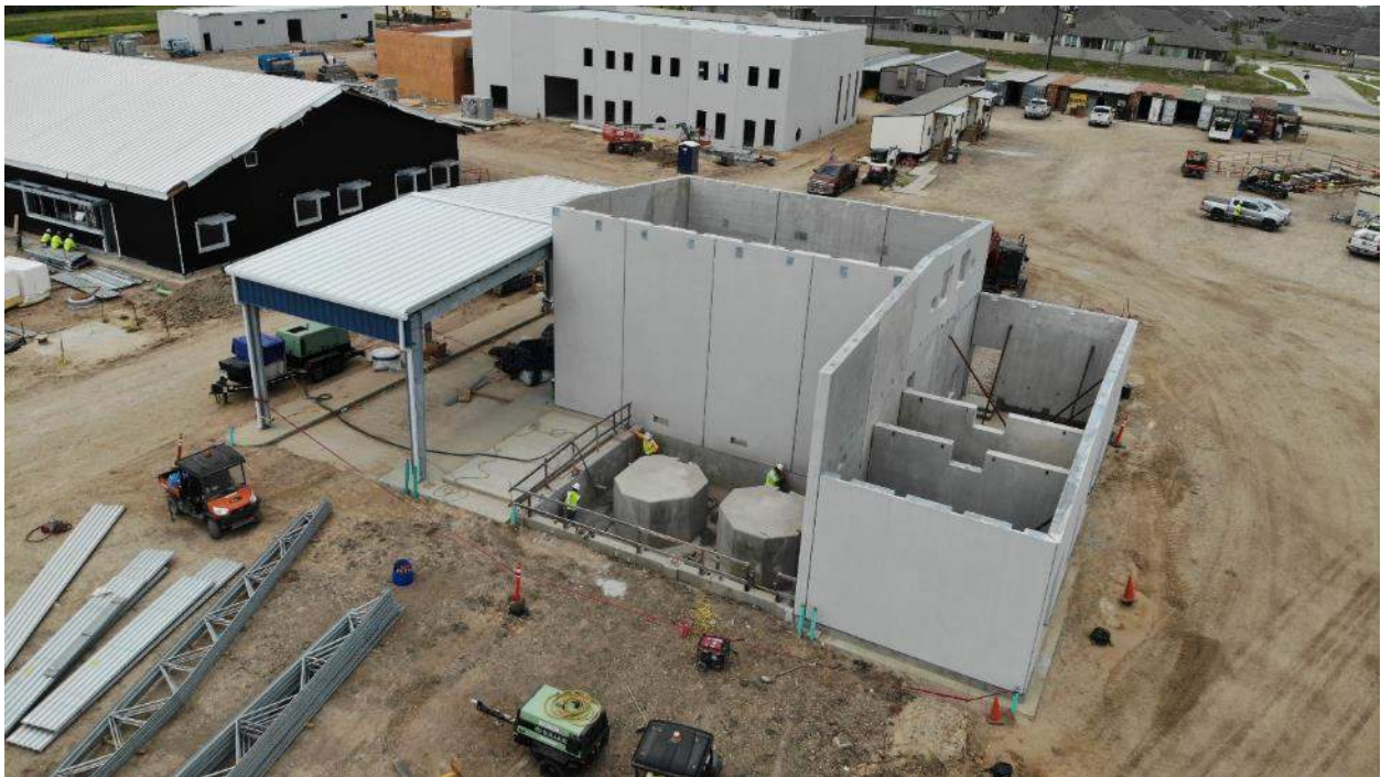
Backside of Chlorine DiOxide Bldg., note roofing materials in foreground
