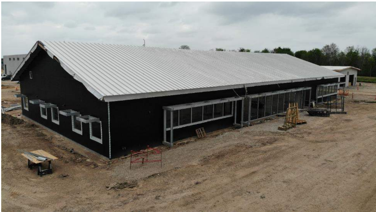
Back side, (west) of Operations Bldg.
