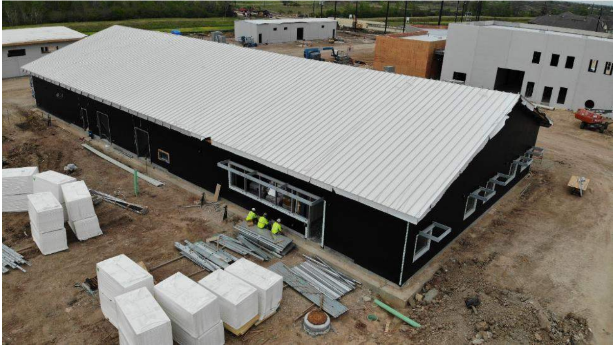
Overhead of Operations Bldg.
