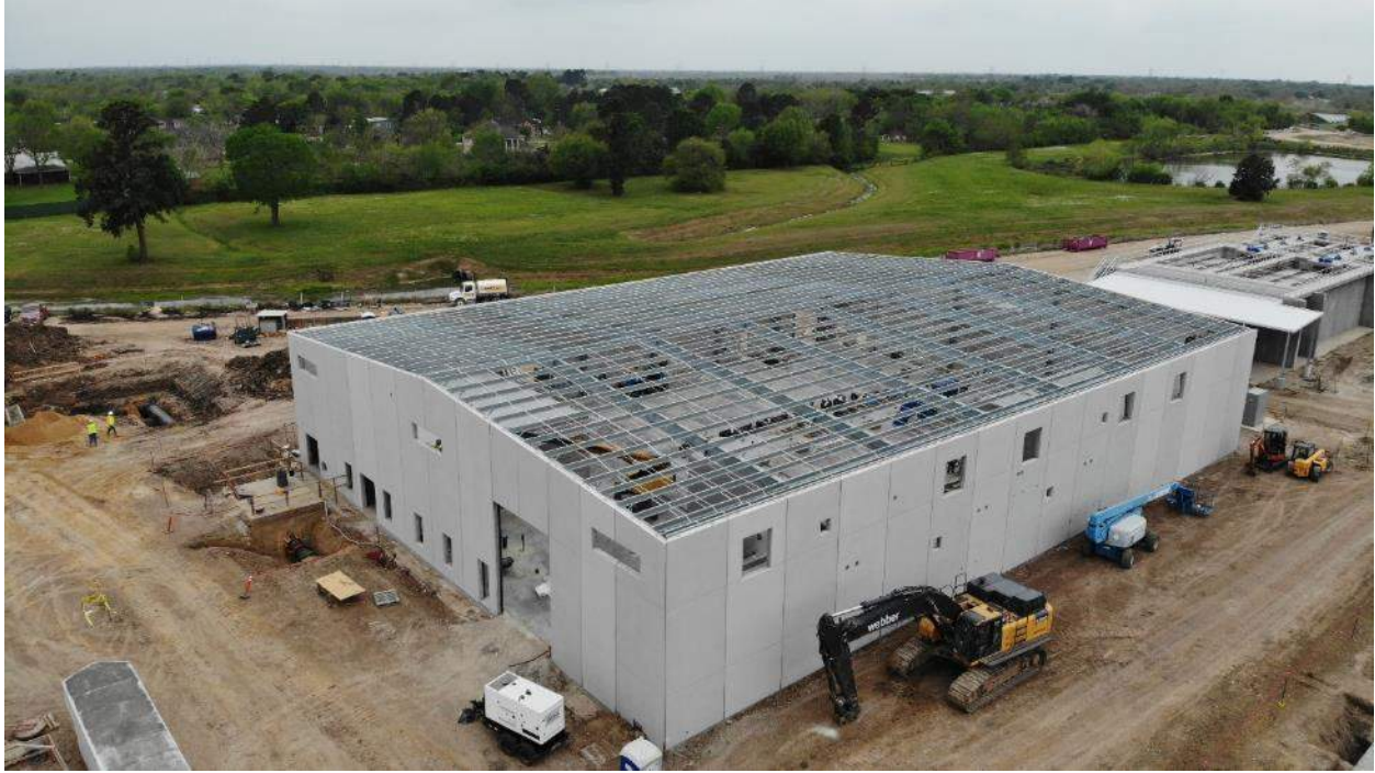
Membrane Bldg., preparing to begin receiving Membrane equipment
