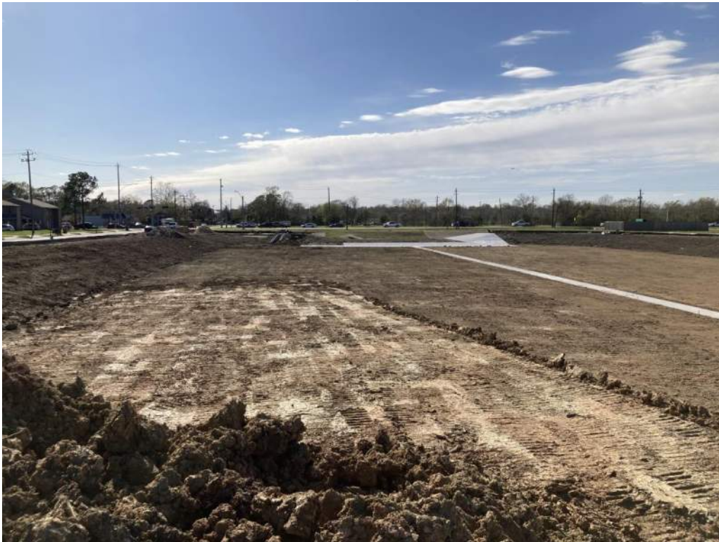
Continuing Excavation of Willowcrest Pond
