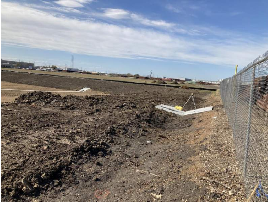
Willowcrest Backslope Drain East End
