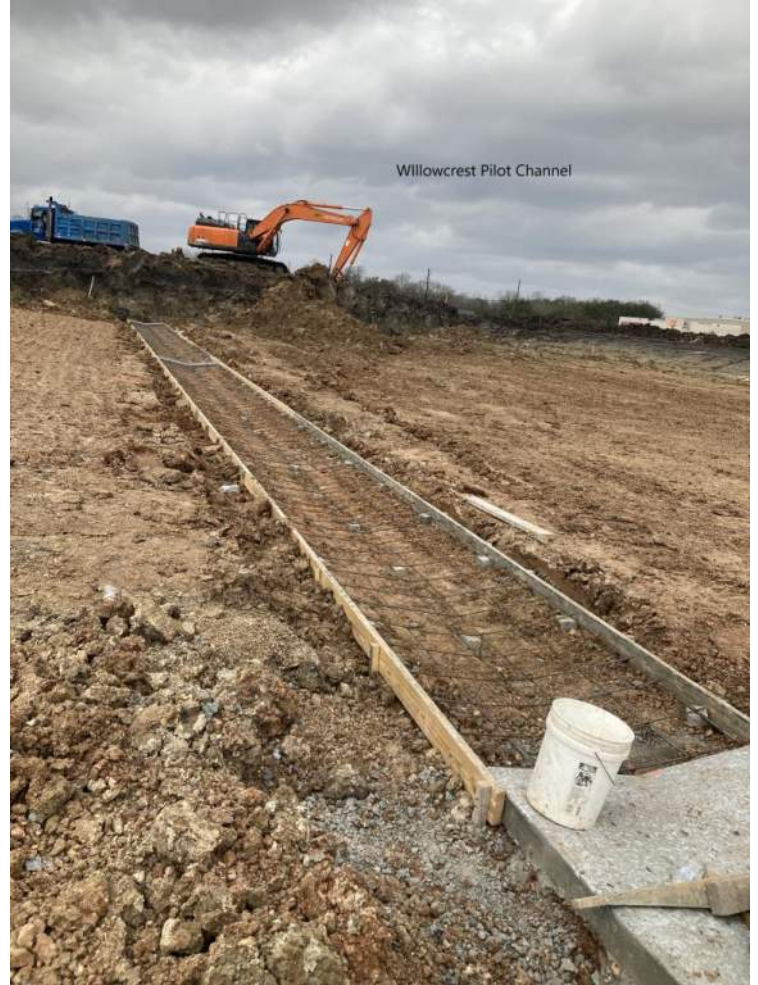
Forms and Steel for Pilot Channel
