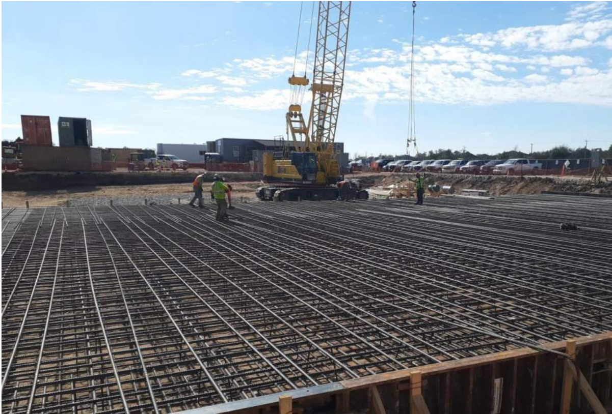
Preparing to pour slab at SBR 5 and 6
