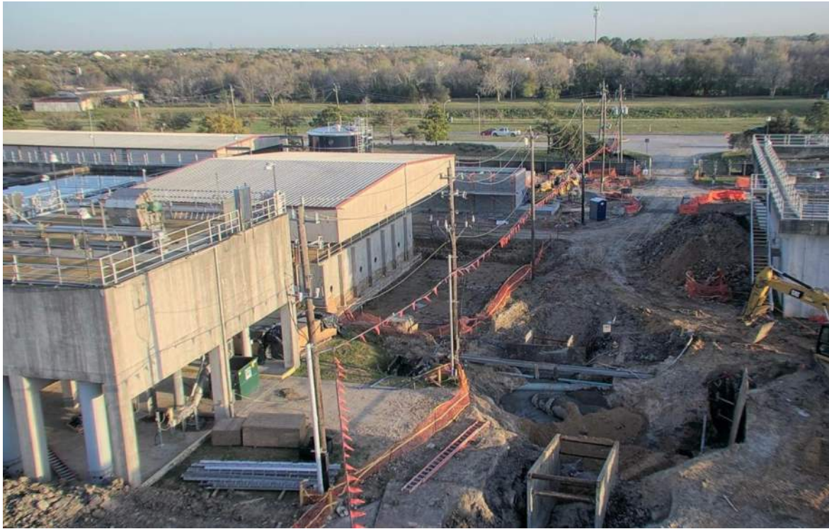
Duct Bank Installation at Plant Entrance
