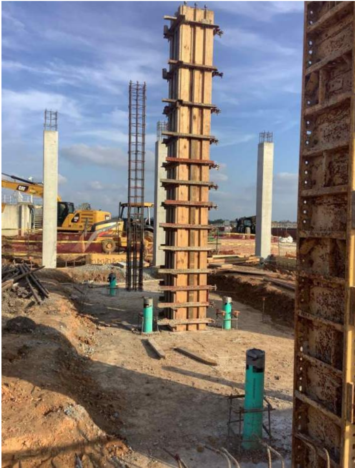
Columns for Sludge Building
