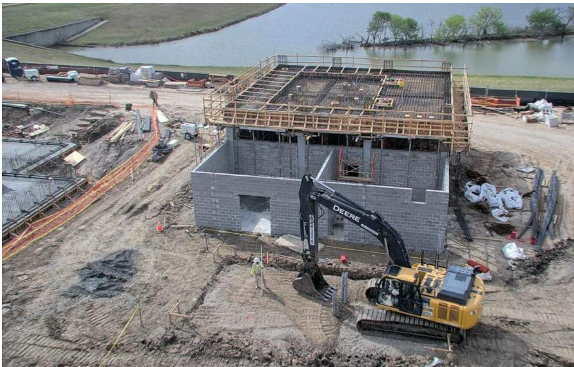
Elevated Deck Scaffolding, Formwork, and Reinforcement at the Sludge Building
