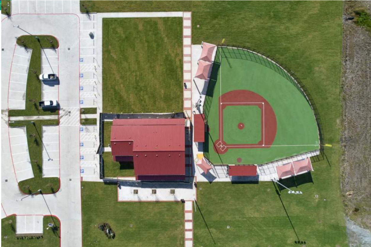
Aerial of Miracle Field, Concession building and added parking lot
