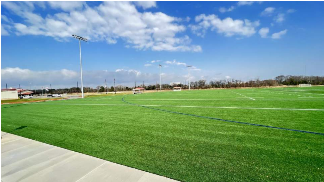
North facing view of synthetic turf multi-purpose fields
