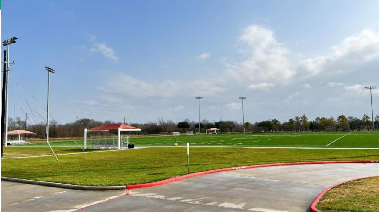
East facing view of multi-purpose fields, with new field lighting and covered spectator bleachers
