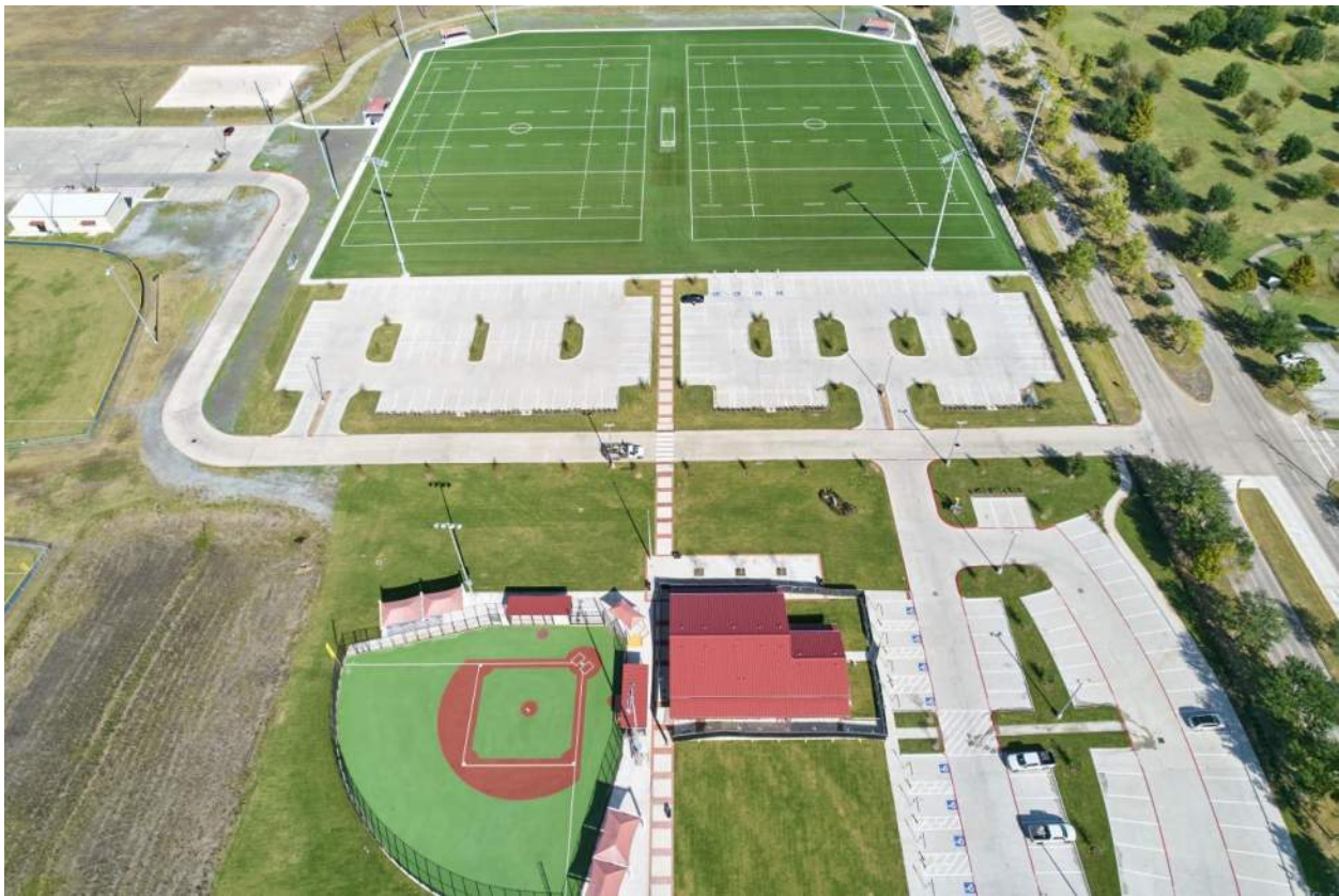
Aerial view of improvements completed at the Sports Complex
