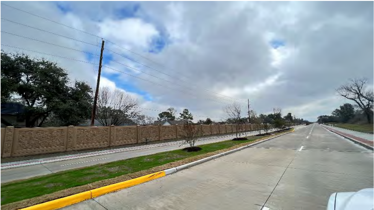
Completed landscaped median
