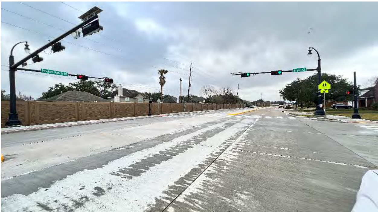
Bryan Court intersection and signal
