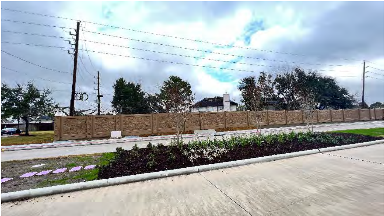
Completed Sound Wall
