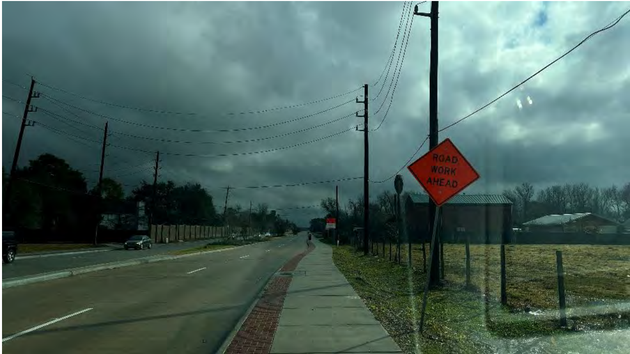
Sidewalk construction along south side looking east
