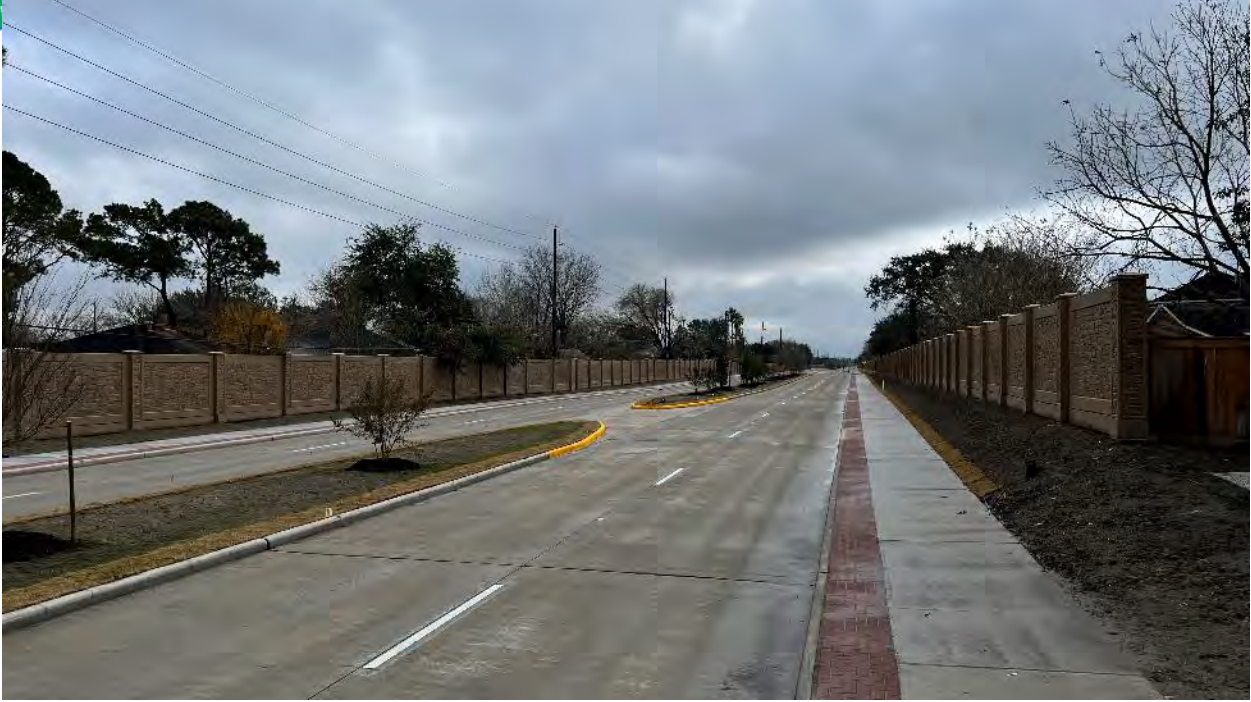
Full view of corridor improvements
