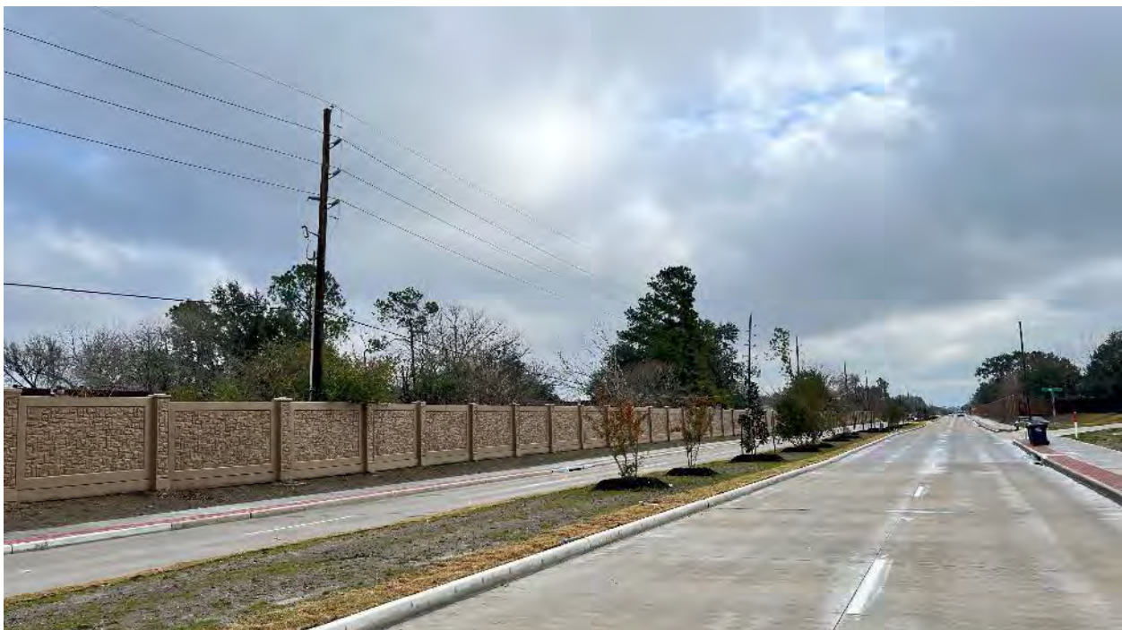
Roadway, sidewalk, median and sound wall completion
