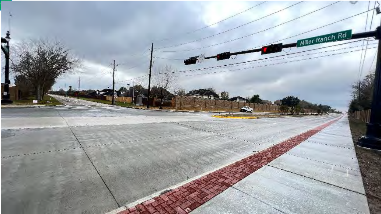
Miller Ranch intersection and signal
