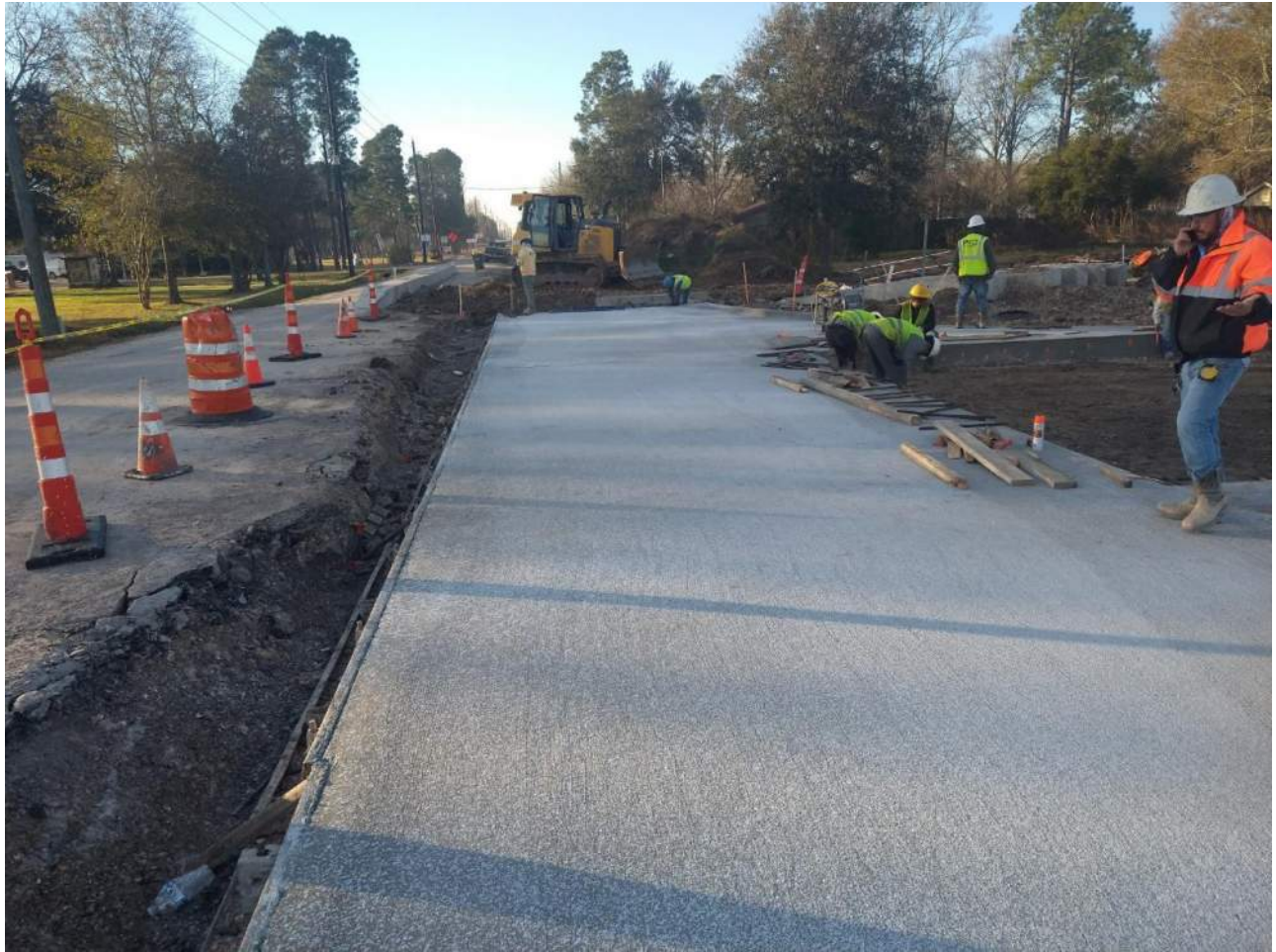
Concrete paving operations at Stone Rd.
