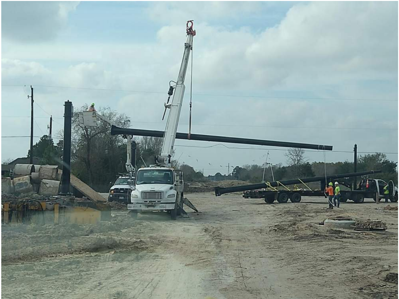
Traffic signal installation at O'Day Rd.
