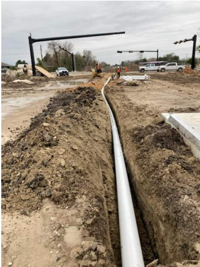
Irrigation system installation between Hatfield Rd. and Mykawa Rd.
