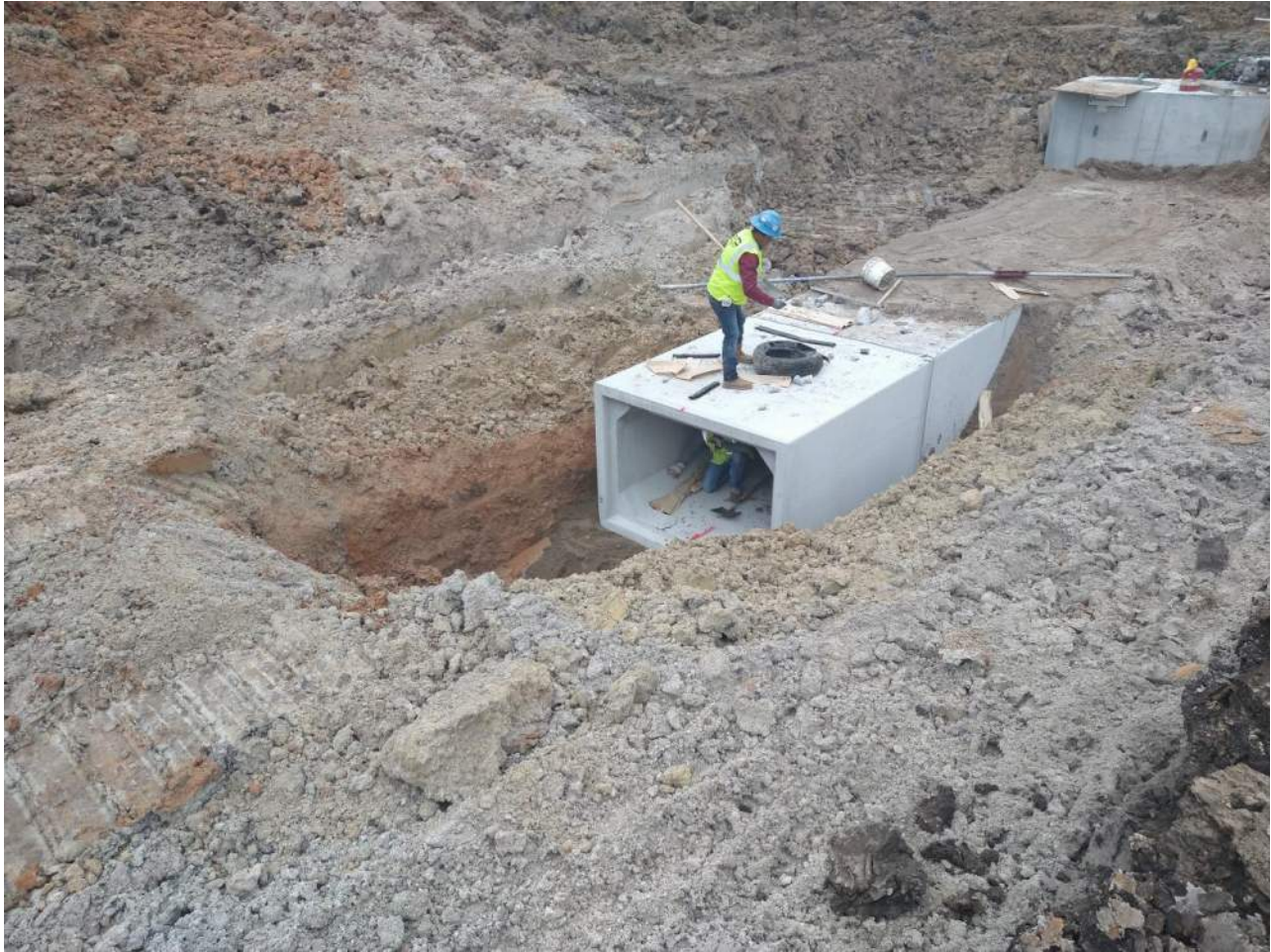
Installation of 7 x 3 boxes between Stone Rd. and Max Rd.
