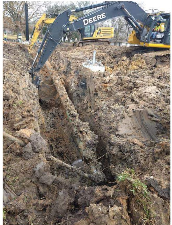
Existing waterline relocation
