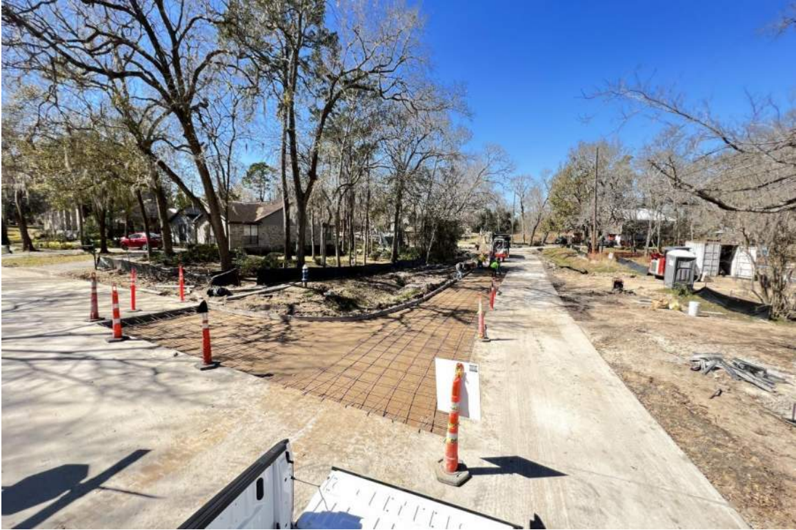
Sleepy Hollow Dr. and Rip Van Winkle Dr. Steel Being Tied
