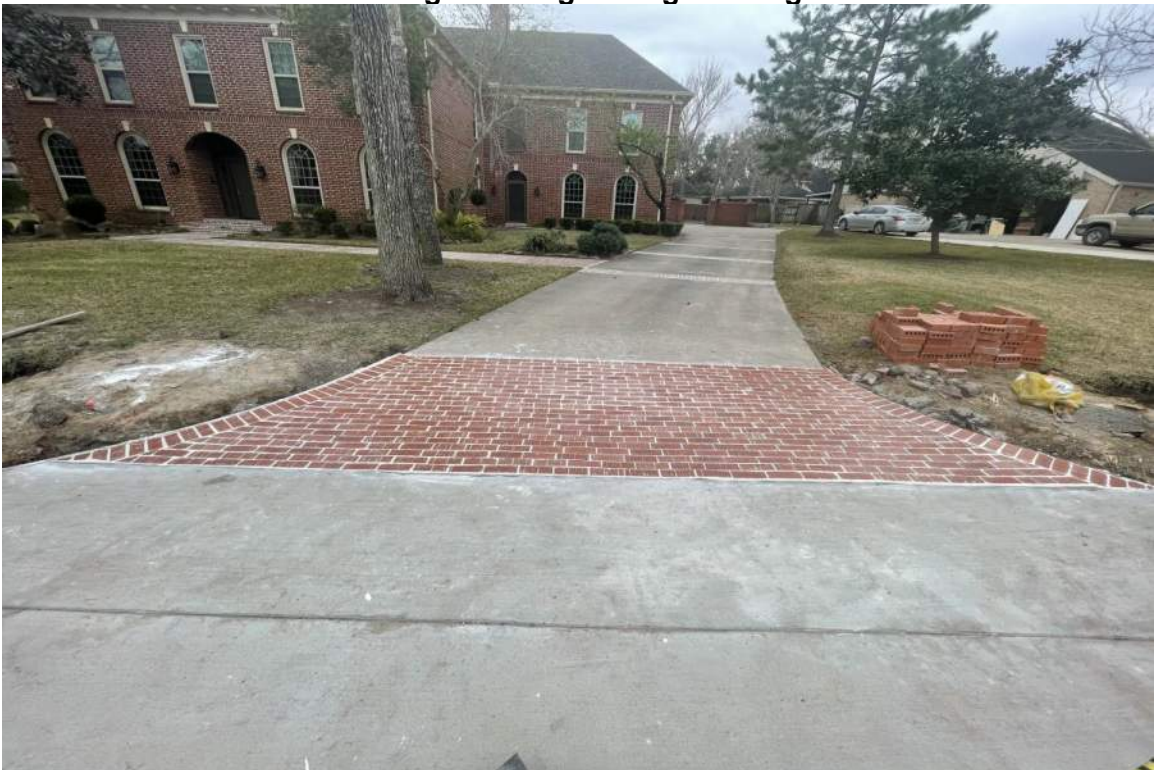
Decorative Drive and Culverts have Been Replaced
