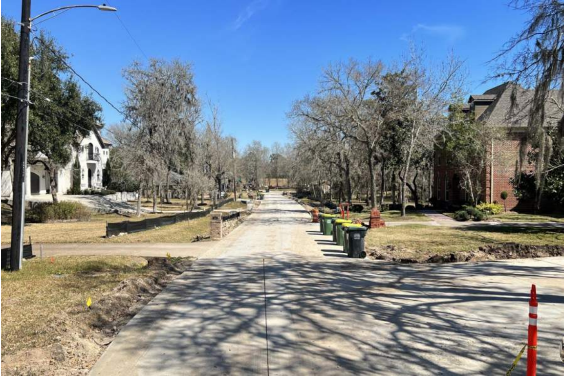
Sleepy Hollow Dr. Pavement Poured
