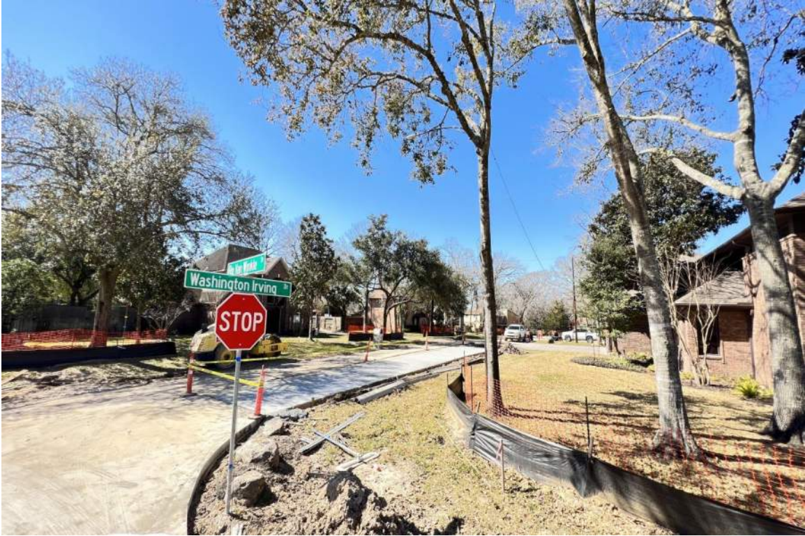
Washington Irving Paving has Begun
