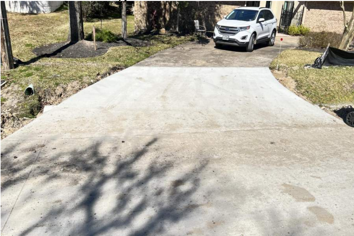
Culverts Installed and Driveway Poured Back
