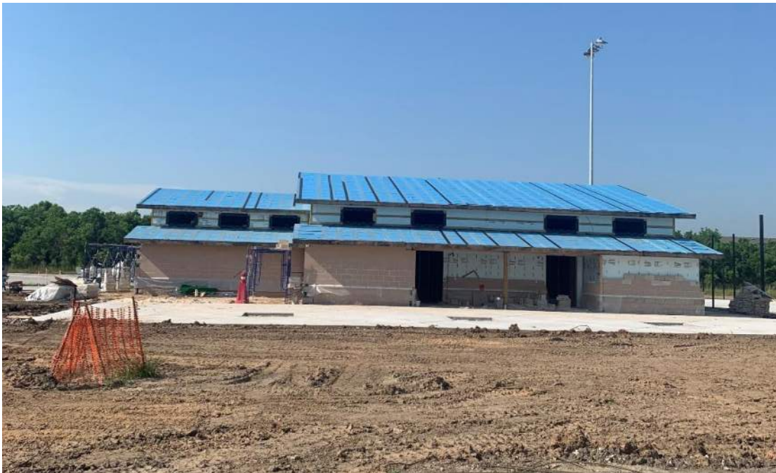
Concession Building (Team rooms entrance)
