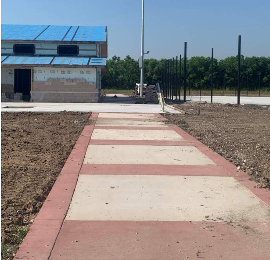
Integral color concrete sidewalk between Concession Building and Miracle Field
