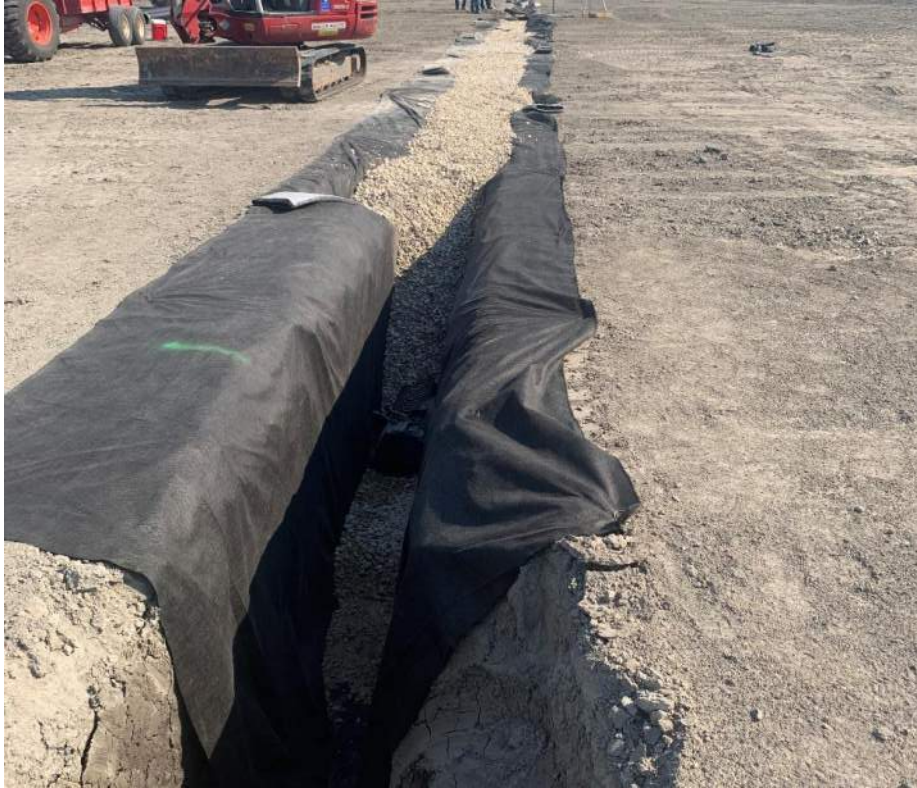
French Drain installation in-progress Between Multi-Purpose fields
