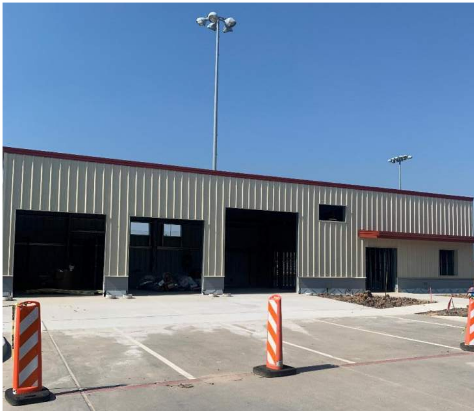
Maintenance Building with new Driveways
