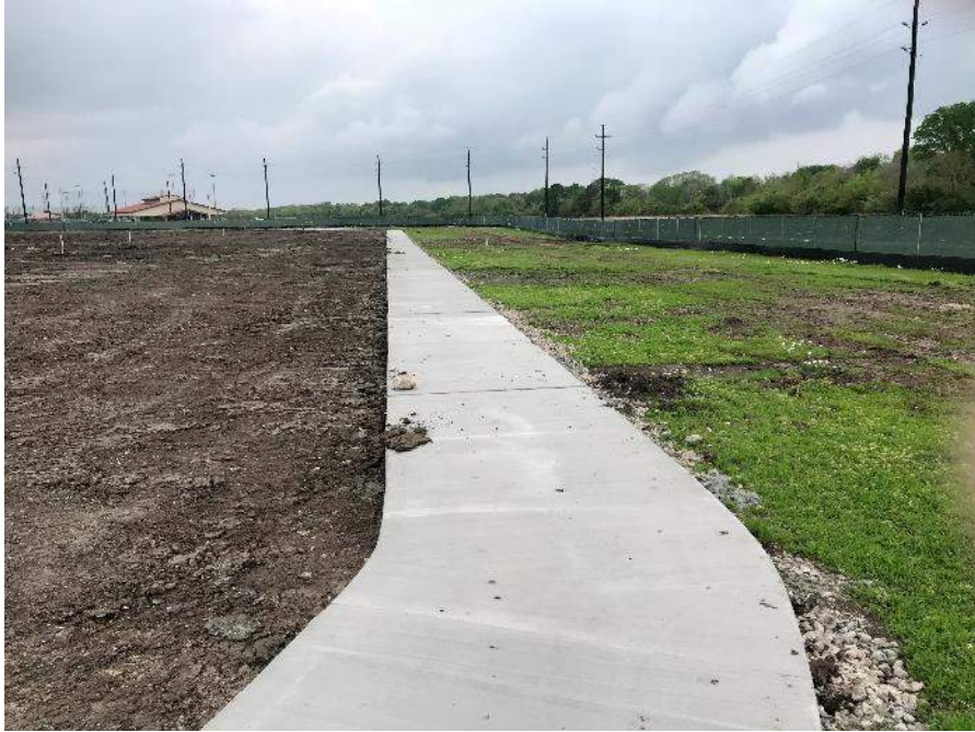
Sidewalk Installation around the Multipurpose Field Perimeter.
