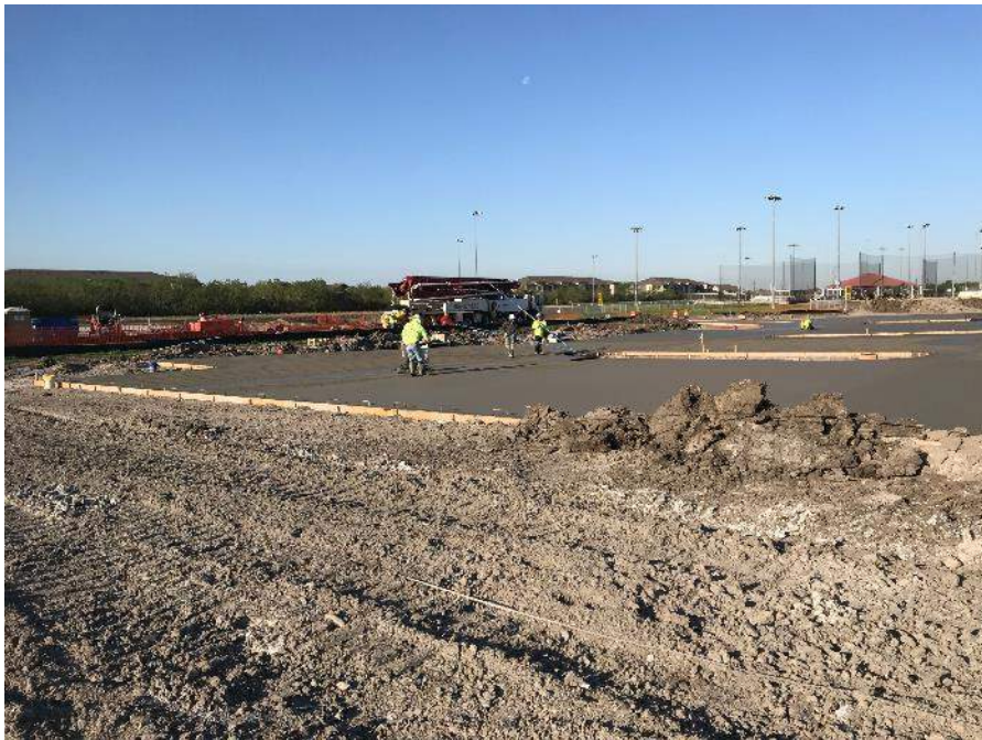
Concrete Placement for the NE and NW Parking Lots
