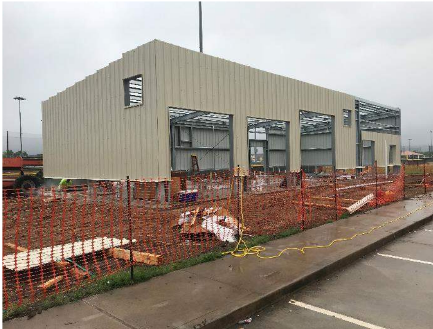
Construction of Maintenance Building.
