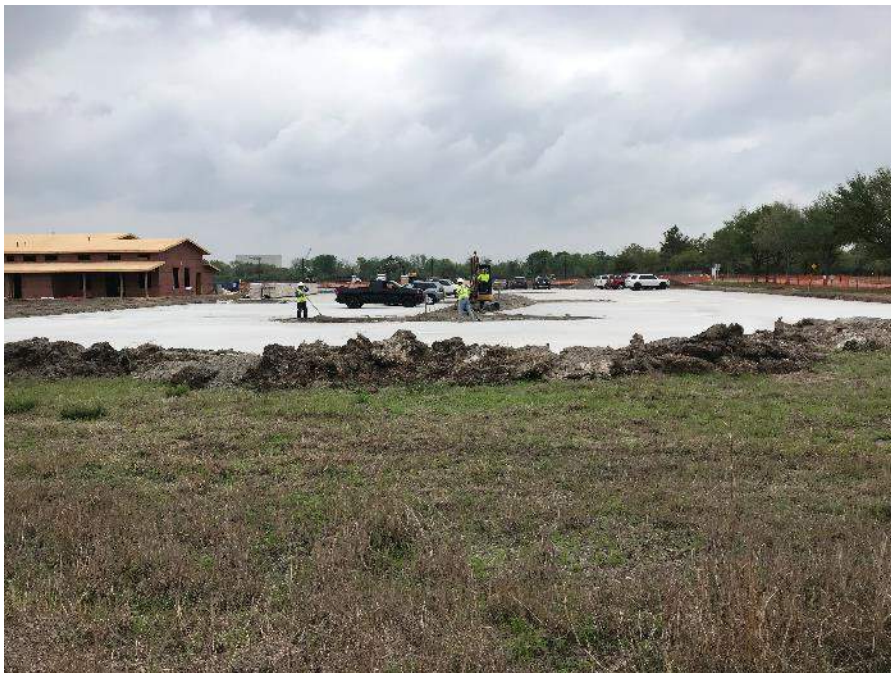
Concrete Placement for South Parking Lot Complete
