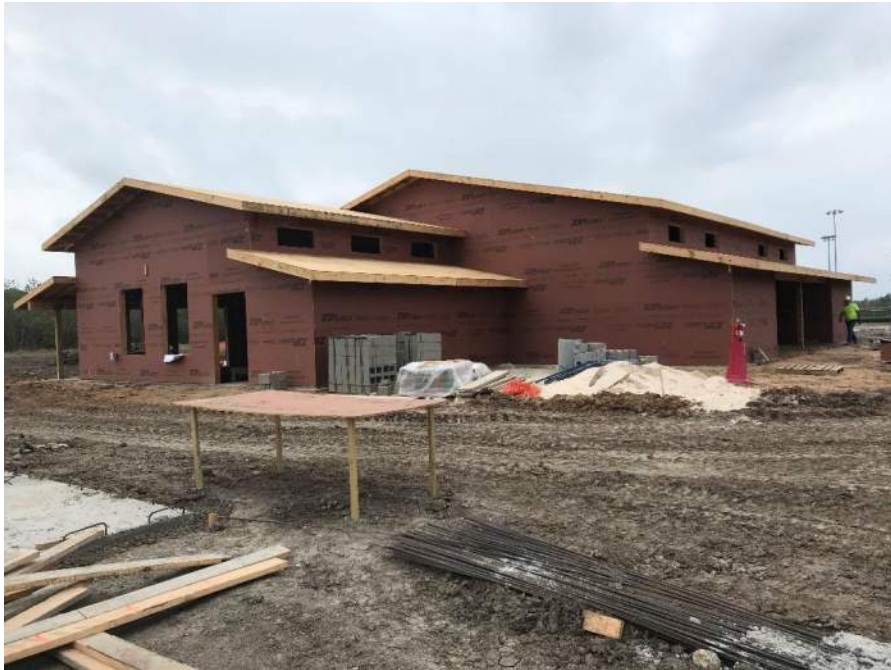
Wood Light-Framing and Sheathing for the Concession Stand.
