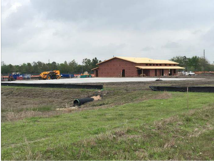
Concrete Slab-On-Grade for the Miracle Field.
