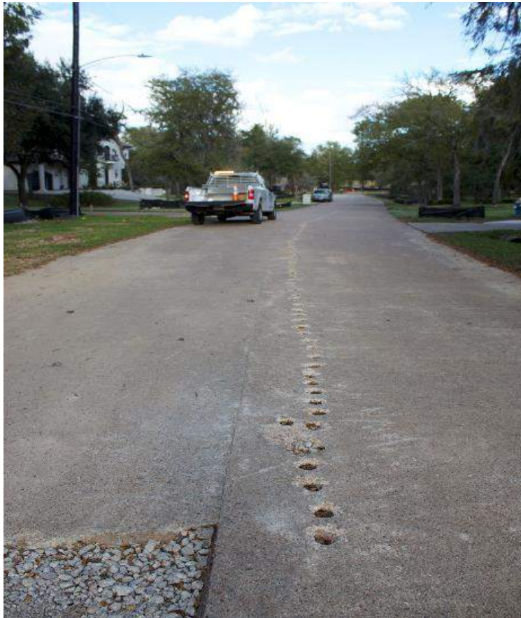
Road Is Being Prepped to Demo One Side at A Time
