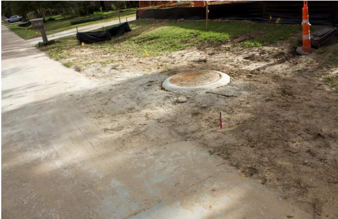
SWPP Protection is in Place and Manholes Have Been Set
