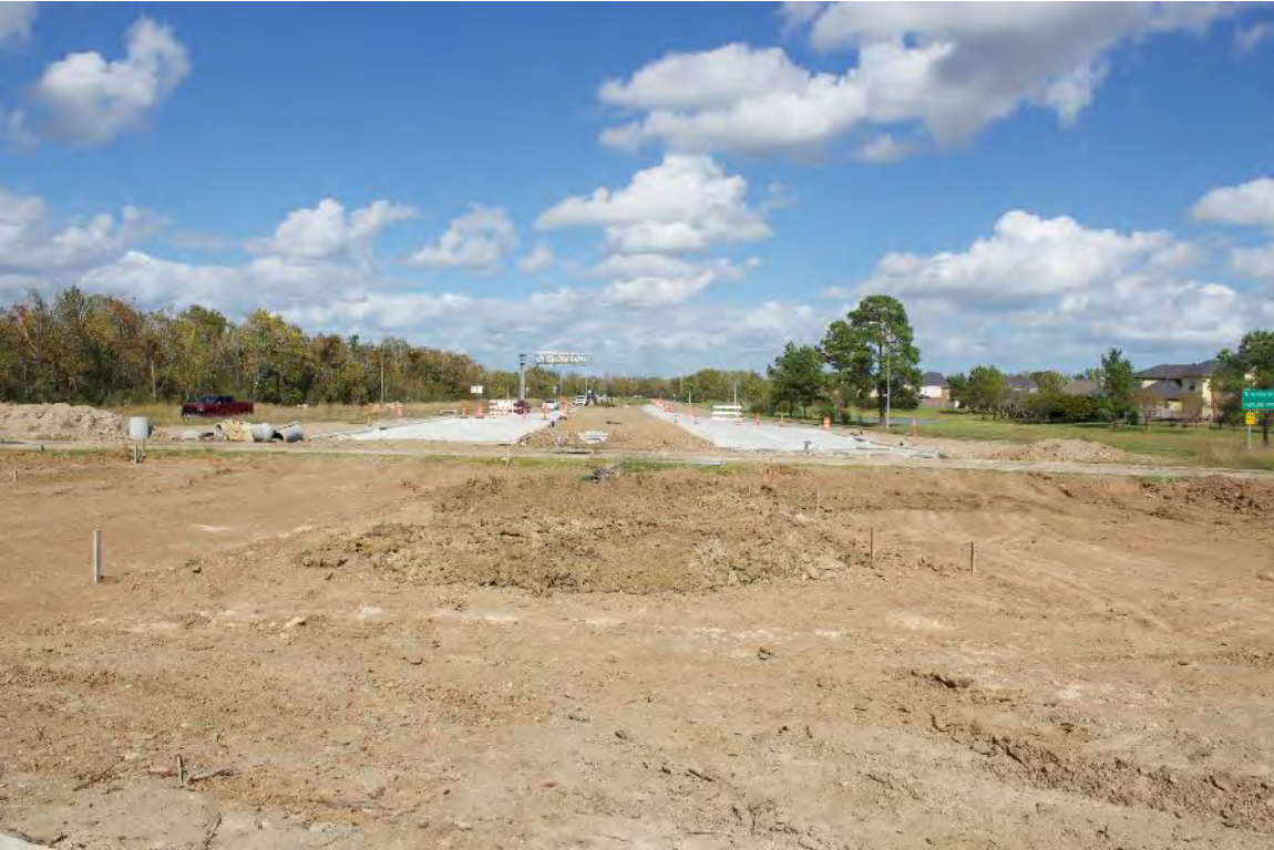
Northern Roundabout Entrance and Exit Have Been Poured
