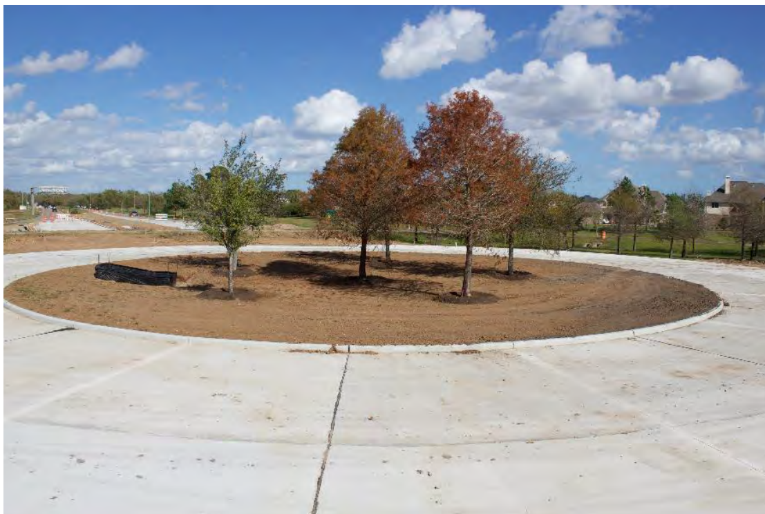
Trees have been Relocated
