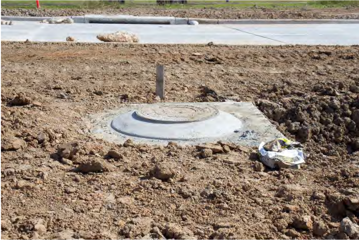
Manholes Have Been Set in Place
