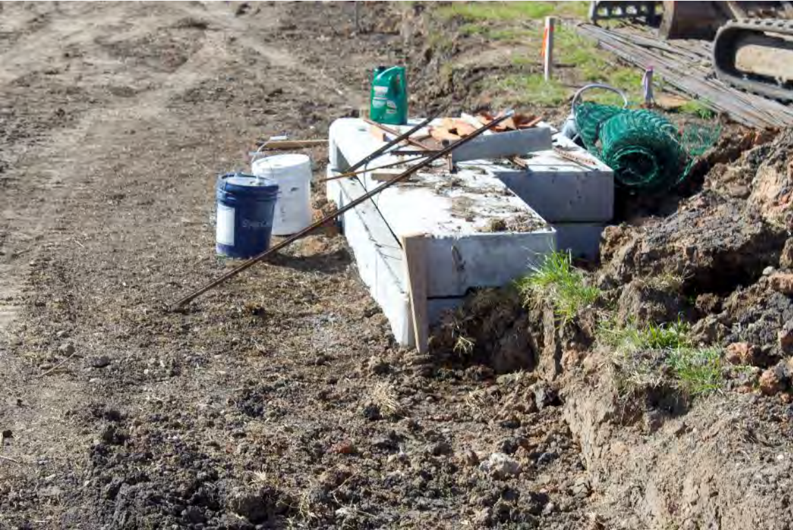
Storm Sewer Inlets Have Been Installed
