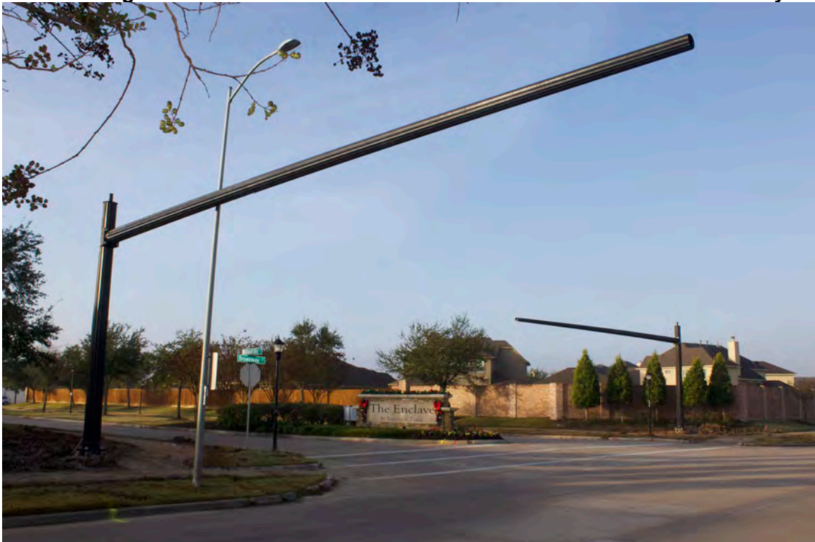
Traffic Signal Masts have been Installed at Windward Bay and Broadway
