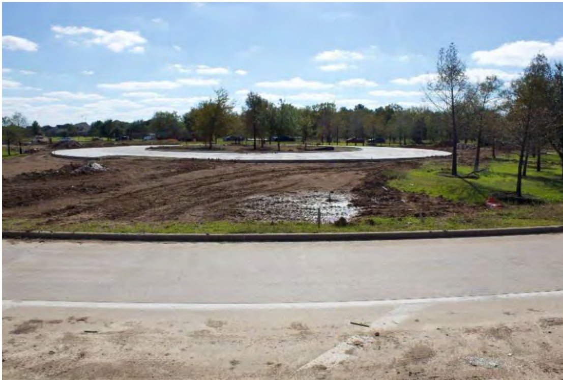
Central Roundabout Has Been Poured
