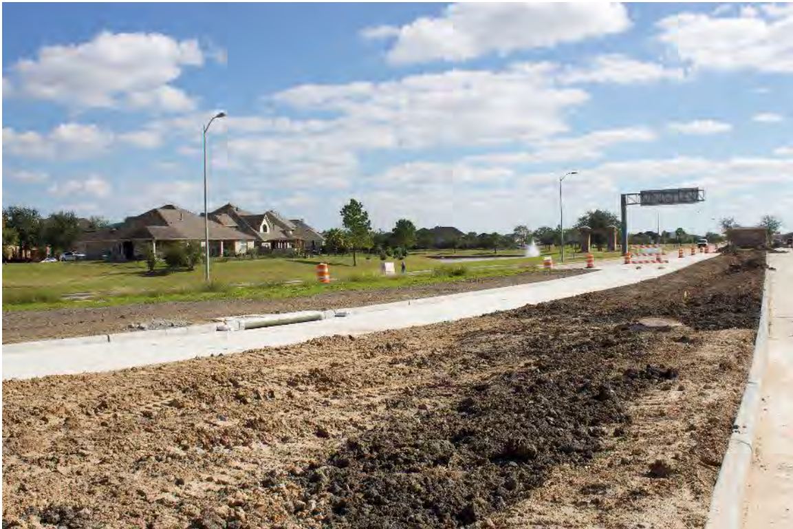
Grading in Medians is Being Brought to Proper Elevation
