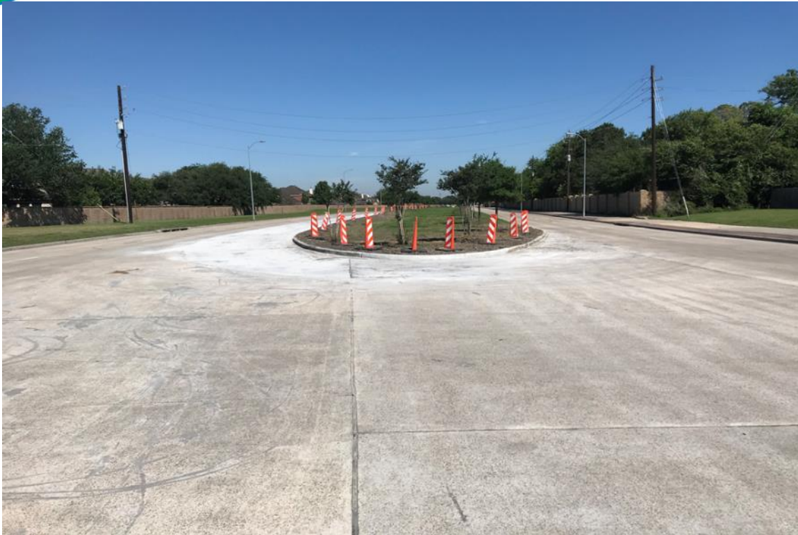
Left Turn Bay at Pearland Parkway and Oakridge Dr. (Facing North)
