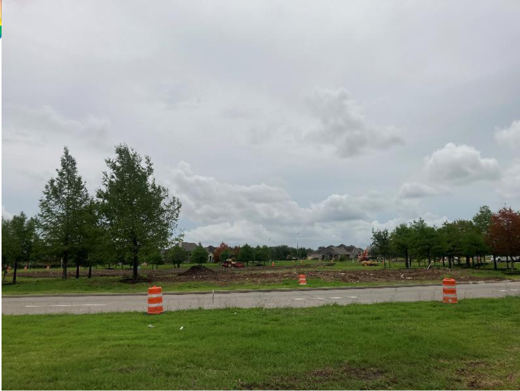
Construction of Traffic Circle is Underway
