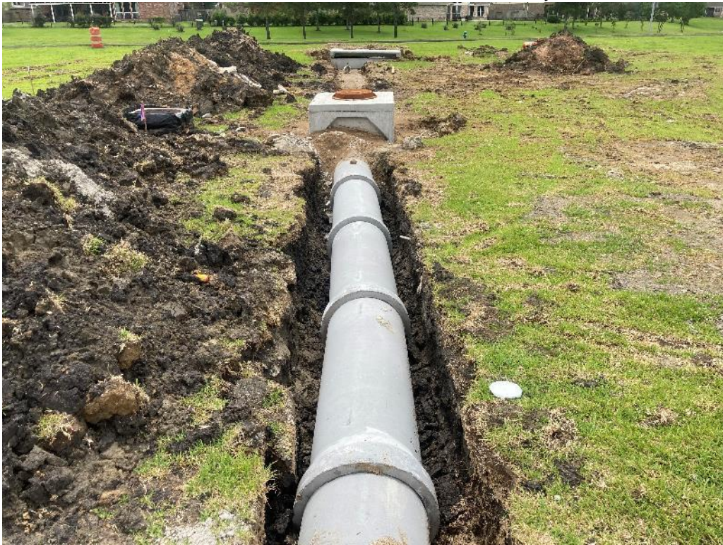
Storm Sewer Being Installed in Traffic Circle
