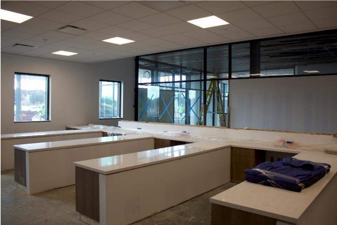
Millwork in Tax Office Has Been Installed.
