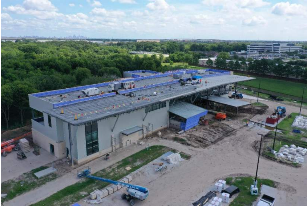
North Facing Aerial View
