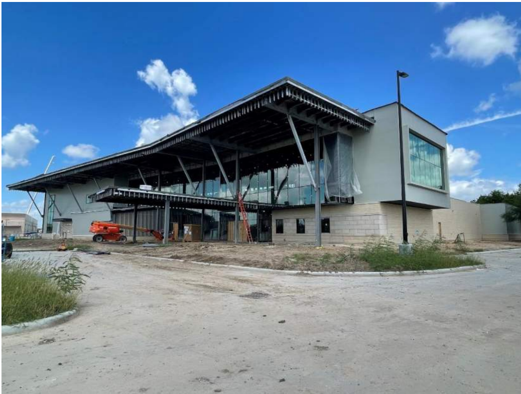
Front View of Library
