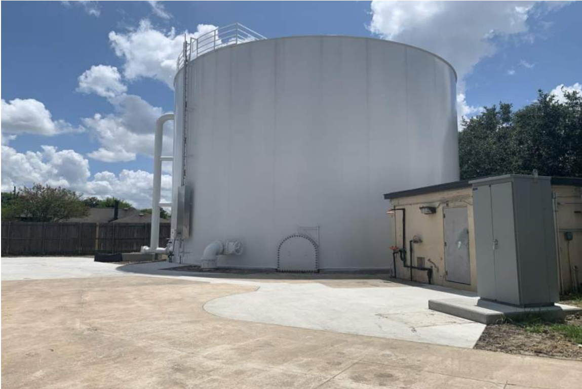
Ground Storage Tank Painted and Flatwork Poured Back
