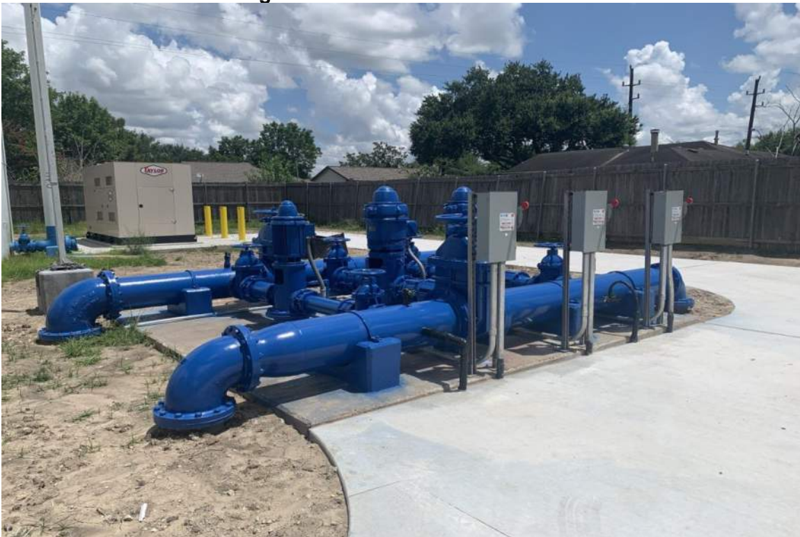
All Piping has been Painted and Pump Disconnects Replaced
