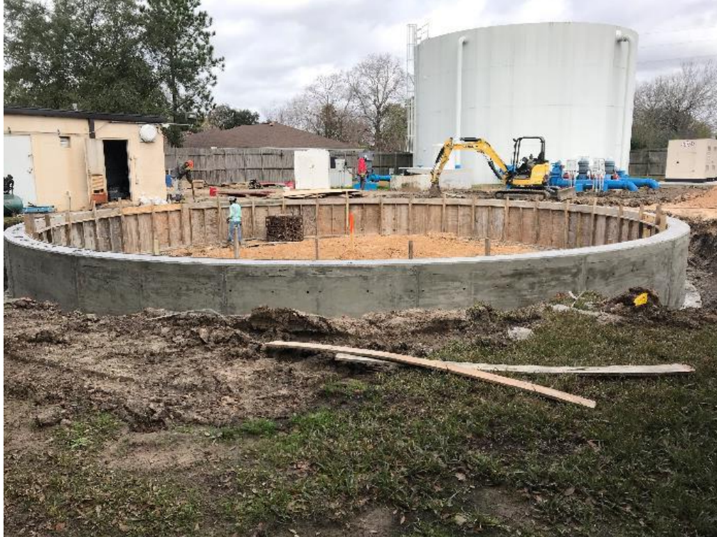
Contractor wrecking forms and applying finish to GST retainer ring foundation.
