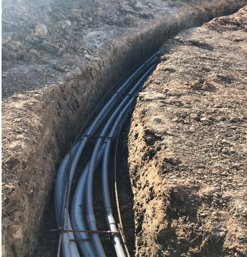
Reinforced duct bank run with 1.5", 3" and 1' (spare) conduit.
