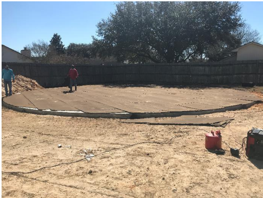
Contractor installing tank padding and waterproofing mastic on proposed GST
