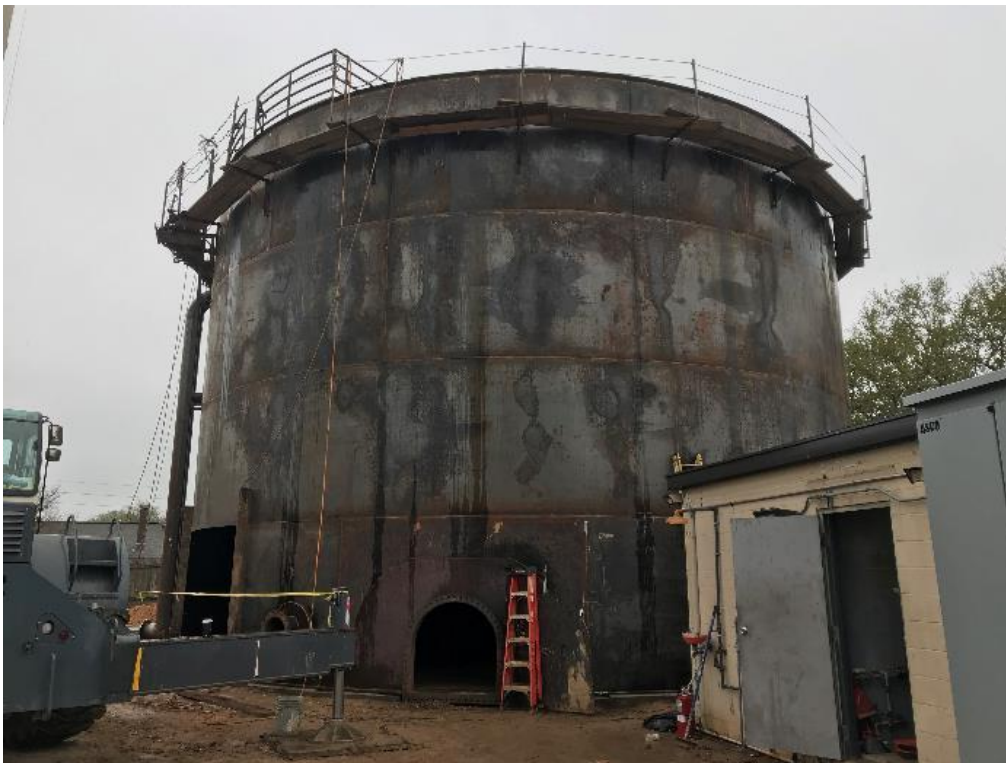
Construction of 400,000-gallon welded GST at Southdown Groundwater Plant
