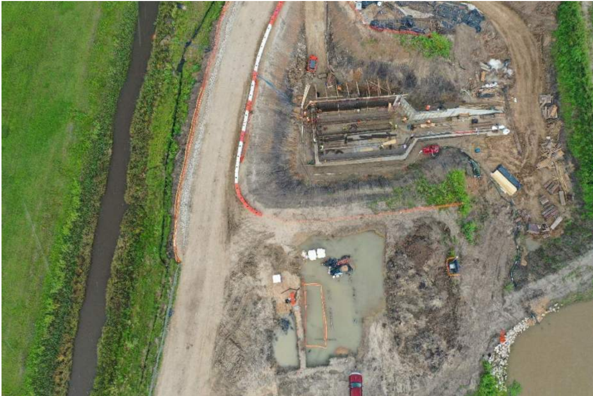
Raw Water Intake Channel & Pump Station
