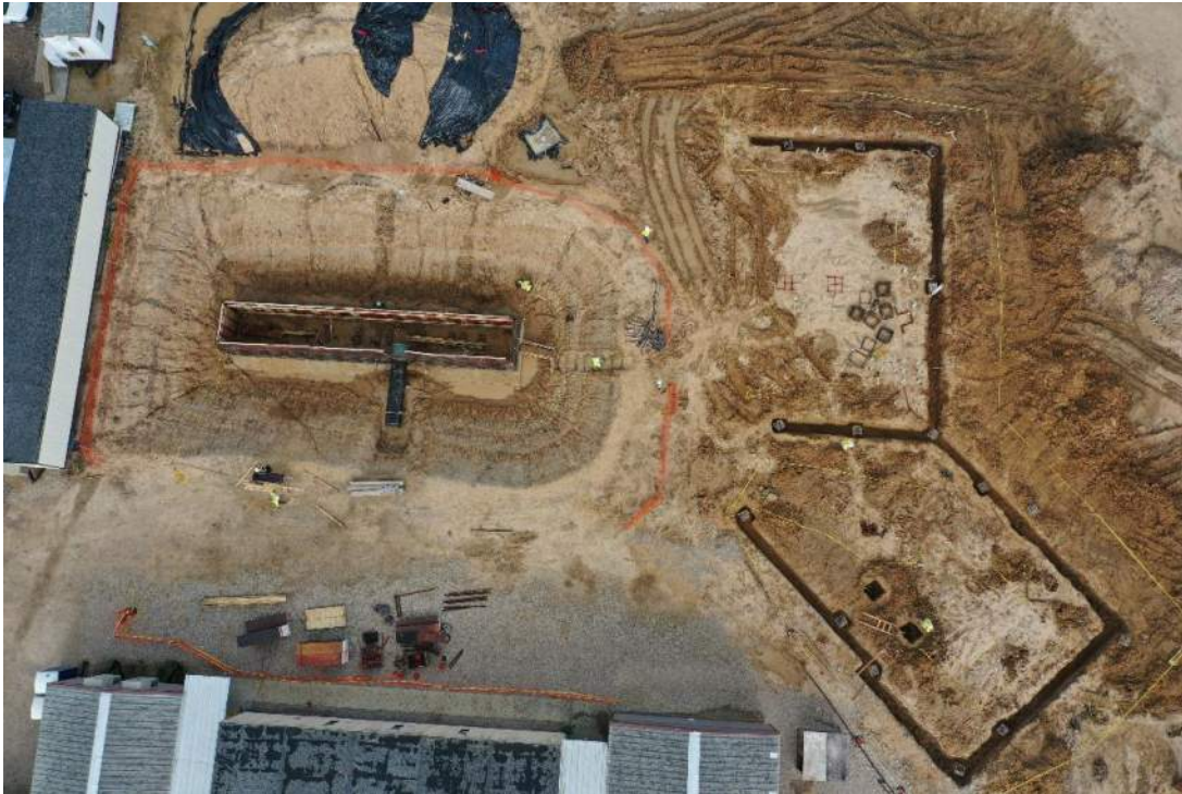
High Service Pump Building Foundation showing Supply Header Pipe Trench
