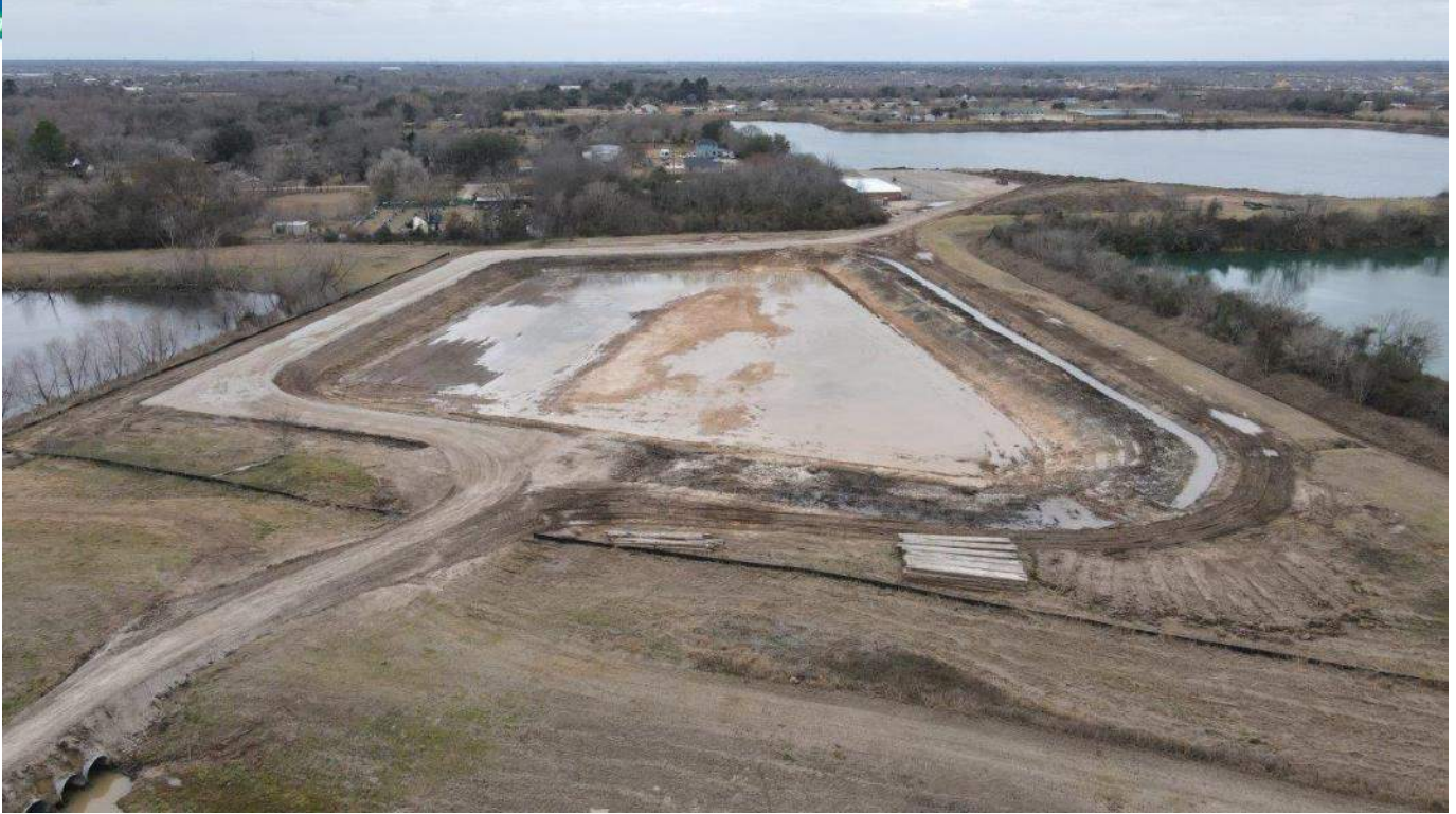
Site Detention Pond
