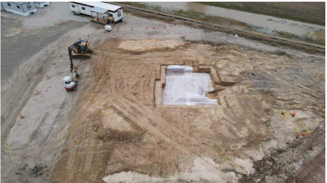
Chlorine & Chlorine Dioxide Building Foundation
