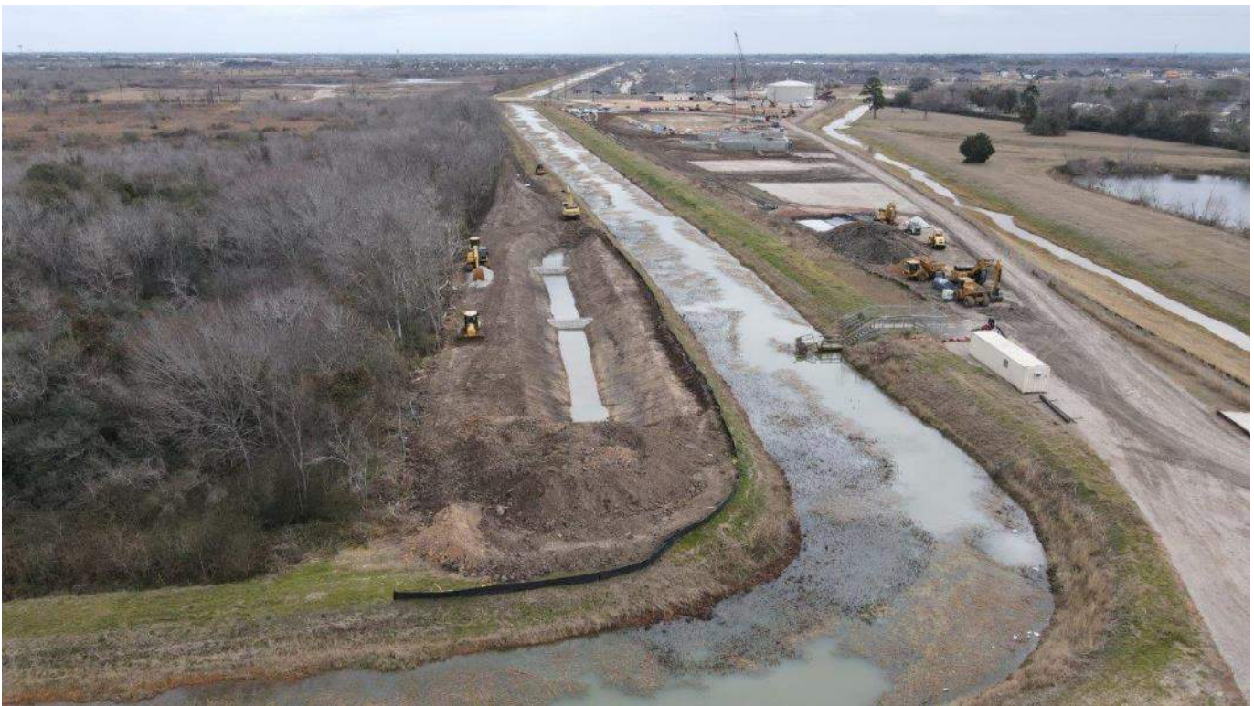
Canal Bi-Pass Channel
