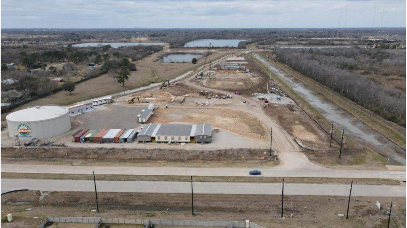
Plant Site Overall View
