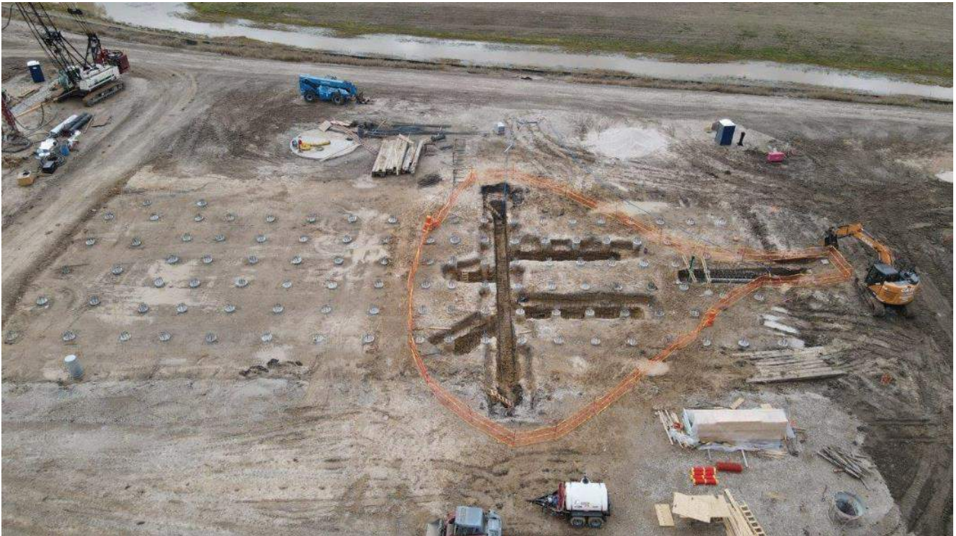
Pre-Treatment Basin Auger Cast Piles and Foundations
